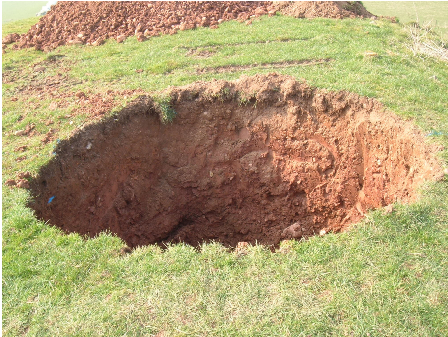
Plate 6: Excavation of Tank 1 (Septic Tank), facing northeast
