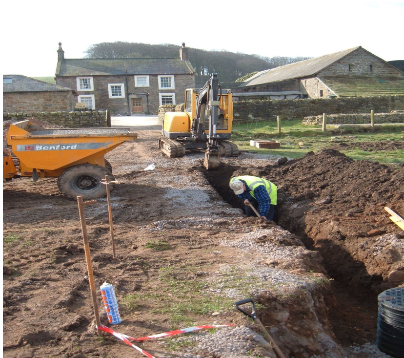
Plate 3: Pipe trench, facing south, Willowford Farmhouse in the background
