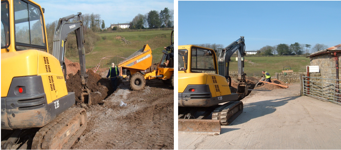
Plate 1 and 2: Excavation of the pipe trench, facing north
