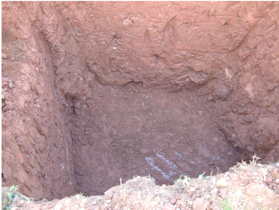
Plate 7: Base of septic tank trench
