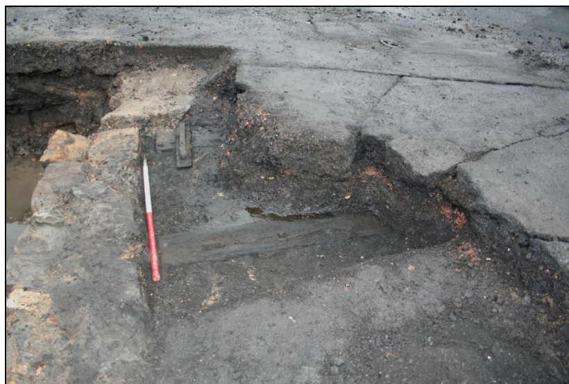
Plate 20: Detail of timber sleepers and iron rail of wagon way in Area C (looking north)
