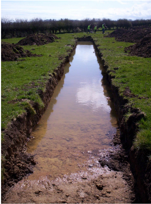
Plate 1. Trench 2, looking south-east showing water drainage issues (southern end of trench is 1.12m deep)
