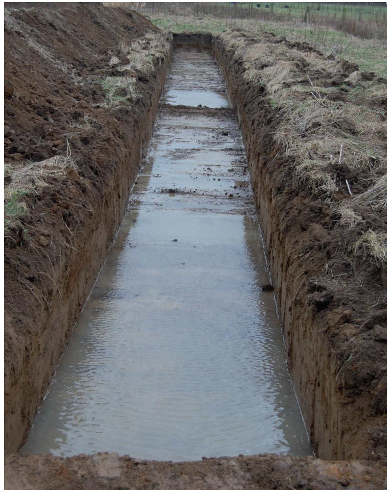
Plate 10: View of Trench 5 Looking Southwest.
