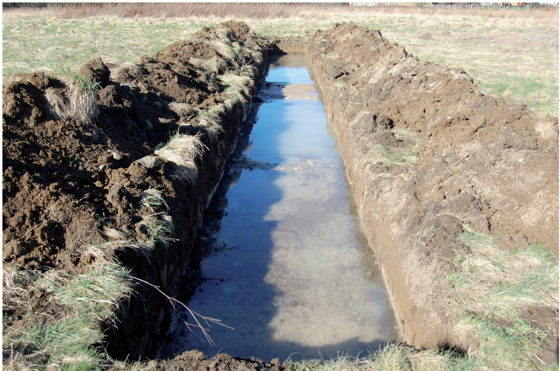
Plate 12: View of Trench 6 Looking Northwest.
