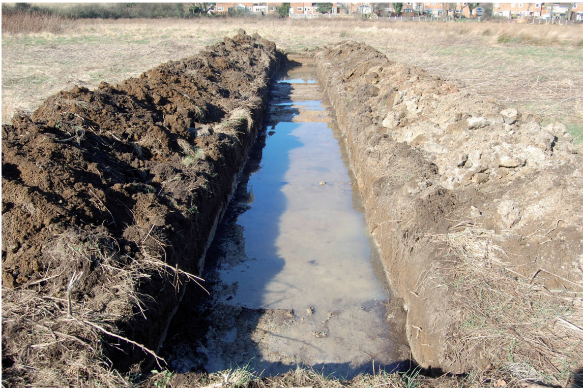
Plate 14: View of Trench 7 Looking Northwest.
