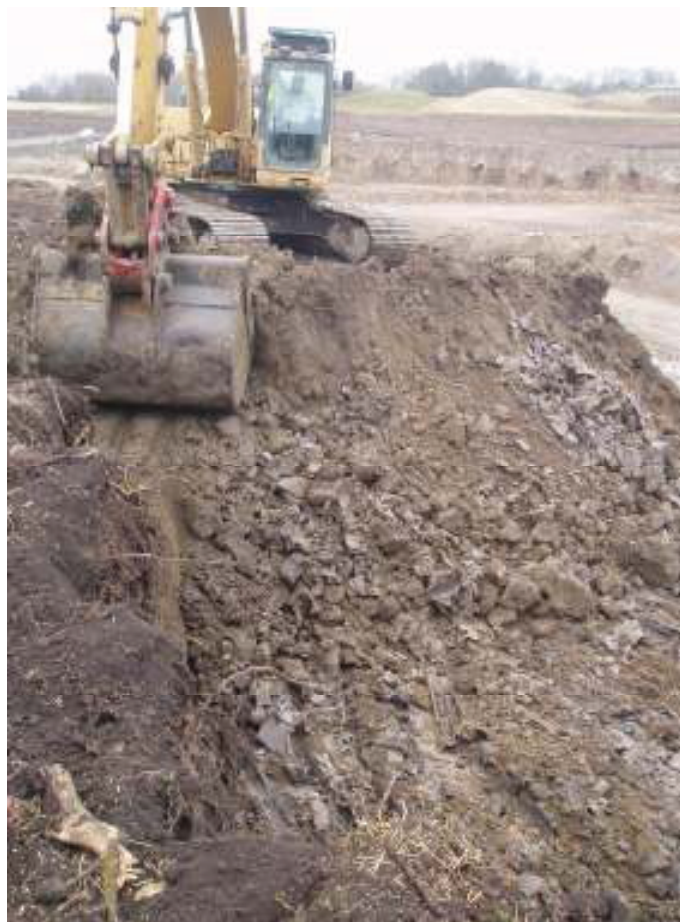
Plate 4: Day 1 excavations looking southeast
