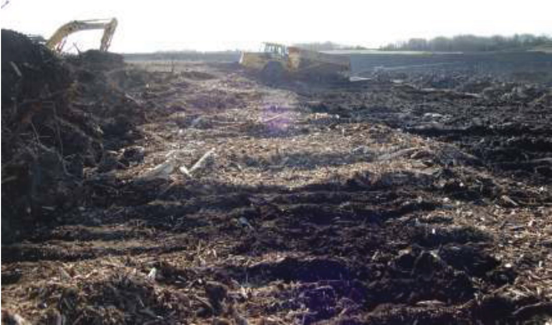
Plate 1 : Day 1 of stripping looking southeast
