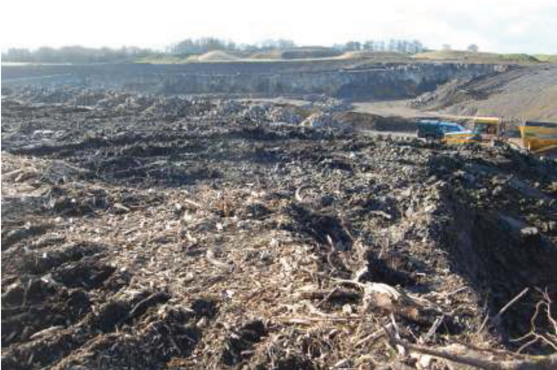
Plate 2: Day 1 of stripping looking south
