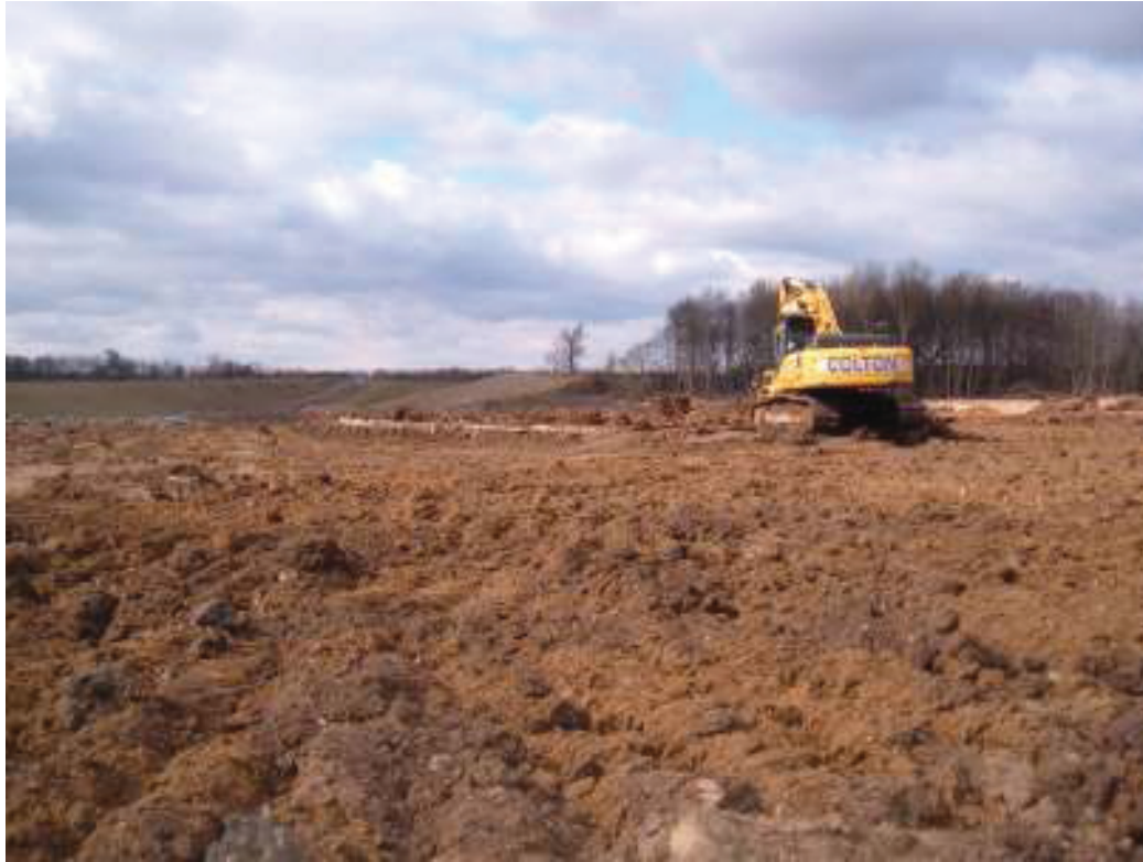
Plate 7 : Day 5 excavations looking northwest
