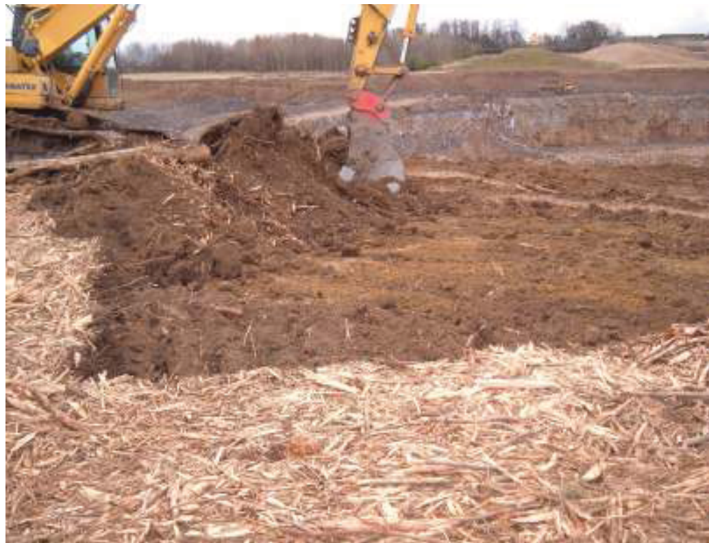
Plate 6 : Day 5 excavations looking south
