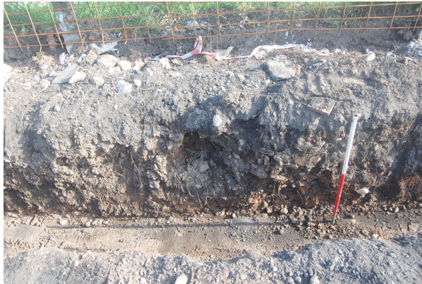
Plate 2: Excavation of the foundation trench, facing north, note demolition rubble.
