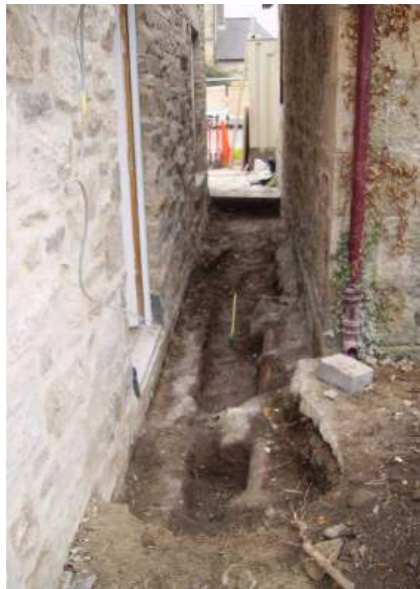
Plate 11: East-west Drain Cut facing west
