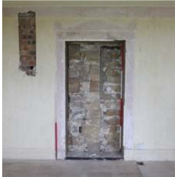
Plate 4: Blocked window in north wall of present drawing room, facing north
