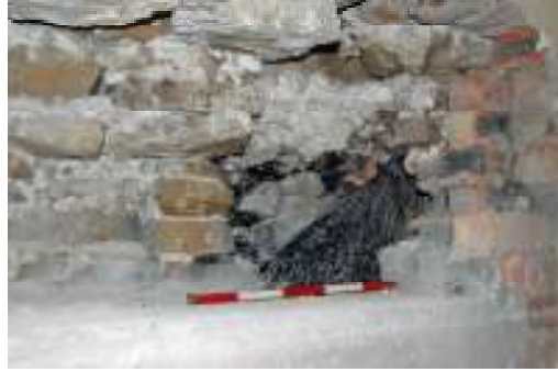
Plate 13: Slate-lined flue
