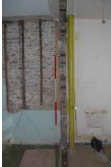
Plate 9: Section of northern hall wall revealed after demolition of Wall 2
