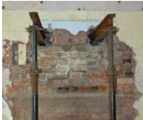
Plate 12: Mixture of brick and rubble revealed above fireplace in kitchen
