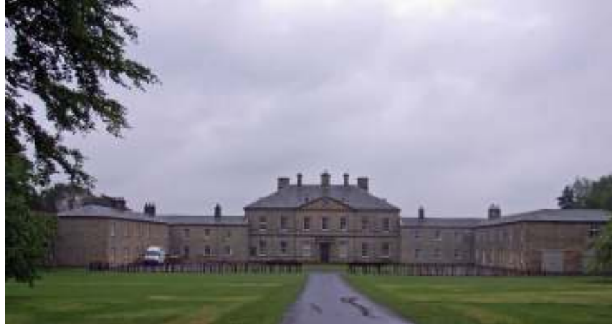
Plate 2: North-facing elevation of Capheaton Hall (eastern wing shown on left)
