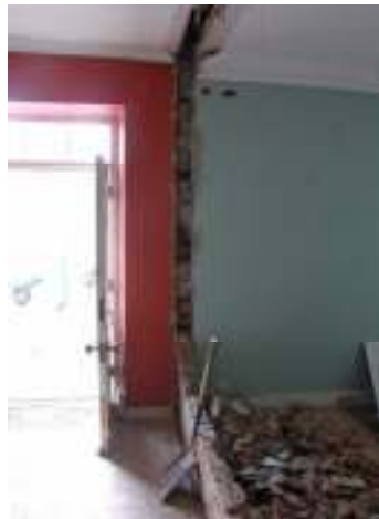
Plate 8: Section of western hall wall revealed after demolition of Wall 1
