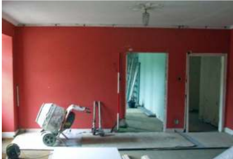
Plate 7: Wall 1 (foreground) and Wall 2 (adjoining, centre) prior to demolition
