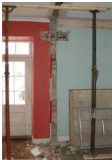
Plate 10: Hole inserted in western hall wall
