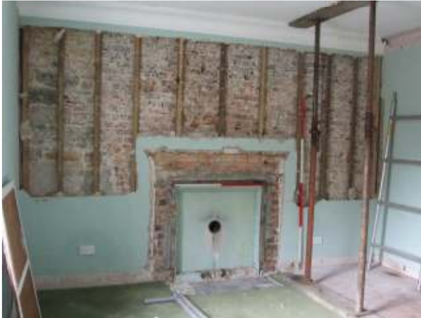
Plate 5: Northern wall of present sitting room, facing north
