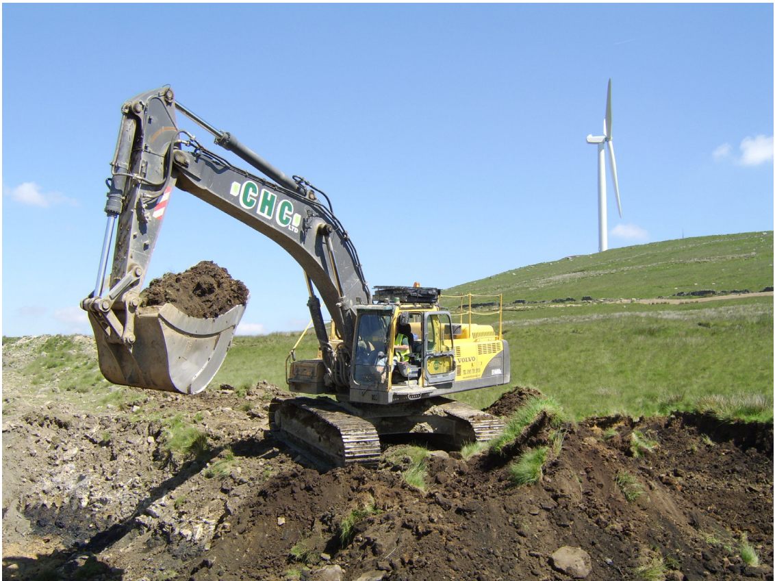
EXCAVATION IN PROGRESS, SCOUT MOOR QUARRY
