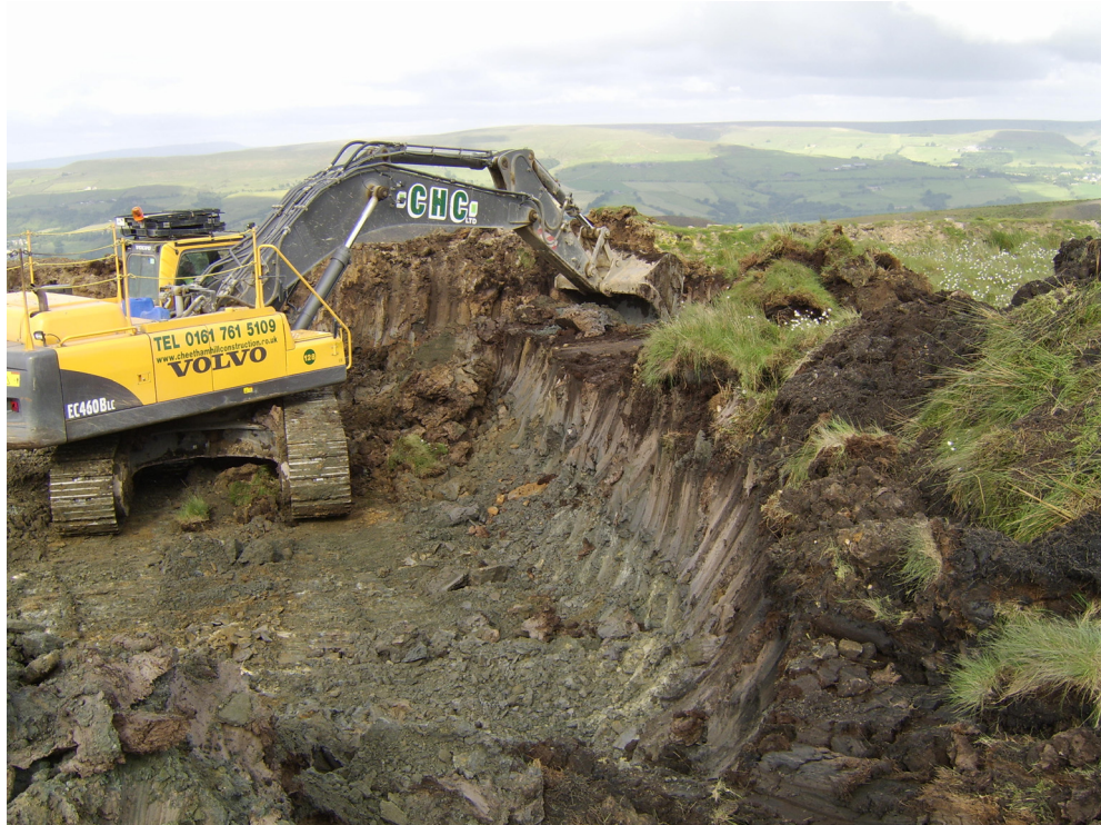
Plate 2: Phase 2 Stripping Operations in Progress, facing West
