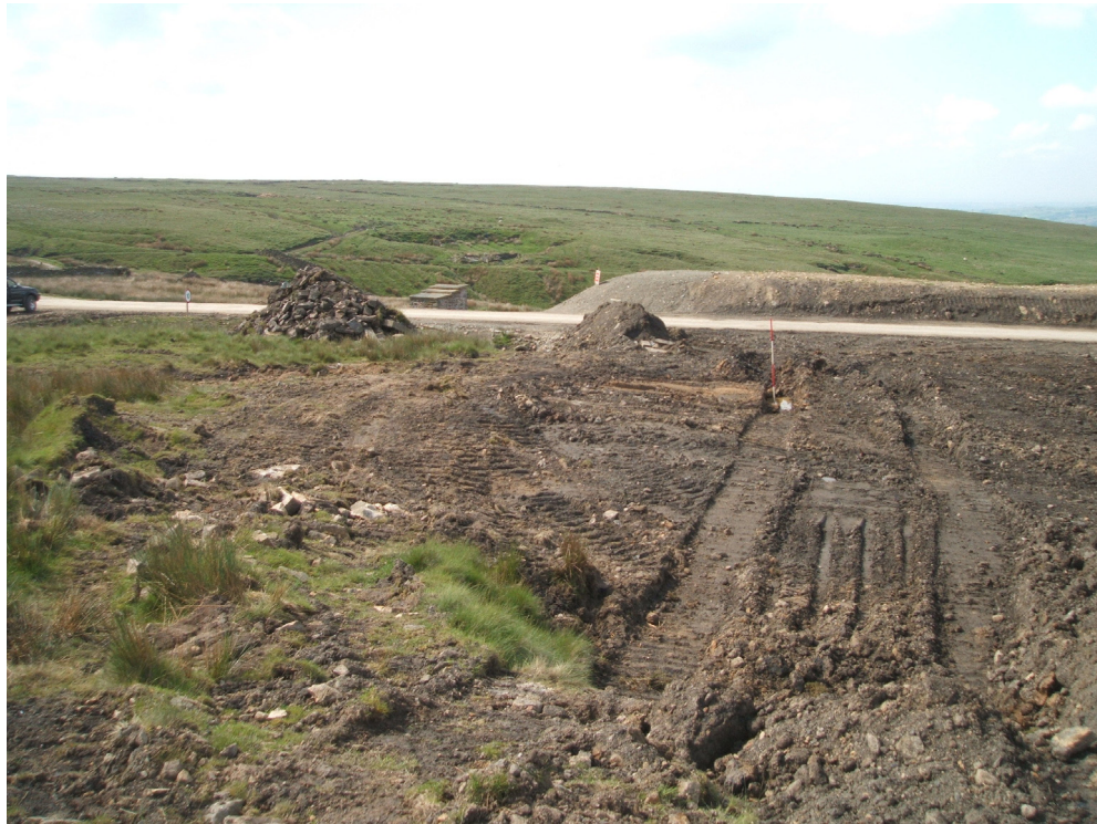
Plate 1: Site of Former Colliery Winding Structure S7, facing South; Ranging-Pole marks Approximate Location of Building
