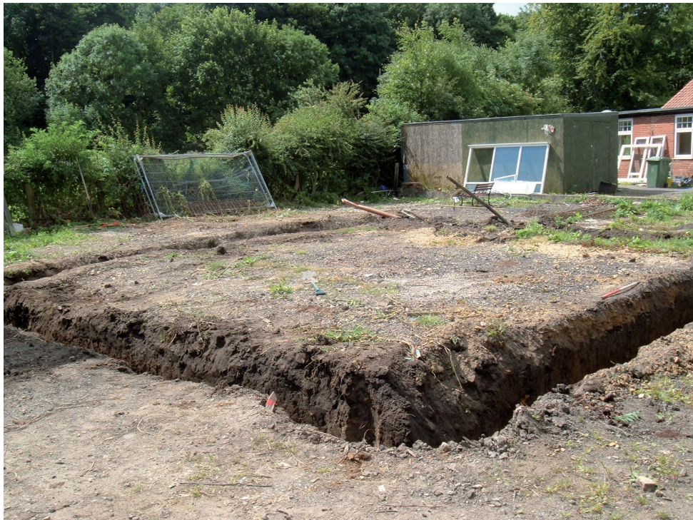
Plate 2: View of completed works taken looking southwest.
