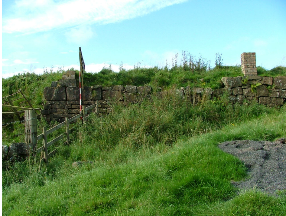
Plate 13 – One remaining brick pier along the top of the retaining wall which presumably relates to the more recent use of the kiln as a safety fence (Scale = 2m)
