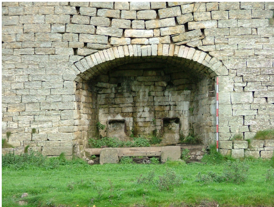
Plate 5 – Right-hand draw arch showing the two draw eye and modern concrete blocks in the foreground (Scale = 2m)
