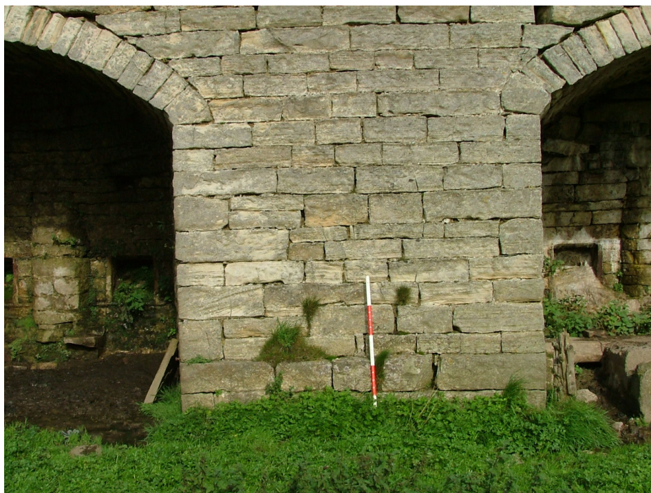
Plate 3 – Section between the two draw arches showing plinth at base of elevation (Scale = 1m)
