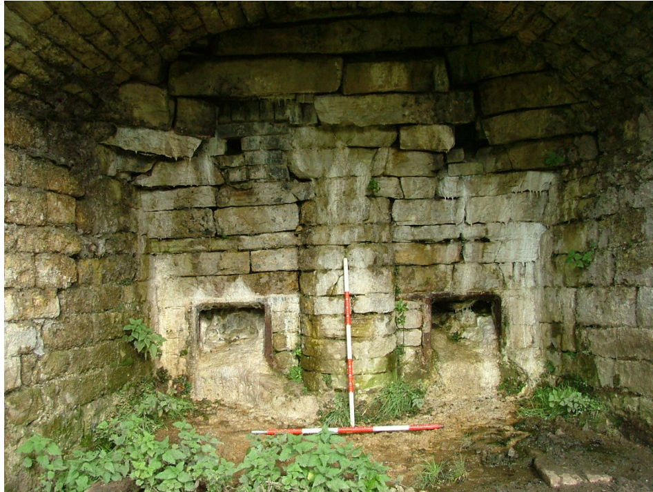
Plate 6 – Detail of the two draw eyes with iron frames, the semi-circular support for the pot and the remains of the most recent lime burning (Scales = 1m each)
