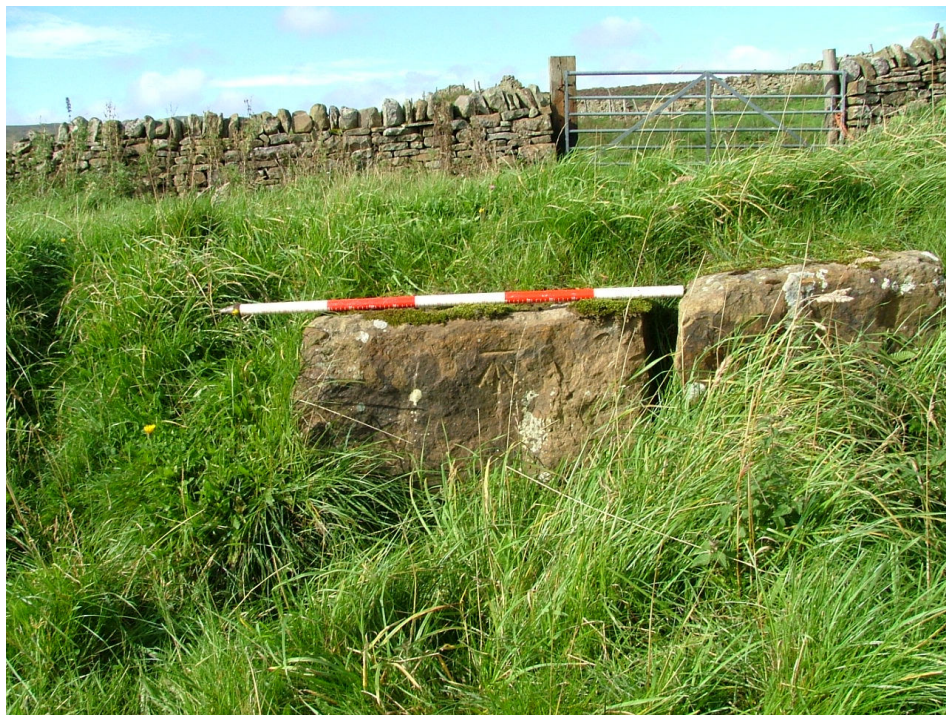
Plate 14 – Bench mark on one of the masonry blocks which make up the retaining wall of the loading ramp (Scale = 1m)
