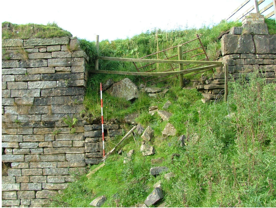
Plate 11 – Vertical construction break between the kiln (left of photograph) and remains of retaining wall (Scale = 2m)
