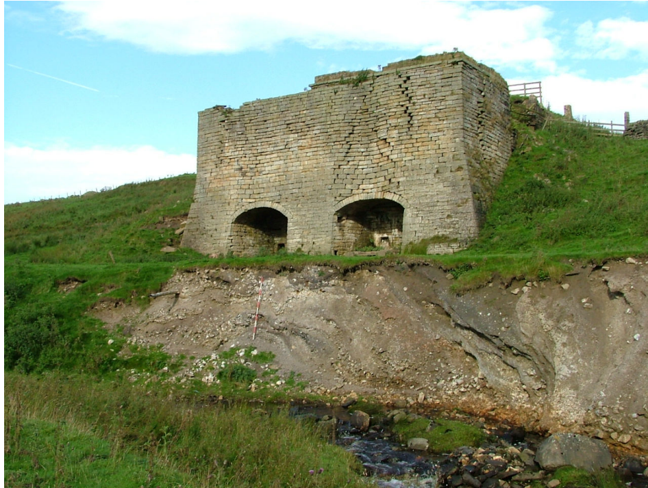
Plate 18 – View looking north-west from the south side of Middlehope Burn showing the stratigraphy of waste material from working of the kiln (Scale = 2m)
