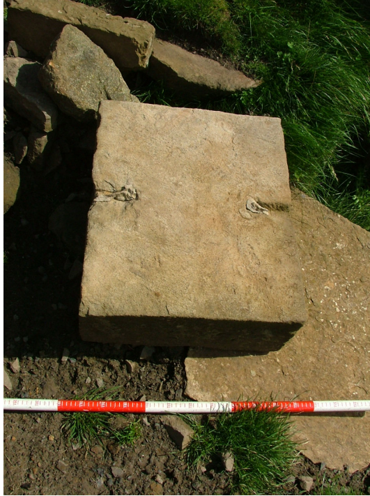
Plate 9 – Dislodged sandstone block with the remains of lead set in grooves either side (Each red and white section of scale measures 20cm)
