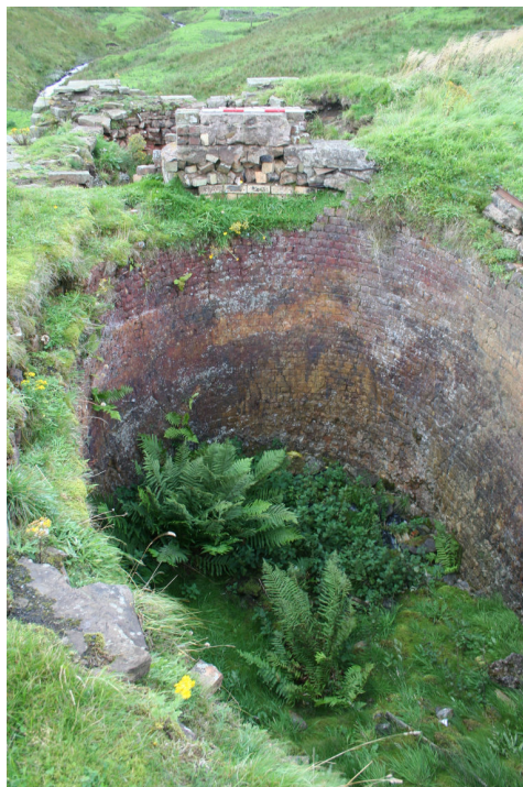
Plate 16 – View looking south-west of eastern pot showing the brick lining (Scale = 1m)
