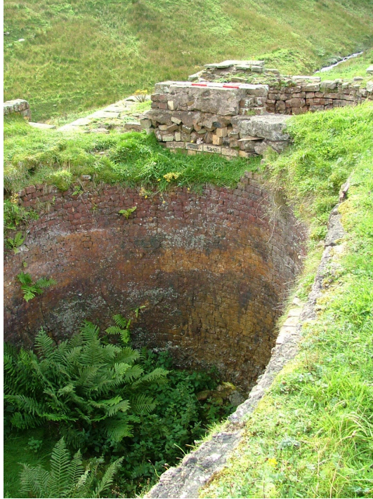
Plate 15 – View facing south-west showing the two pots in the top of the kiln. Note the brick-lining of the pot in the foreground and the remains of a modern brick and concrete wall between the two (Scale = 1m)
