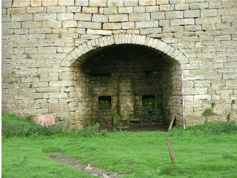
Plate 4 – Left-hand draw arch which protects the two draw eyes (Scale = 2m)
