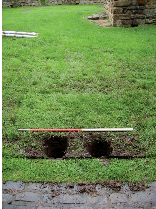
Plate 10: foundation cuts for Interpretation Panel No. 4, facing south.
