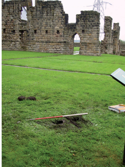
Plate 5: foundation cuts for Interpretation Panel No. 2, facing north east.
