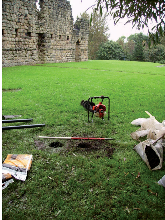
Plate 2: foundation cuts for Interpretation Panel No. 1, facing south east.
