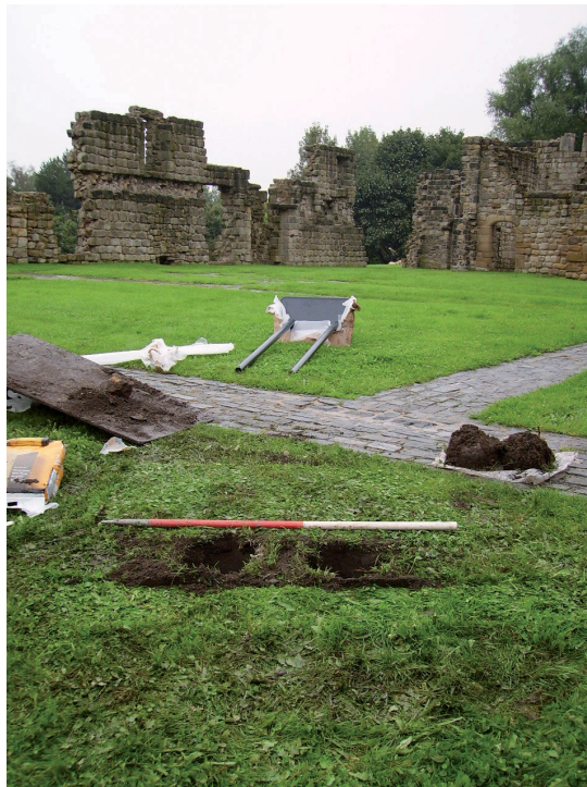
Plate 16: foundation cuts for Interpretation Panel No. 6, facing west.
