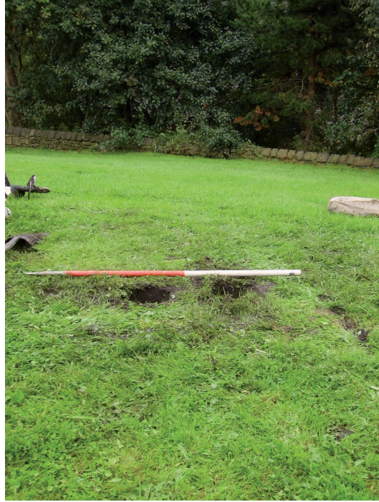
Plate 8: foundation cuts for Interpretation Panel No. 3, facing south east.
