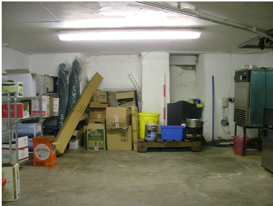
Plate 21 – North-east wall of cellar, note the two niches (Scale = 1m)
