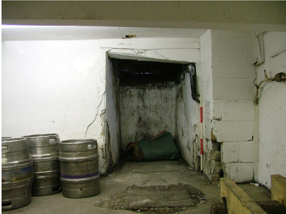
Plate 22 – Barrel drop, southern end of north-east cellar wall (Scale = 1m)
