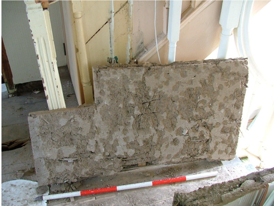
Plate 58 – The removed wattle and daub panel, the corner was removed to allow for analysis of construction method (Scale = 1m)
