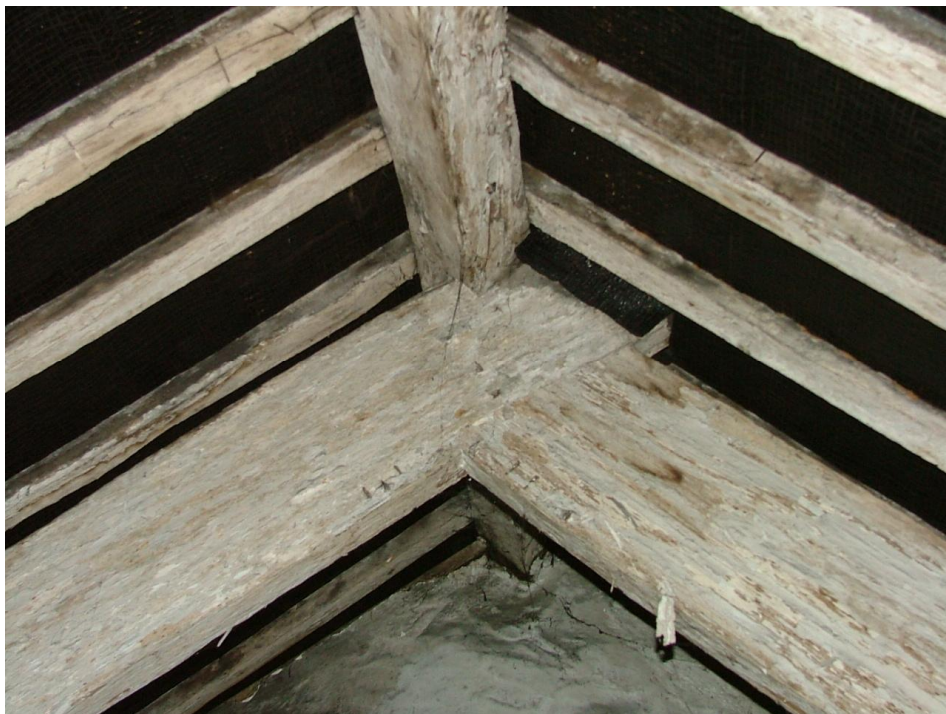
Plate 43 – Southernmost roof truss showing assembly marks IIIø
