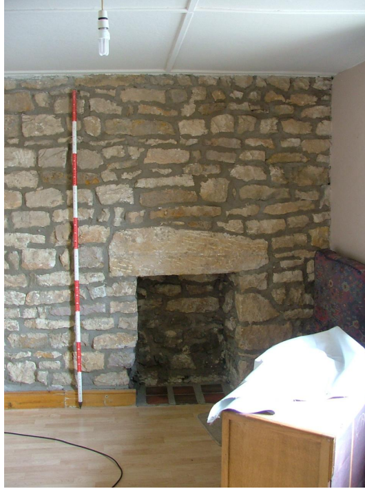
Plate 32 – Fireplace in Bedroom 2, second floor. The panelled ceiling is a modern insertion (Scale = 2m)
