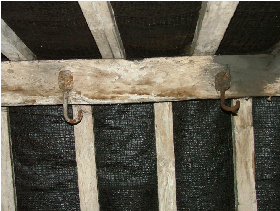
Plate 45 – Two iron hooks fixed to the ridge beam in the attic
