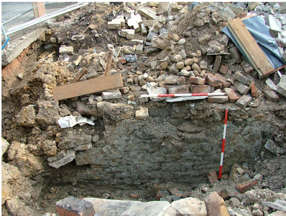
Plate 48 – View looking north-east showing masonry wall revealed to the rear of the Wagon and Horses (Scales = 1m)
