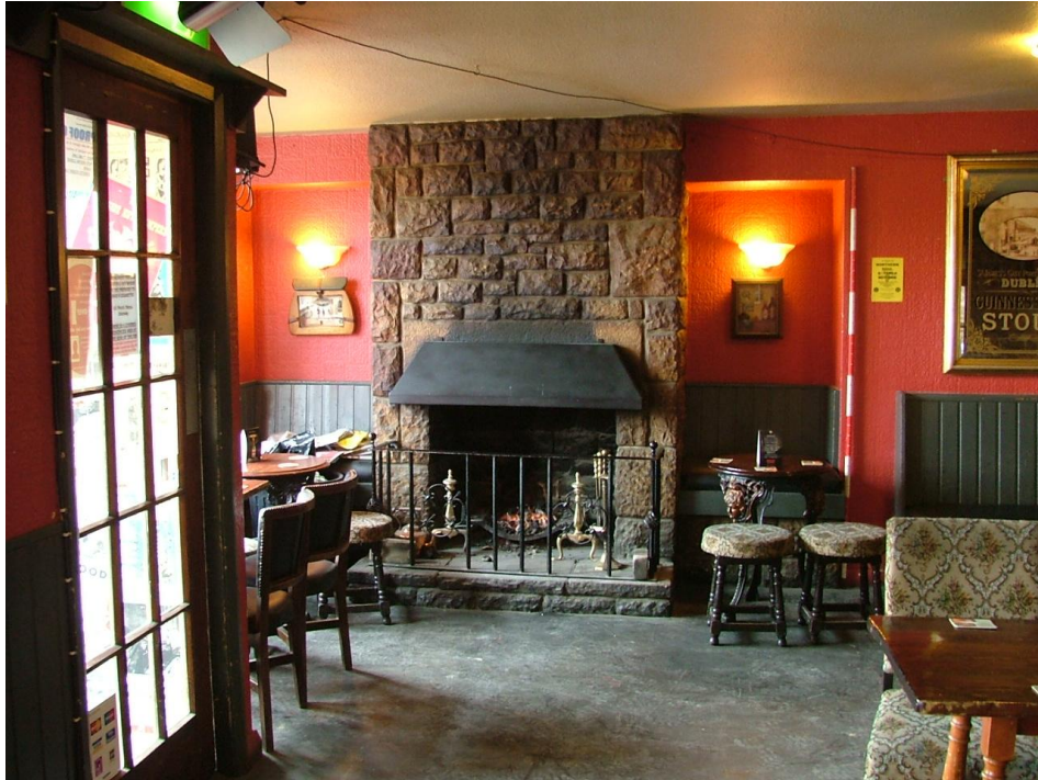
Plate 18 – South-east internal wall of Wagon and Horses showing two of the three recesses set in this wall, possibly original but perhaps inserted to provide an 'inglenook' feel to the pub (Scale = 2m)
