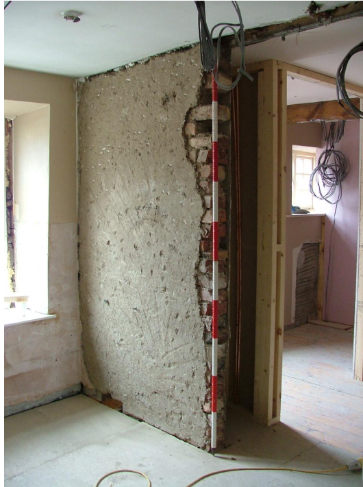
Plate 65 – Layer of plaster consisting of mud and straw, former bathroom wall, second floor (Scale = 2m)
