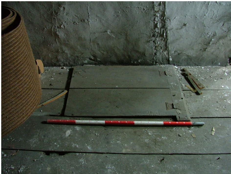
Plate 39 – Wooden hatch in attic floor, note the butterfly hinges (Scale = 1m)
