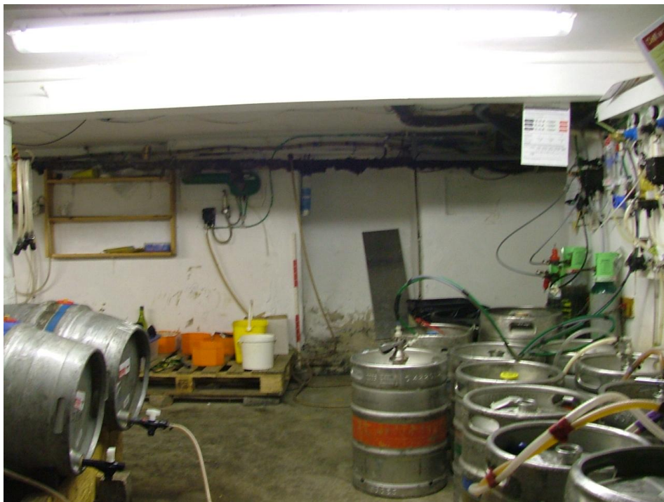
Plate 25 – Recess in south-west wall of cold cellar (Scale = 1m)
