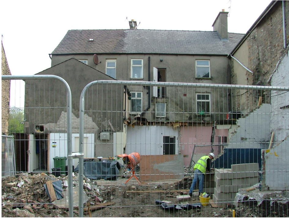
Plate 49 – View looking north-east of the rear of the Wagon and Horses after the removal of the garage/workshop and the single-storey extension
