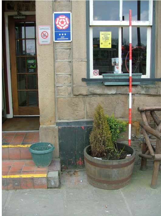
Plate 13 – Small door in north-east elevation (Scale = 2m)
