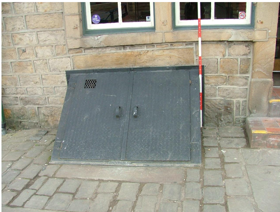
Plate 12 – Barrel-drop, north-east elevation (Scale is in 20cm graduations)
