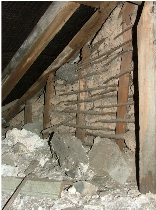
Plate 37 – Detail of the wattle and daub of one of the cross-walls in the attic
