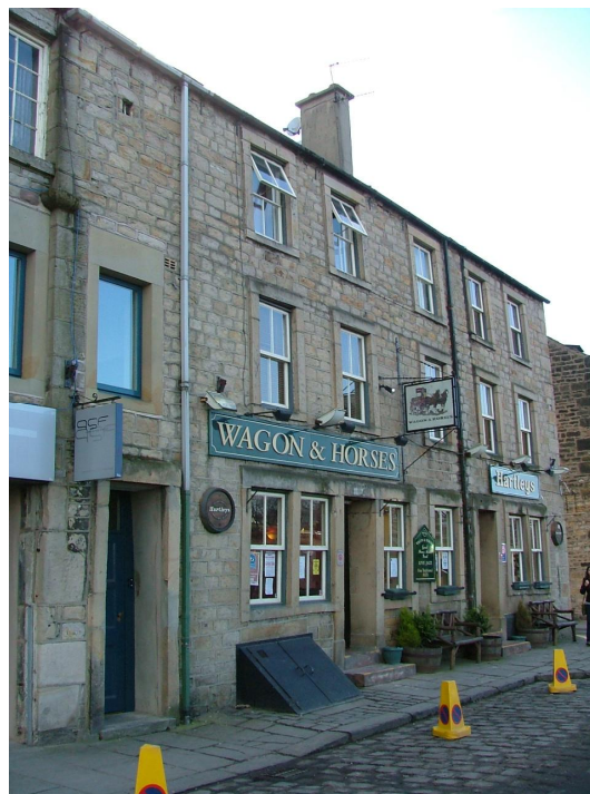
Plate 8 – View of north-east elevation facing St George's Quay, the doorway to left of photograph does not provide access into any part of the Wagon and Horses; however it clearly formed part of the original building as shown by the stonework
