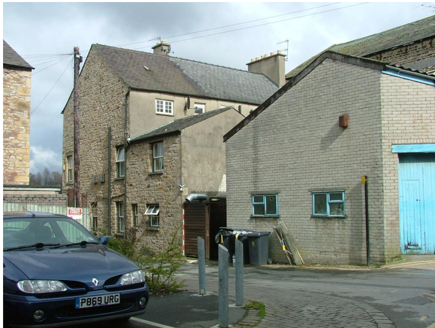
Plate 15 – View looking east of the north-west and south-west elevations. The garage/workshop to right of photograph was demolished as part of the renovation work (Scale = 2m)
