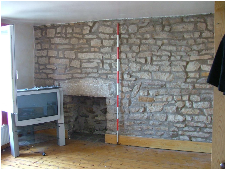
Plate 31 – Fireplace in Bedroom 1, second floor (Scale = 2m)
