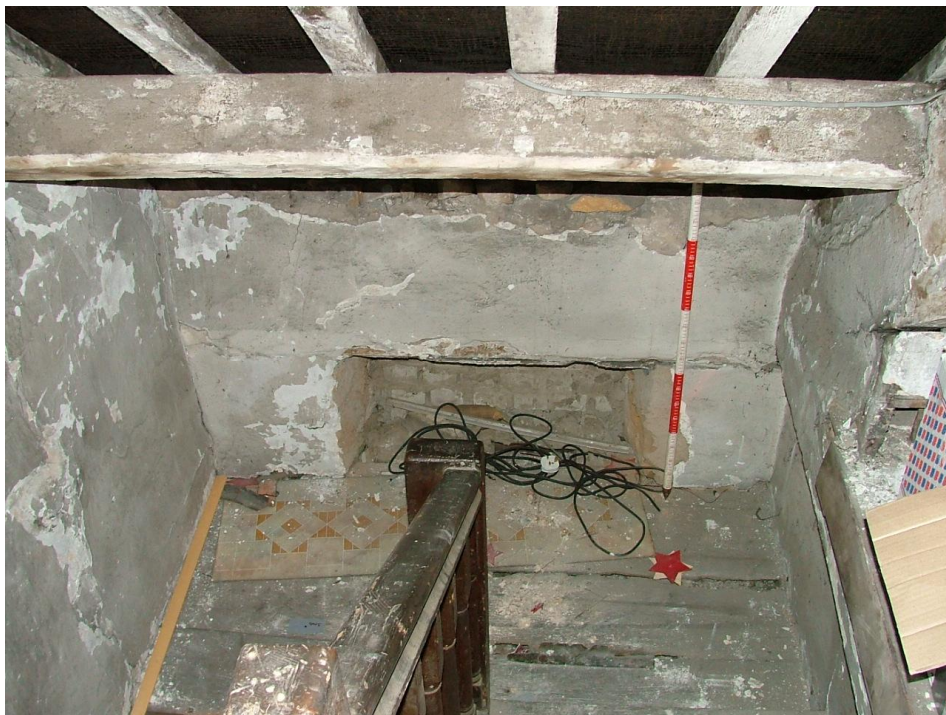
Plate 35 – Blocked aperture, landing to attic (Scale = 1m)
