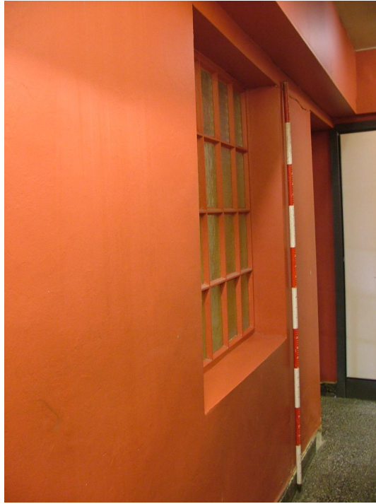
Plate 20 – View from corridor in extension of 20-pane window located in original back wall of No.27 St George's Quay (Scale = 2m)
