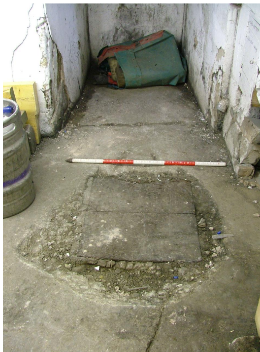
Plate 23 – Wooden cover over ? well or possibly relating to some form of flood alleviation (Scale = 1m)
