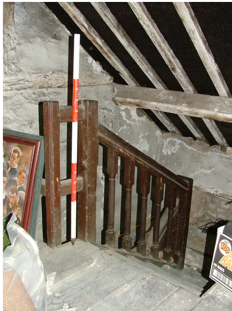
Plate 33 – Detail of 18 th century staircase as seen from the attic (Scale = 1m)
