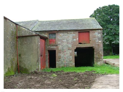
**Plate 57** – North elevation of Building F. Note the difference in roof level suggesting different construction phase (Scale = 2m)
