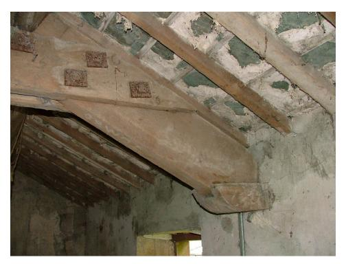
Plate 79 – Detail of the end of the roof truss, first floor, Building F
