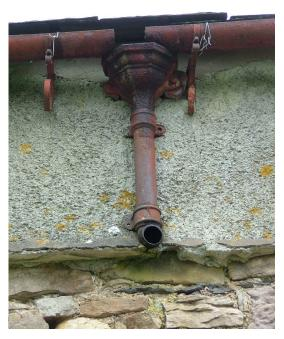
**Plate 55** – Downpipe remains *in-situ* which formerly discharged onto the roof of the now demolished cattle shed, south elevation of Barn D, Range C
