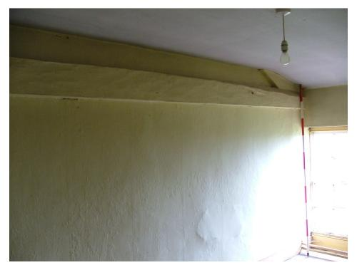
Plate 17 – Base of a roof truss visible in the wall between the box room and the bathroom. Note the slope of the ceiling at the edge over the window, as is also the case in the bathroom
