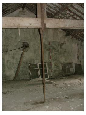
Plate 78 – Iron rod supporting the roof truss, first floor, Building F (Scale = 2m)
