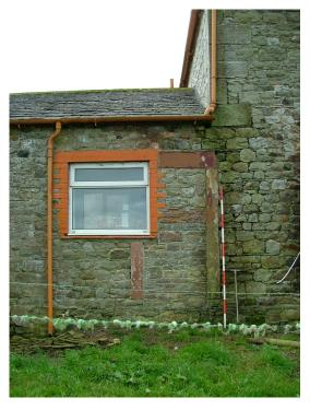
Plate 27 – Surround of former doorway, north end of north-east elevation of Range A. Note the quoins of the single-pile extension which stop at the top of the wall for Range A suggesting they may be contemporary (Scale = 2m)
