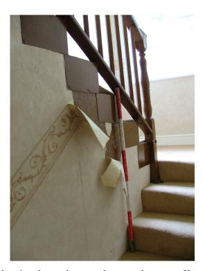
Plate 11 – Staircase, showing decorative newel post and veneer-effect covering (Scale = 1m)
