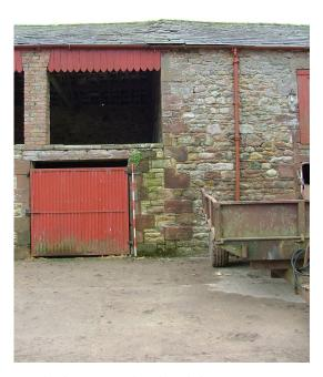
Plate 47 – Evidence for vertical construction break between Barns C and D, north elevation, Range C (Scale = 2m)
