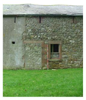
Plate 33 – Blocked doorway and window, north-west elevation of Range B (Scale = 2m)
