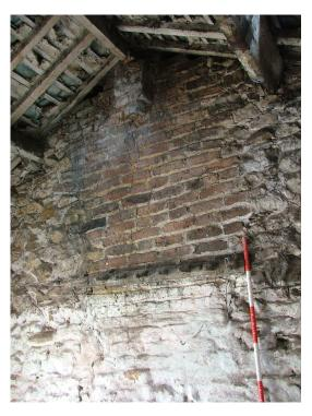
Plate 21 – Internal wall which divides one of the storage rooms and the utility room in Range A showing brickwork and wooden hooks (Scale is in 20cm graduations)
