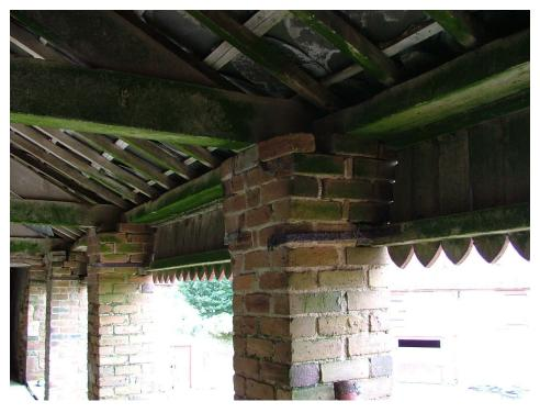
Plate 69 – Detail of the tops of the brick piers and the woodwork, first floor hay barn, Barn C
