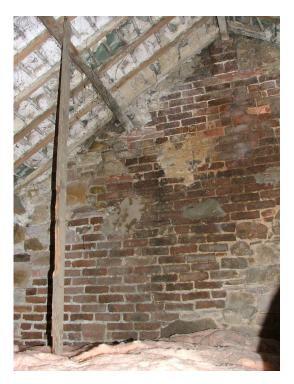
Plate 19 – North-east gable of double-pile house showing brickwork in the masonry
