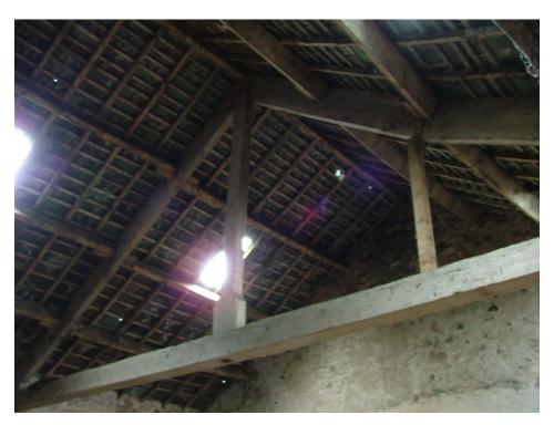
Plate 38 – Roof truss with king post, first floor of Range B
