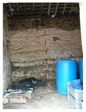
Plate 22 – Interior of store in Range A showing sandstone flag floor, limewashed walls and ventilation slit above the scale (Scale = 2m)
