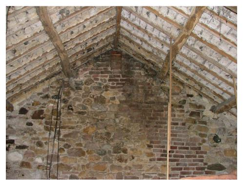
Plate 18 – South-west gable end of double-pile house showing brickwork in the earlier masonry, possibly filling the gap of a removed or repaired chimney flue. Note the two rows of hand-cut purlins either side of the roof
