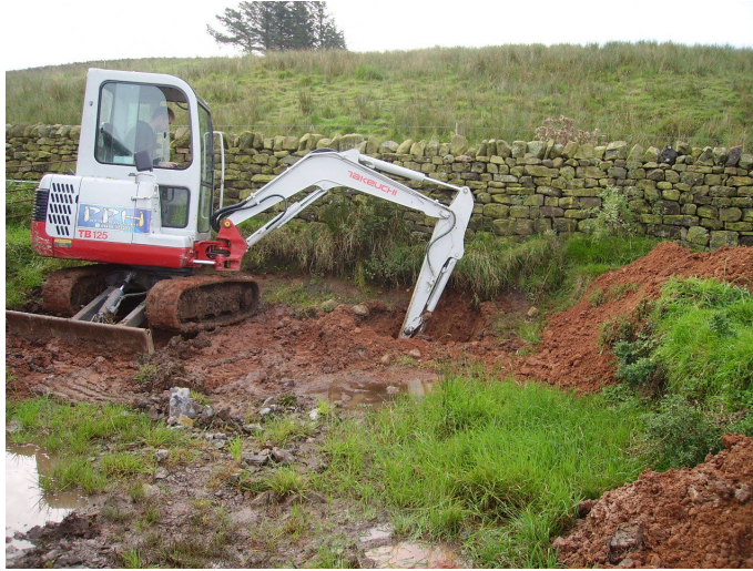
Plate 1: Foundation Pit No. 1 under excavation, facing south
