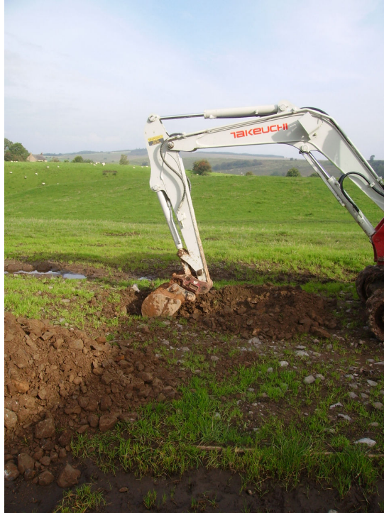
Plate 9: Foundation Pit No. 5 under excavation, facing north.
