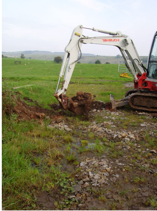
Plate 5: Foundation Pit No. 3 under excavation, facing north.
