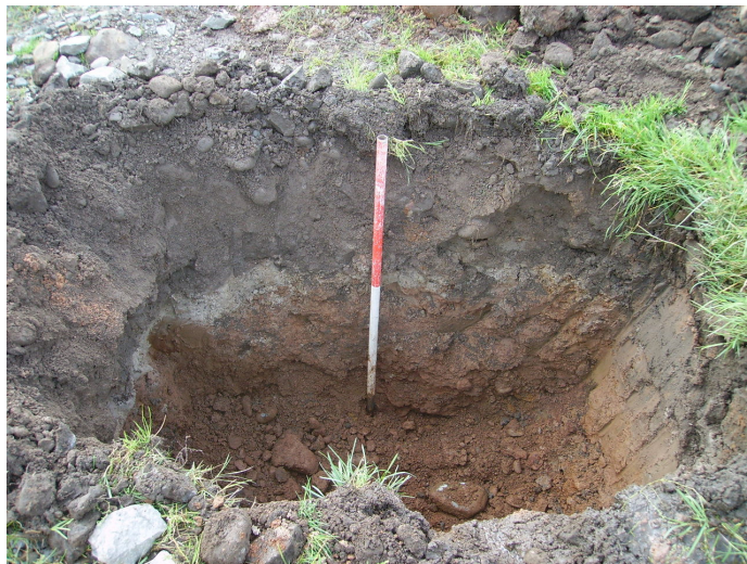
Plate 6: Section of Foundation Pit No. 3, facing south.
