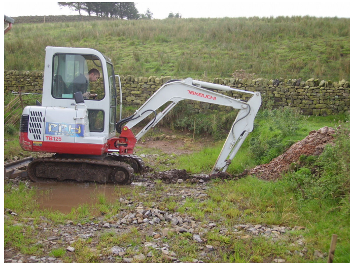
Plate 3: Foundation Pit No. 2 under excavation, facing south.
