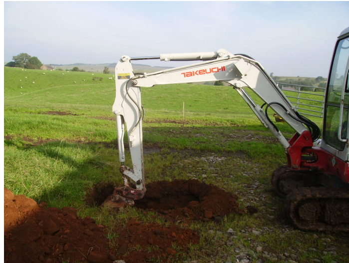
Plate 7: Foundation Pit No. 4 under excavation, facing north.
