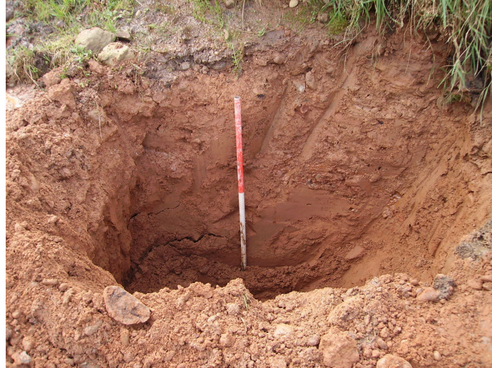
Plate 2: Section of Foundation Pit No. 1, facing south.
