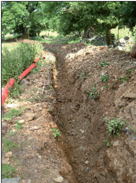
Plate 5 – View north towards northern end of monitored section of service trench
