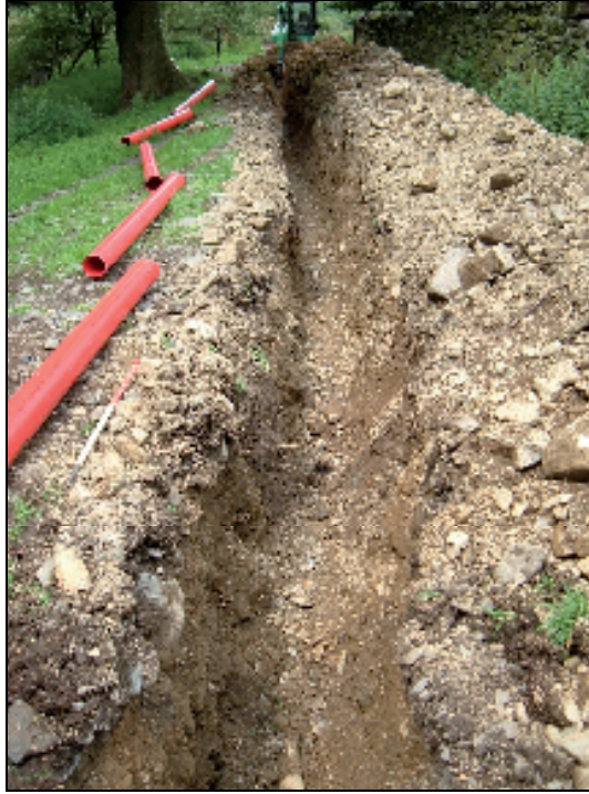
Plate 4 – View north of southern section of service trench
