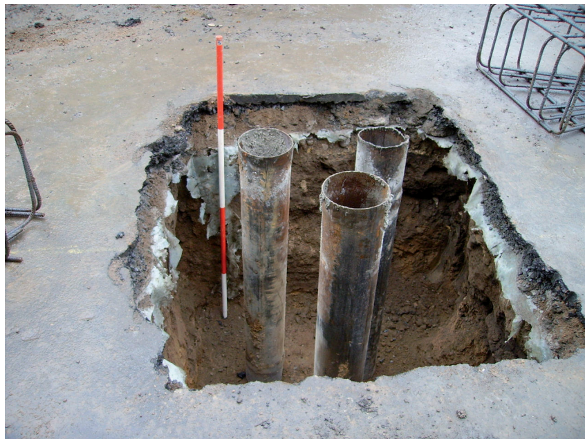
Plate 5. Support Pile 'b' excavation, looking west.
