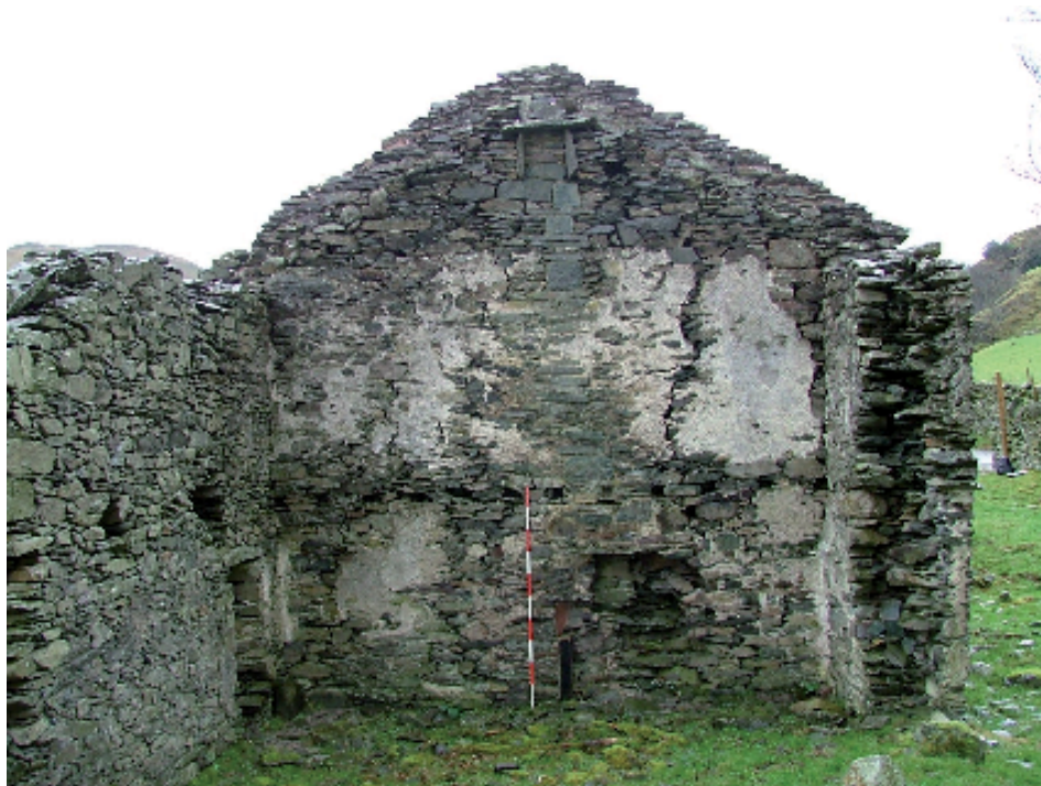
Plate 10 – View looking south of the south gable of house showing remains of fireplace at ground level, joist holes for former first floor, areas of mortared wall and support for the chimney at apex of gable (Scale = 2m)
