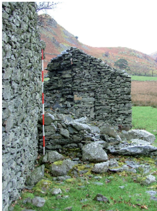
Plate 8 – View looking north showing the possible remains of a semi-circular outshut to rear (east) side to house staircase (Scale = 2m)
