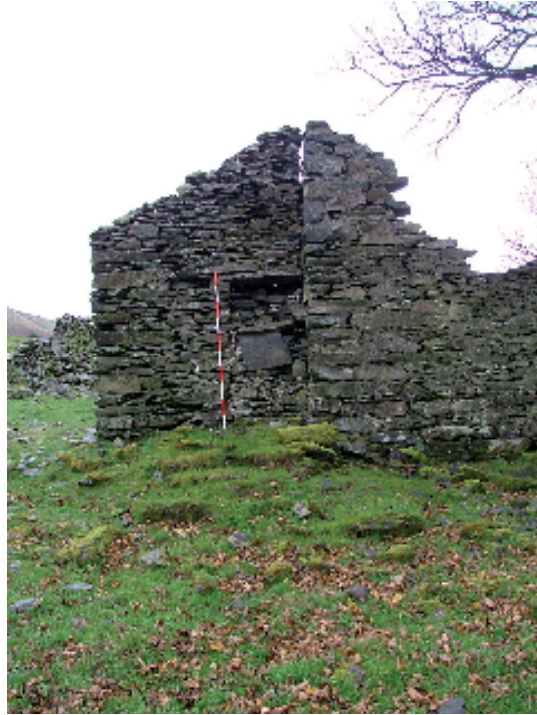
Plate 15 – View looking south showing the vertical line of a construction break between main house and outshut which contains a blocked doorway (Scale = 2m)
