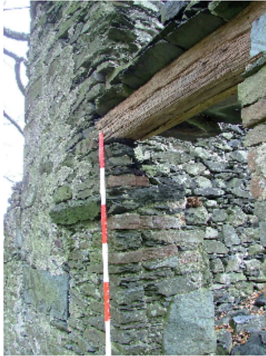
Plate 13 – View of doorway at north end of west wall showing extant wooden lintel, and rebated jambs constructed from a mix of slate and red sandstone. Note the slates over the lintel which kept rainwater from the doorway
