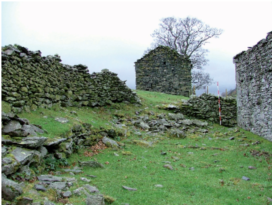
Plate 16 – View looking south down east side of house showing drystone wall and 'ledge', with north gable of the barn in background (Scale = 2m)
