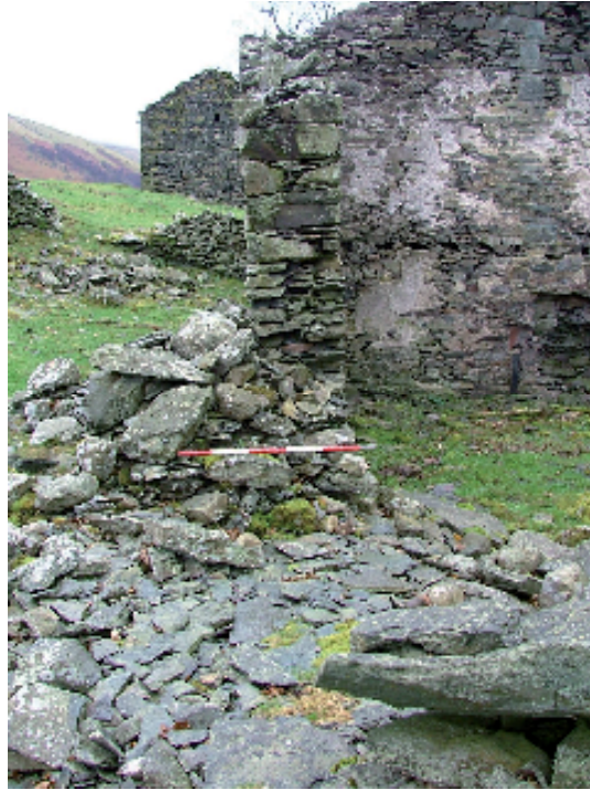
Plate 9 – View looking south showing possible location of former staircase and detail of drystone wall construction (Scale = 1m)
