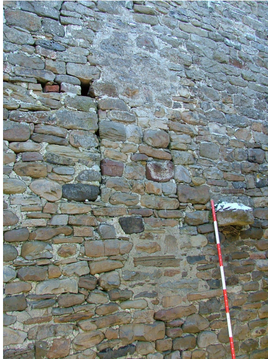
Plate 34 – Blocked window and single through-stone, west elevation of byre
