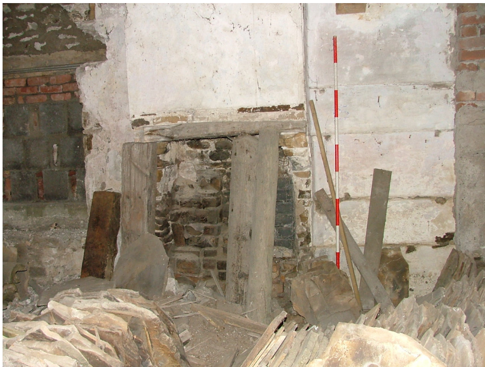
Plate 16 – Fireplace, blocked window and scarring of former shelving, ground floor of former cottage (Scale = 2m)
