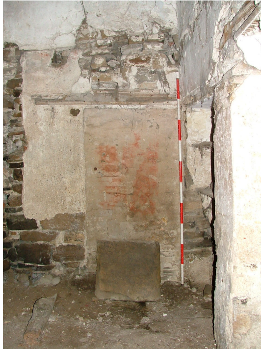
Plate 21 – Blocked doorway in west elevation of former cottage (Scale = 2m)
