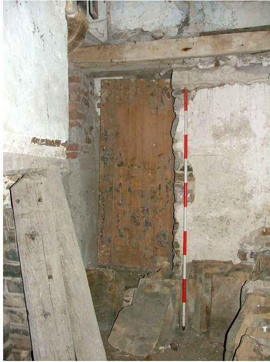
Plate 17 – Inserted doorway, south wall of former cottage (Scale = 2m)
