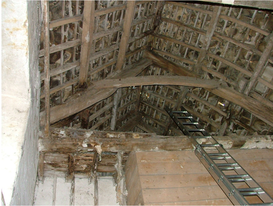
Plate 27 – View from the ground floor of one of the three roof trusses with horizontal collar
