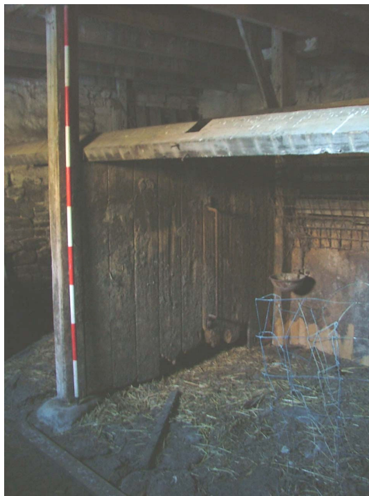
Plate 37 – Detail of one of the stall divisions in the byre (Scale = 2m)
