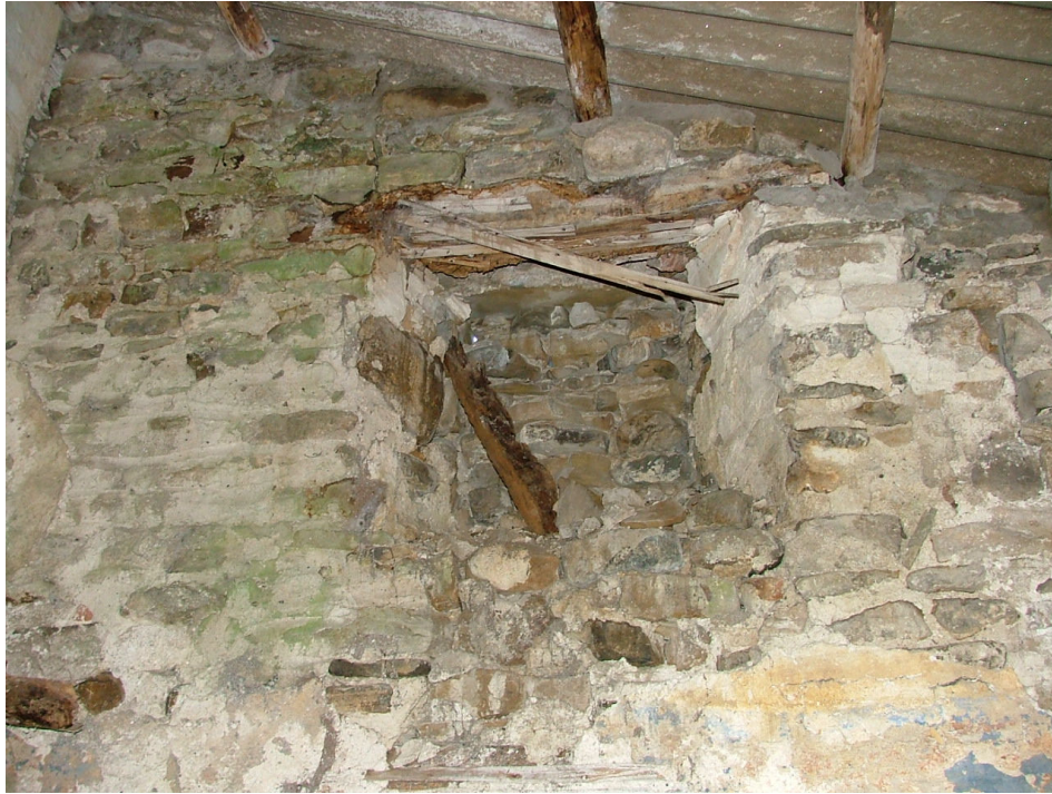
Plate 13 – Internal view of small window in west elevation of extension
