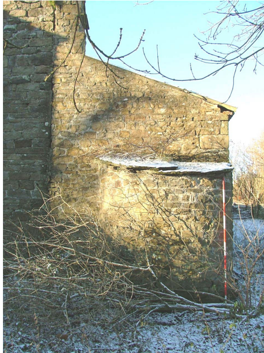
Plate 5 – East elevation of single-storey extension showing semi-circular bread oven (Scale = 2m)
