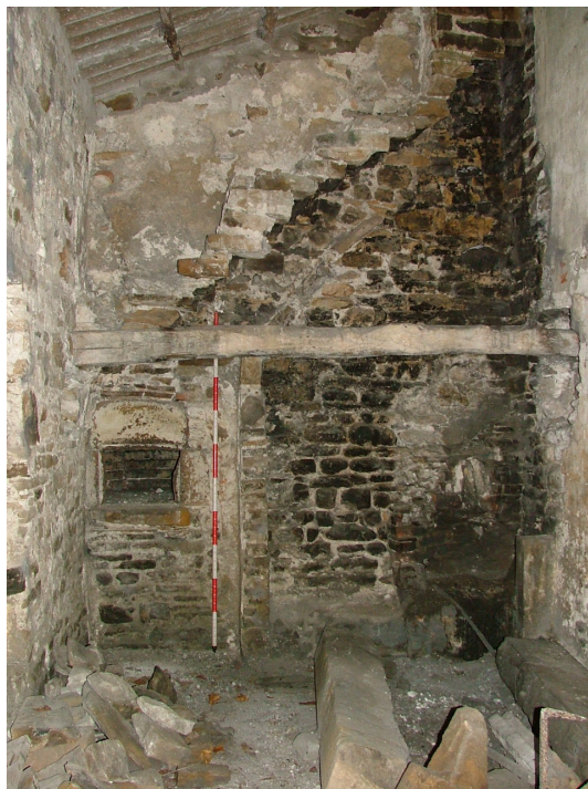
Plate 10 – East interior elevation of single-storey extension showing hole for bread over and the remains of a fireplace (Scale = 2m)
