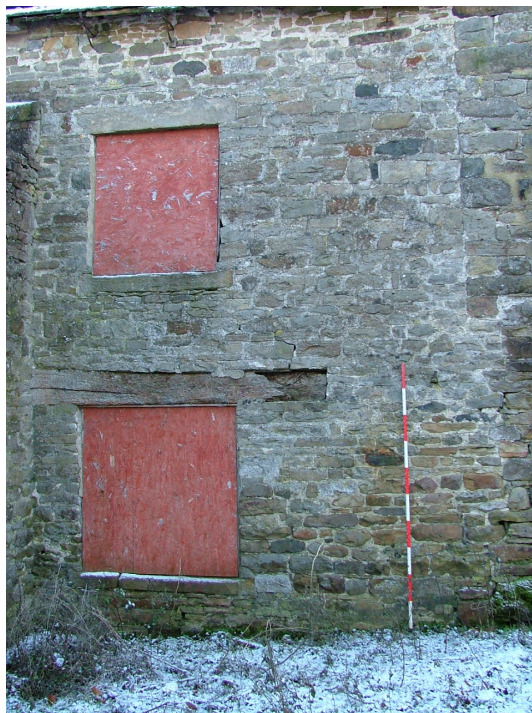
Plate 2 – North elevation of cottage showing windows and vertical construction break between the cottage and the byre (Scale = 2m)
