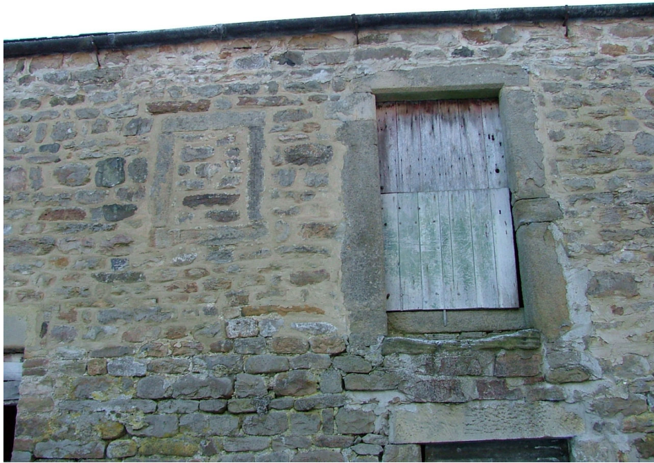
Plate 32 – Detail of first floor doorway and blocked window, north elevation of byre
