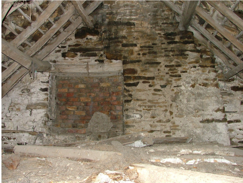
Plate 29 – Blocked window and chimney flue in east wall of former cottage
