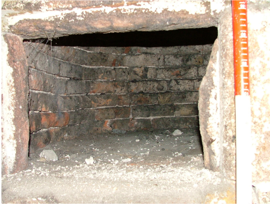
Plate 11 – Interior of bread oven showing brick lining
