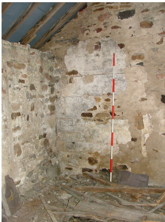
Plate 40 – Horizontal lines of former shelves, first floor of byre (Scale = 2m)
