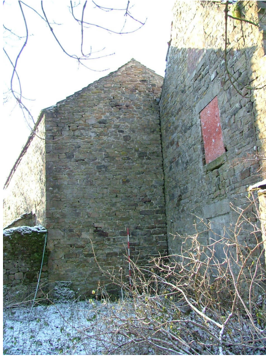
Plate 7 – View looking south showing the farm building constructed against the former cottage (Scale = 2m)
