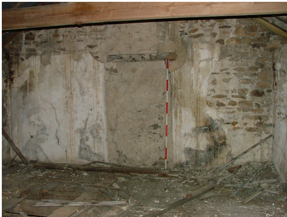
Plate 39 – Former window or doorway, first floor, east elevation of byre (Scale = 2m)
