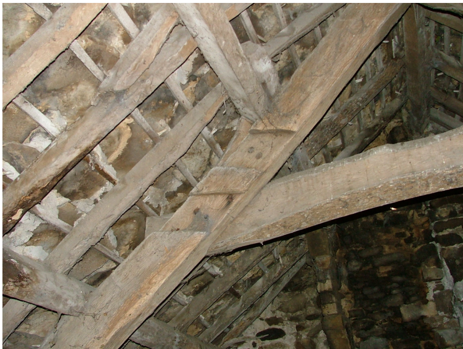
Plate 28 – Detail of the western truss showing evidence of reuse
