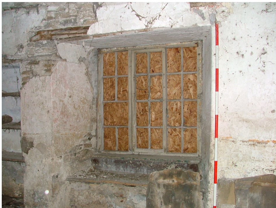
Plate 18 – North elevation of former cottage with Yorkshire sash window frame remaining in-situ (Scale is in 20cm graduations)
