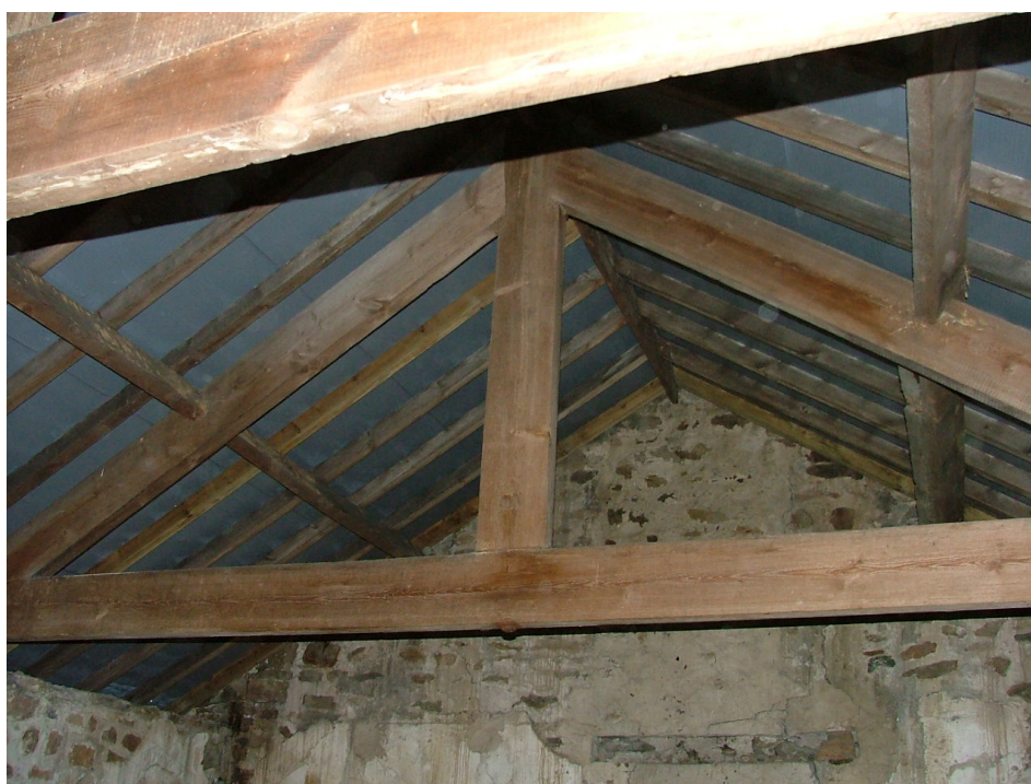
Plate 41 – Roof truss, byre
