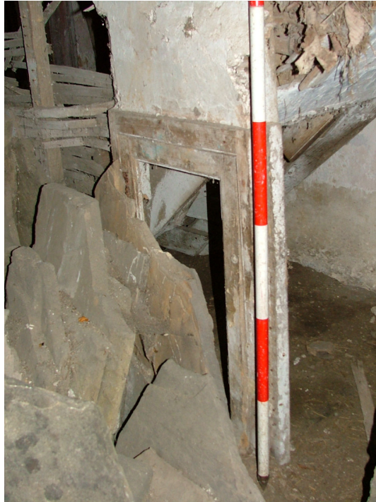
Plate 23 – Small hatch at base of stairs, ground floor of former cottage (Scale is in 20cm graduations)
