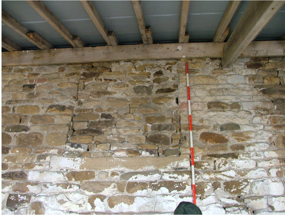
Plate 36 – One of the two blocked-up windows, south elevation of byre (Scale is in 20cm graduations)
