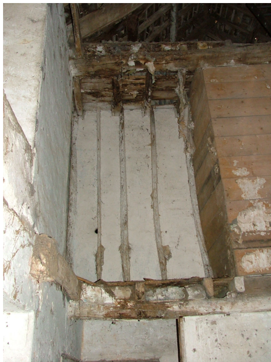
Plate 26 – First floor storage space over the entrance and horizontal boarding of staircase wall
