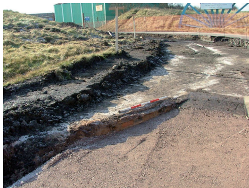
Plate 1: Haig Colliery access improvement works. Note concrete layer sealing red bricks
