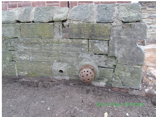
Plate 4: Interior of pond feature showing the head of an outlet pipe.
