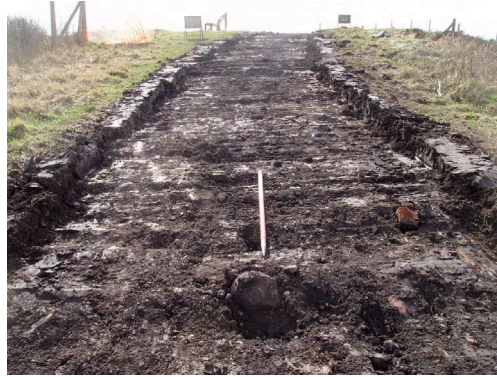
Plate 3: Pathway excavation on the Howgill Incline.
