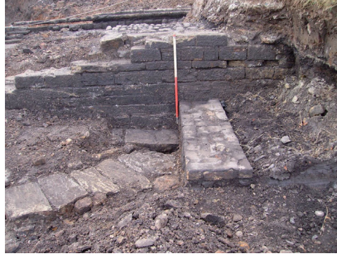
Plate 5: Tooled north face of north wall (112). Also shown is brick wall (113) and culverts (115) and (117).
