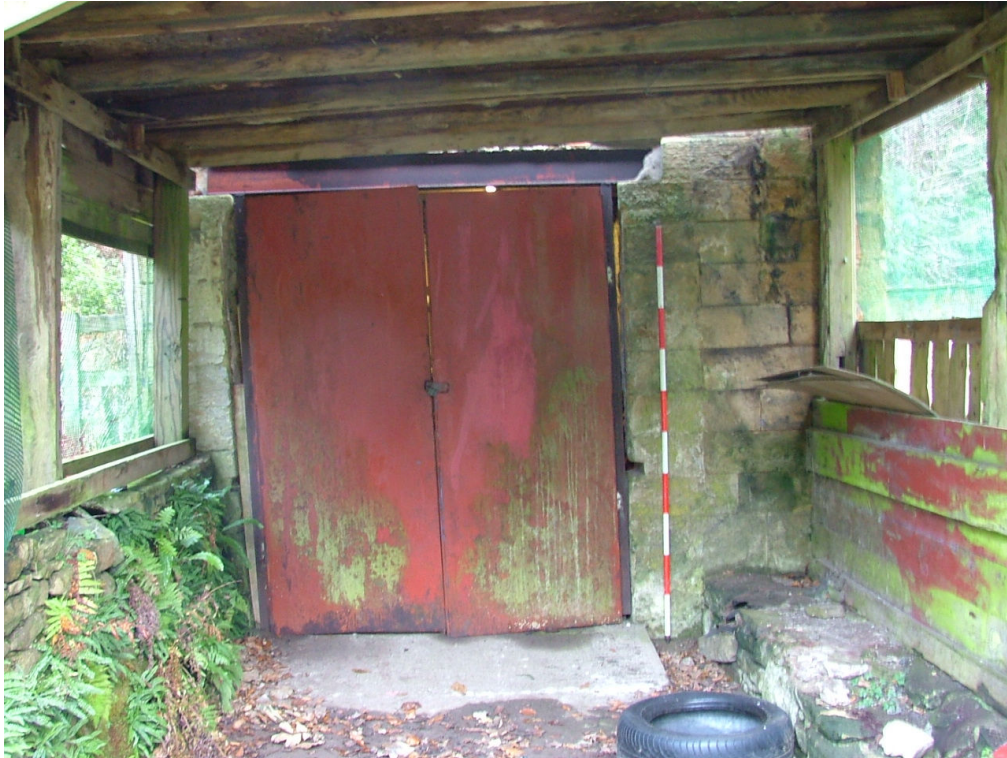
Plate 14 – Large doorway, west elevation of The Bothy (Scale = 2m)
