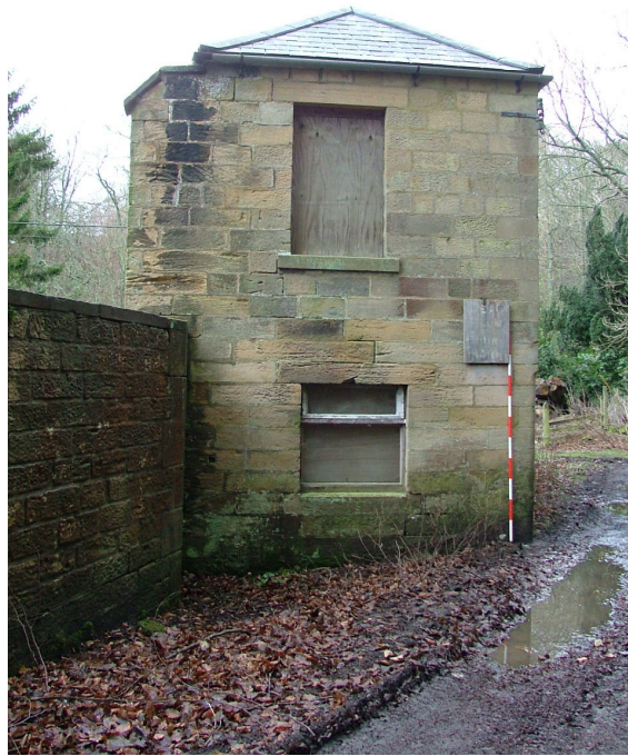
Plate 4 – East elevation of The Bothy (Scale = 2m)
