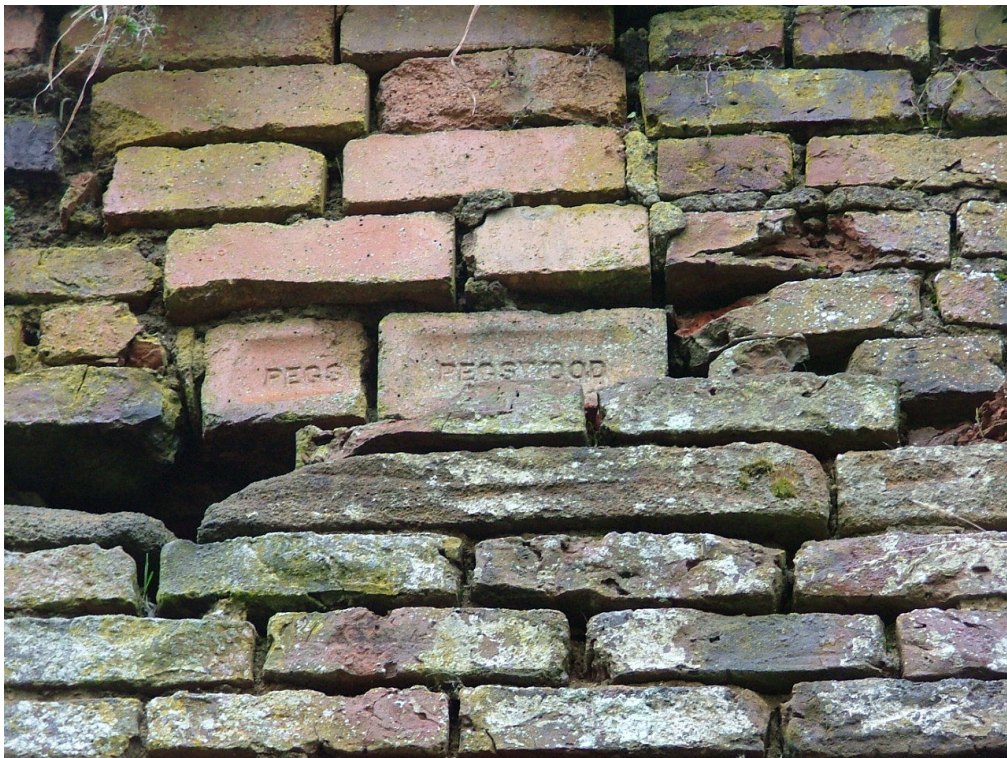
Plate 23 – Detail of 'Pegswood' bricks in south elevation of The Bothy
