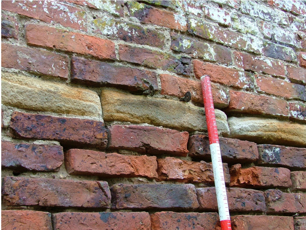
Plate 18 – Detail of brickwork and masonry string course, south elevation
