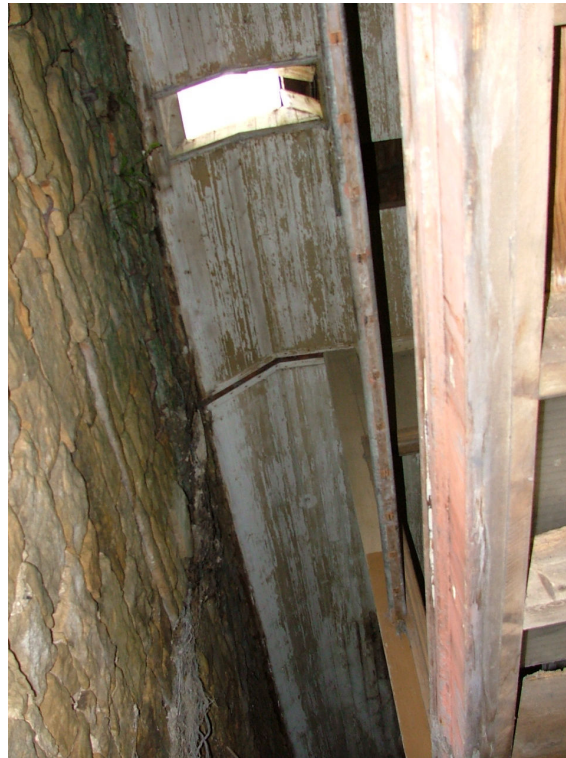
Plate 28 – View of the first floor ceiling showing skylight and boarding
