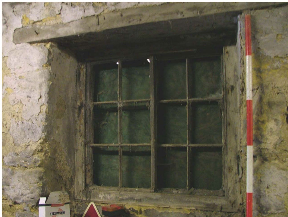
Plate 27 – Yorkshire sash window, north elevation of The Bothy (Scale is in 20cm graduations)
