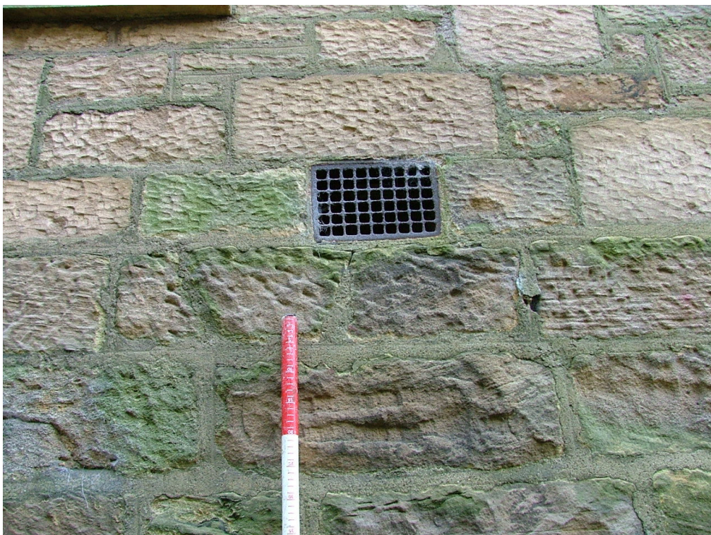
Plate 11 – Detail of one of the ventilation grilles in the north elevation
