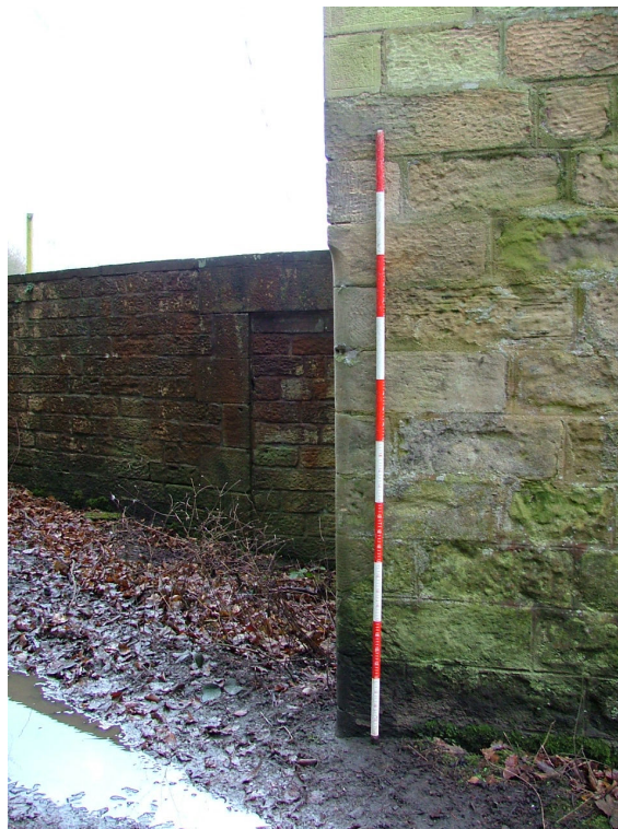
Plate 5 – North-east corner of The Bothy showing the curved edge to prevent animals and carts from catching on the otherwise sharp edge (Scale = 2m)
