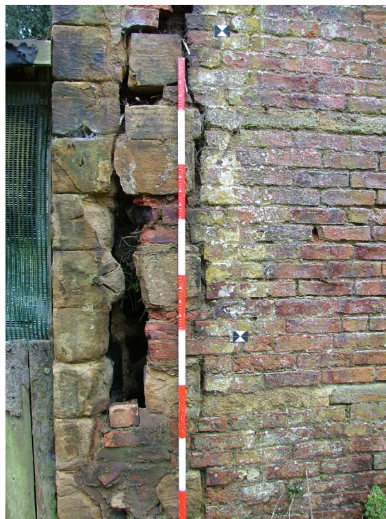
Plate 19 – West side of south elevation showing join between masonry and brickwork (Scale is in 20cm graduations)
