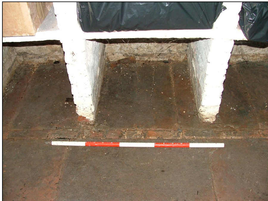
Plate 83 – Detail of course of bricks between sandstone floor, central room of cellar (Scale = 1m)
