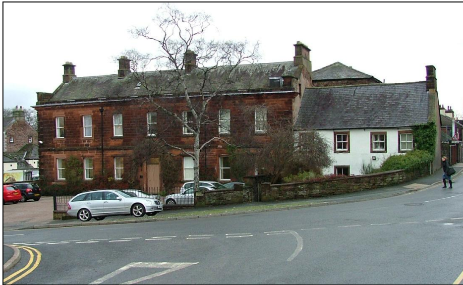
Plate 3 – Hutton Hall as seen from the south-east, showing the red sandstone 18 th century mansion house, with 16 th /17 th century cottage to right, and the pyramid roof of the pele tower behind
