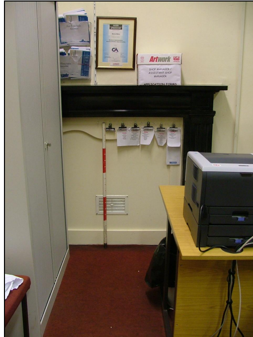
Plate 52 – Fireplace in south-west end wall, ground floor of mansion house (Scale = 1m)
