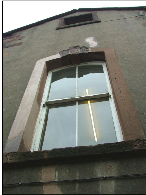
Plate 45 – First floor stair window and attic window above
