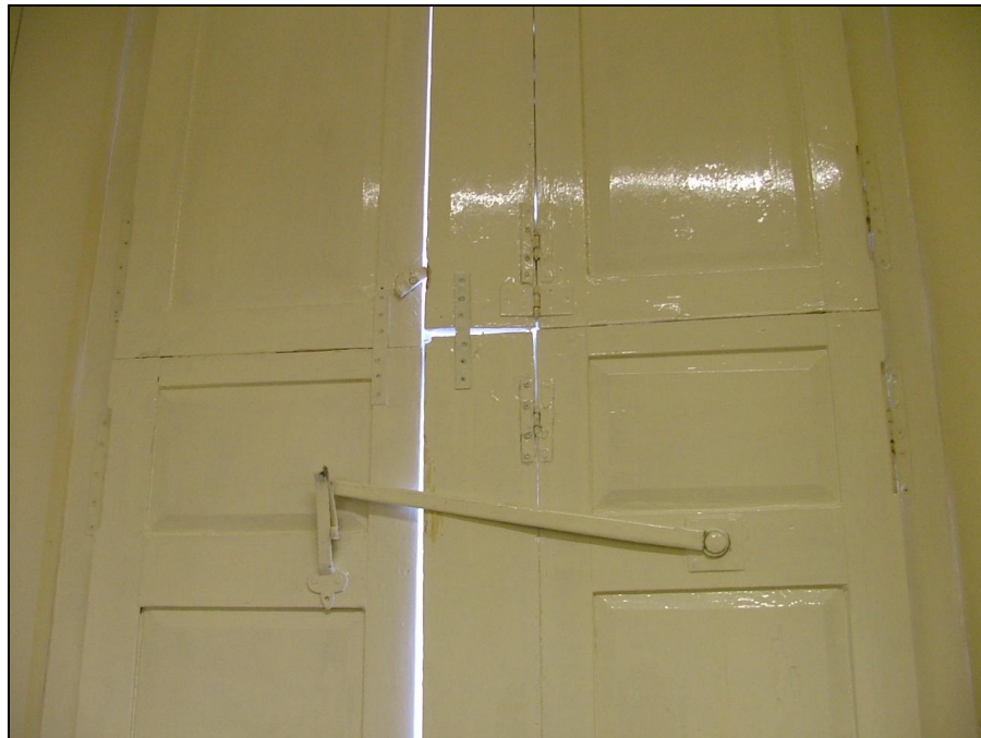
Plate 59 – Detail of hinges and hook stay, ground floor shutter, mansion house
