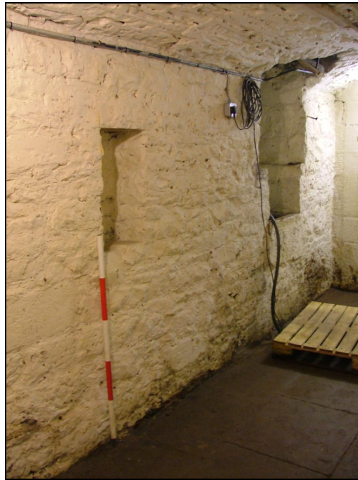
Plate 84 – Niche and stone sink with semi-circular feature above, north-west wall of cellar (Scale = 1m)
