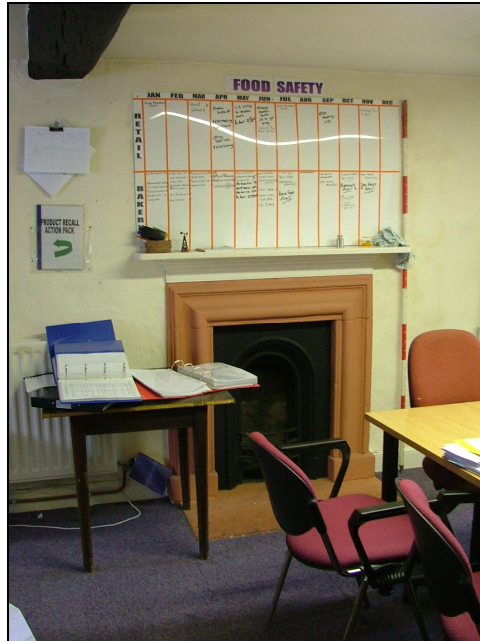
Plate 21 – Bolection-moulded fireplace, second floor of pele tower (Scale = 2m)
