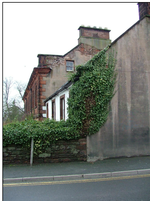
Plate 41 – South-west elevation of mansion house showing blocked first floor and attic windows, note the pitched roof of the 20 th century thin extension to left of main house and ranging pole
