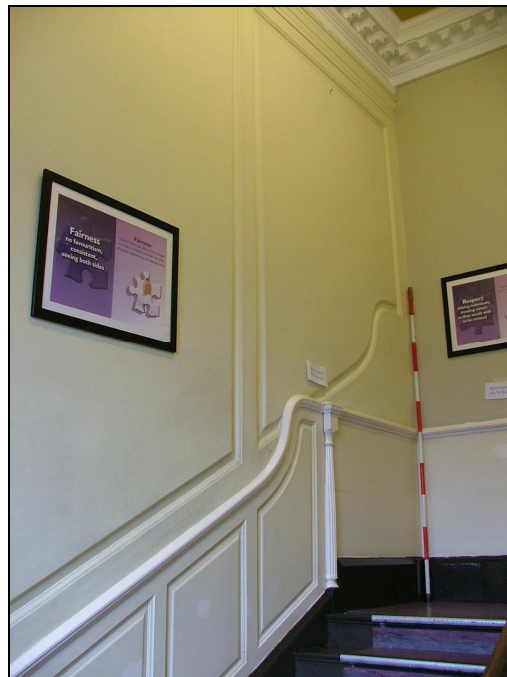
Plate 61 – Panelling, first floor of staircase in mansion house (Scale = 2m)
