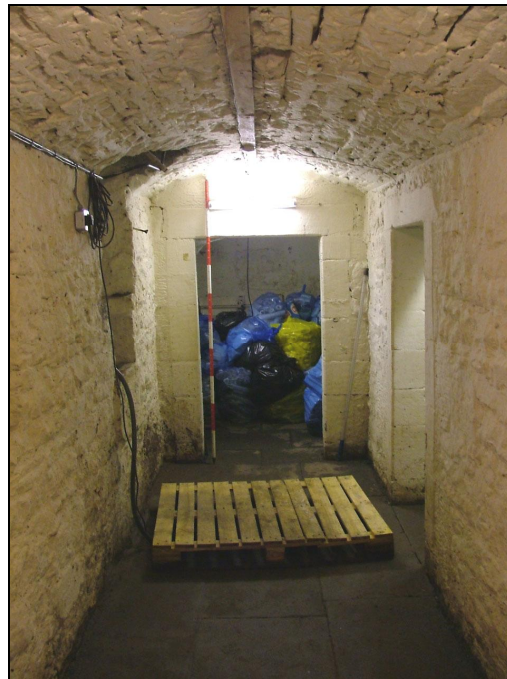
Plate 81 – View looking north-east of cellar below mansion house, note the stone walls and door surrounds, stone flagged floor and brick vaulting (Scale = 2m)
