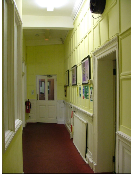
Plate 54 – View looking south-west down corridor from door into cottage showing panelling, modern office partition to left, and former doorway to exterior on right
