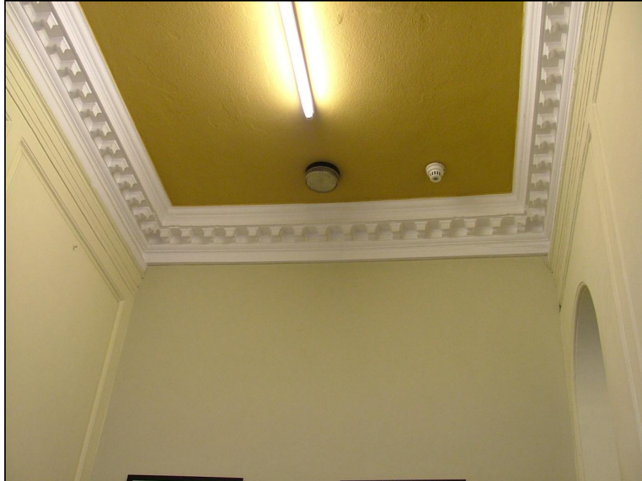
Plate 62 – Dentilated cornice, first floor of main staircase. Note the lack of panelling and coving below one wall suggesting this is a later insertion
