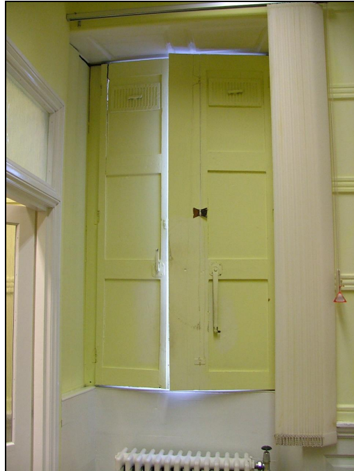
Plate 58 – Shutter, ground floor of mansion house
