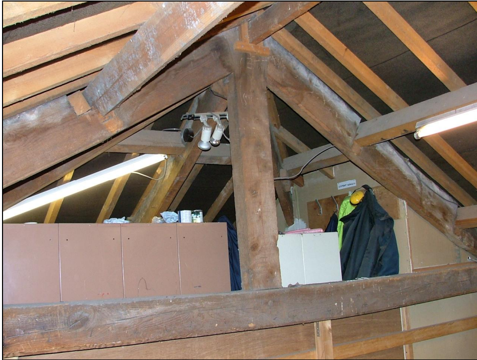
Plate 95 – Roof truss, stable block
