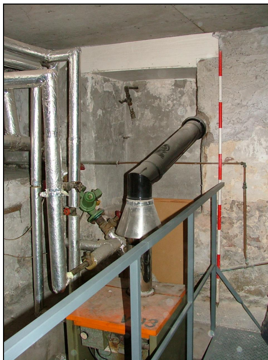
Plate 15 – Ground floor of pele tower, ?blocked window in north-west wall (Scale = 2m)
