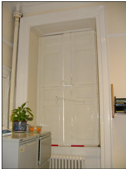
Plate 57 – Detail of shutters, ground floor of mansion house (Scale = 1m)
