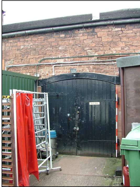
Plate 94 – Large doorway in north-east elevation of stable block (Scale = 2m)
