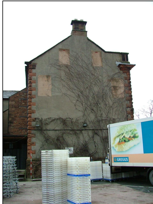
Plate 41 – South-west elevation of mansion house showing blocked first floor and attic windows, note the pitched roof of the 20 th century thin extension to left of main house and ranging pole
