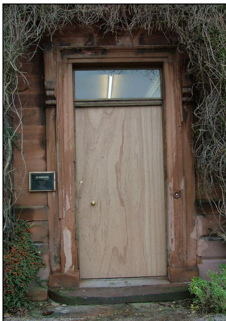
Plate 38 – Main doorway, south-east elevation of mansion house
