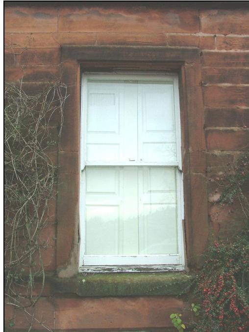
Plate 39 – Detail of ground floor window, south-east elevation of mansion house
