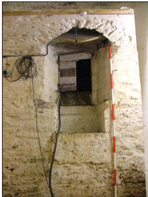
Plate 85 – Recess in north-west wall of cellar, with small wooden door and stone sink
