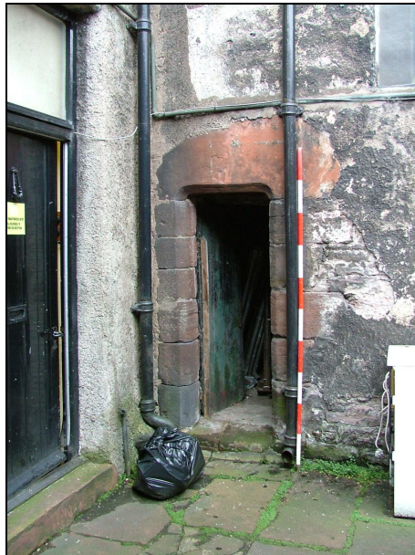
Plate 8 – Doorway, north-east elevation of pele tower (Scale = 2m)
