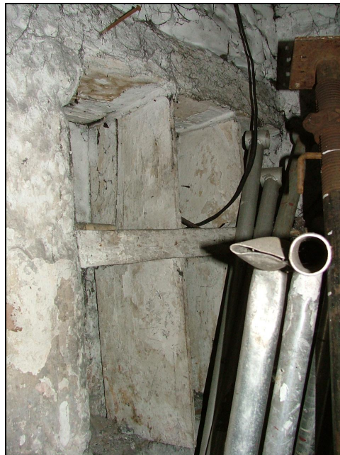
Plate 13 – Blocked window, ground floor, SE wall of pele tower
