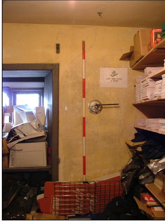
Plate 25 – Remains of gas light fitting, third floor of pele tower (Scale = 2m)
