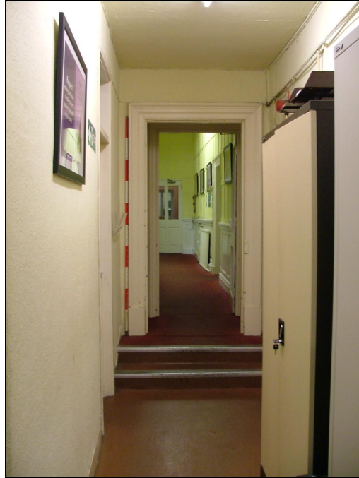
Plate 31 – View looking south-west from the cottage showing the difference in ground floor level between the cottage and the mansion house
