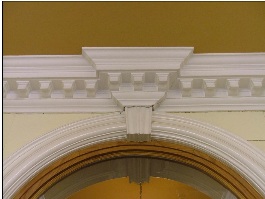
Plate 48 – Detail of dentilated cornice and architrave
