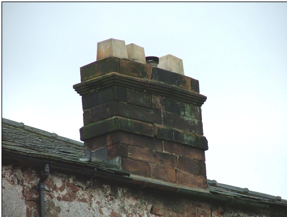
Plate 6 – Chimney stack, north-west elevation of pele tower
