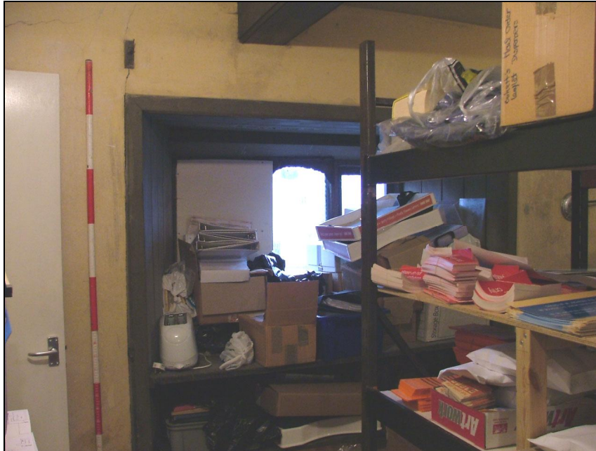
Plate 23 – Third floor of pele tower, window in south-west wall
