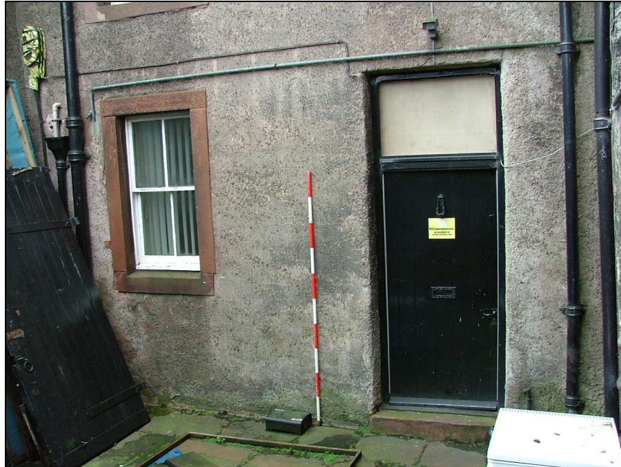
Plate 29 – North-west elevation of cottage (Scale = 2m)
