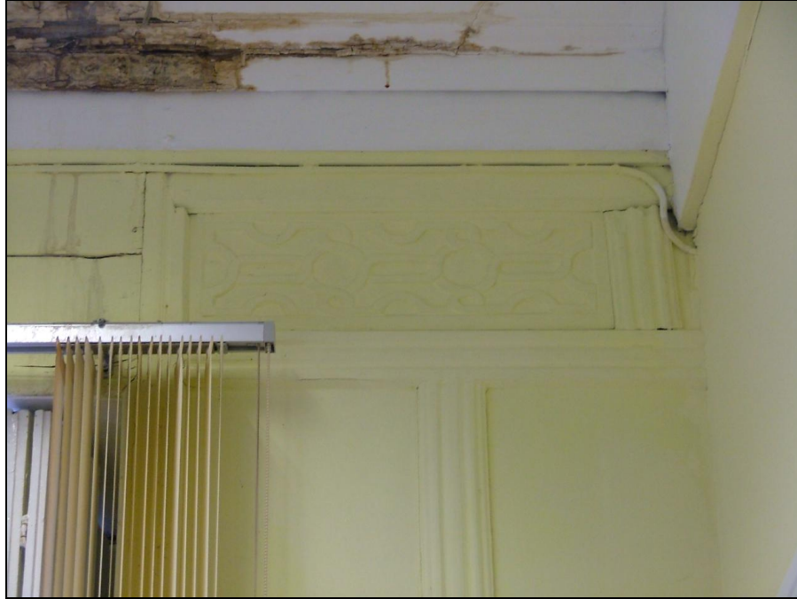
Plate 56 – Detail of panelling against south-east internal wall, ground floor of mansion house
