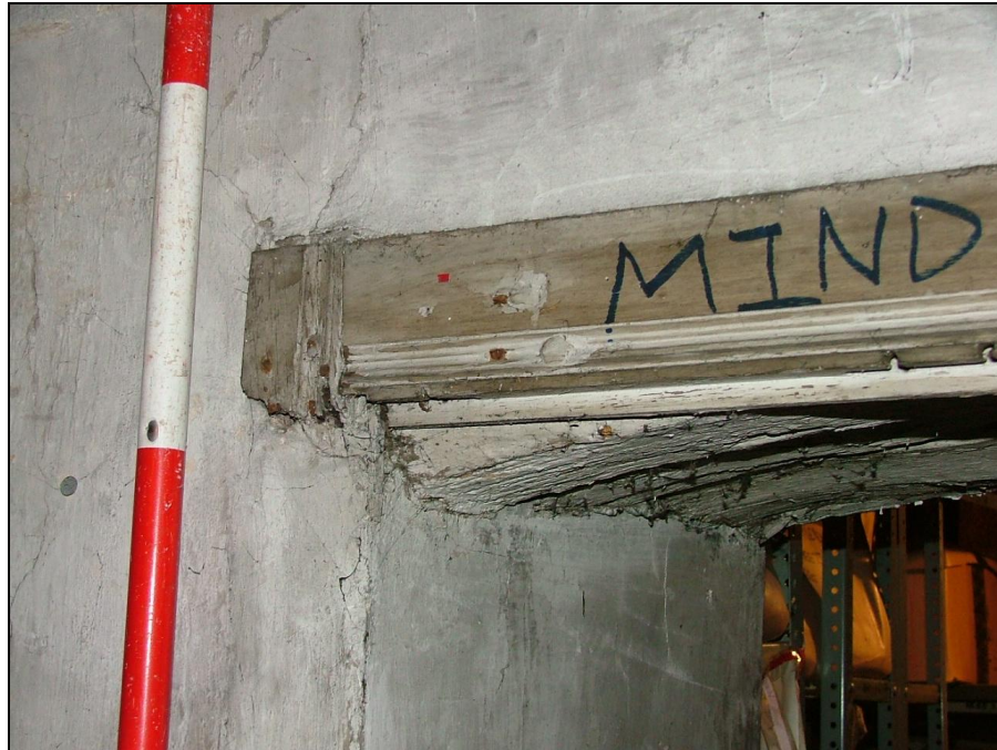
Plate 69 – Remains of some of the possible original architrave, doorway in attic of mansion house (Scale is in 20cm graduations)
