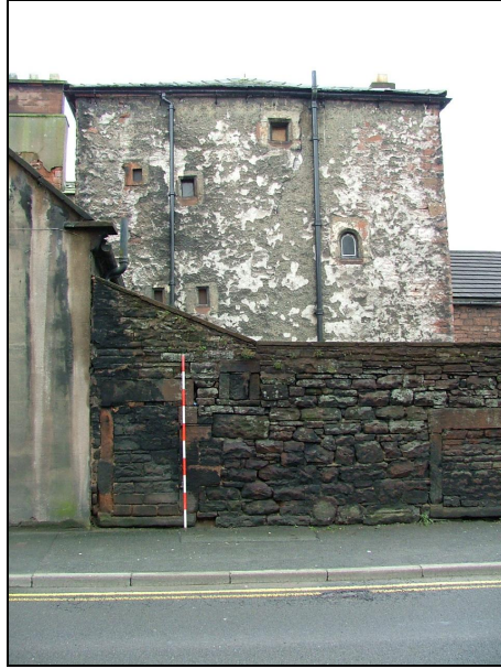
Plate 7 – North-east elevation of pele tower, note the blocked windows in the boundary wall which may relate to a now missing building located against the north-west wall of the cottage
