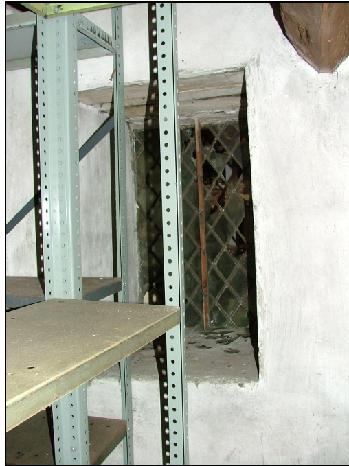
Plate 71 – Window in cross-wall of attic, still retains some diamond glass panes within lead cames, and a central vertical piece of wood to which some of the cames are tied
