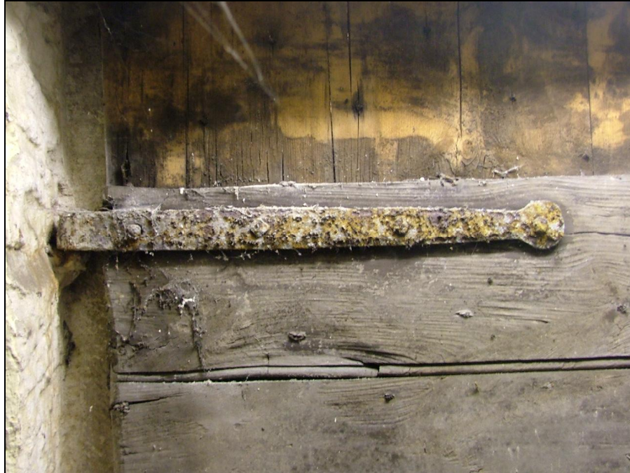
Plate 88 – Detail of strap hinge, cellar door
