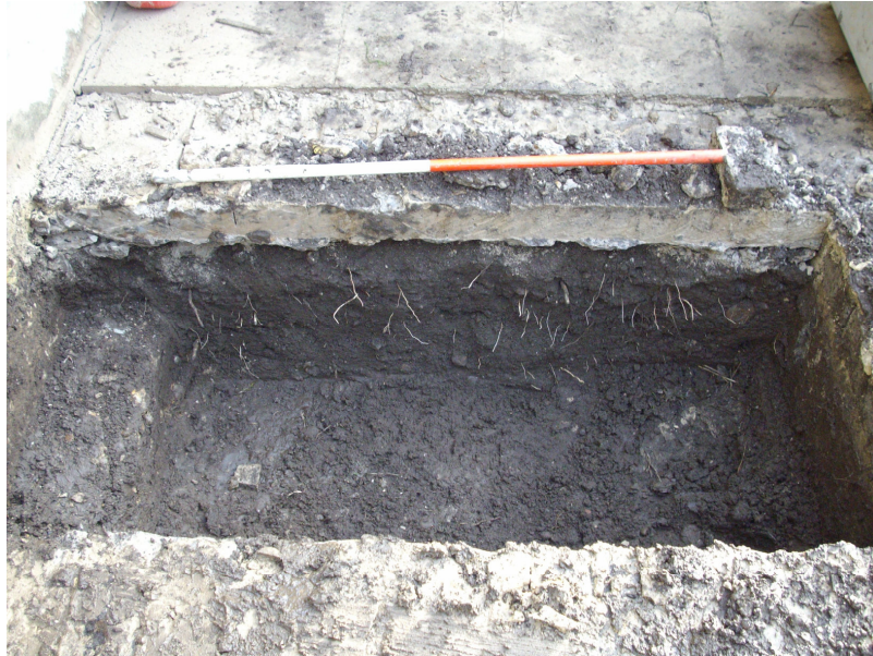
Plate 2: Section of Foundation Trench No. 1, facing east
