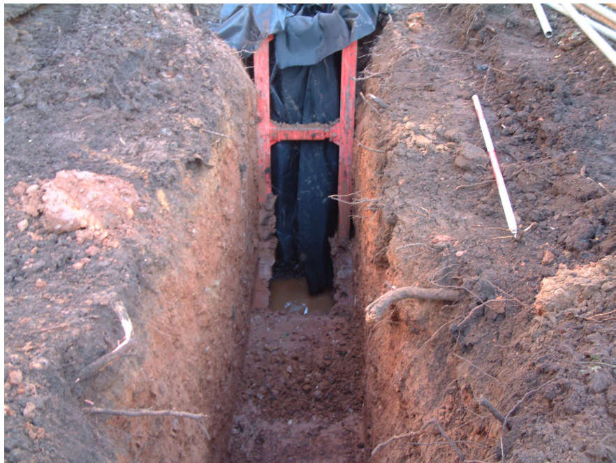
Plate 1: View east along gas trench
