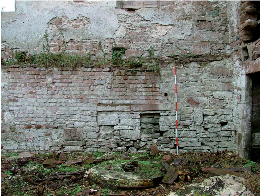
Plate 55 – Northern interior wall of main mill building
