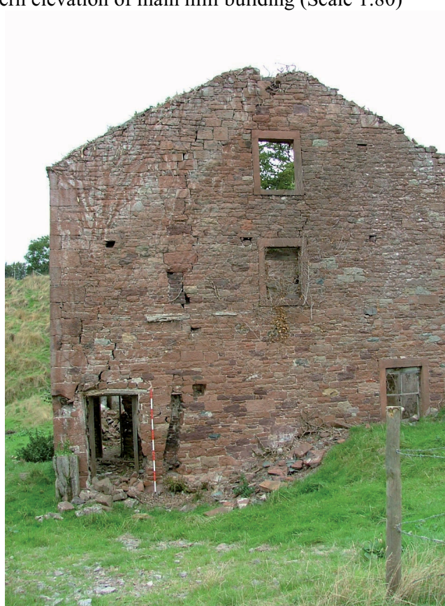
Plate 41 – Southern elevation of main mill building
