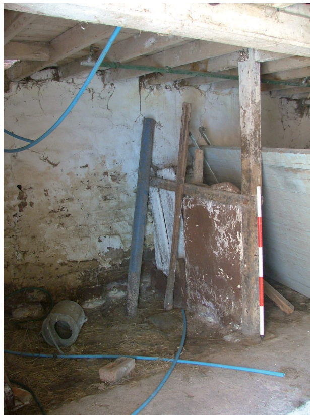
Plate 20 – Interior of northern byre in Building ‘D’
