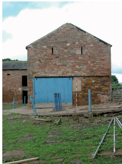
Plate 25 – Eastern gable end of ‘E’
