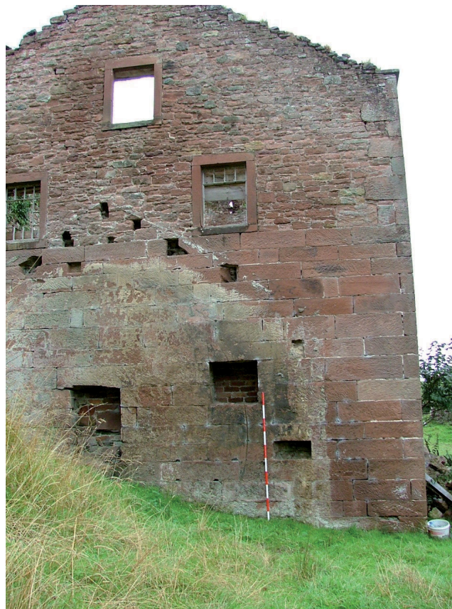
Plate 45 – Northern elevation. The scarring of the water-wheel is visible just to the left of the ranging pole
