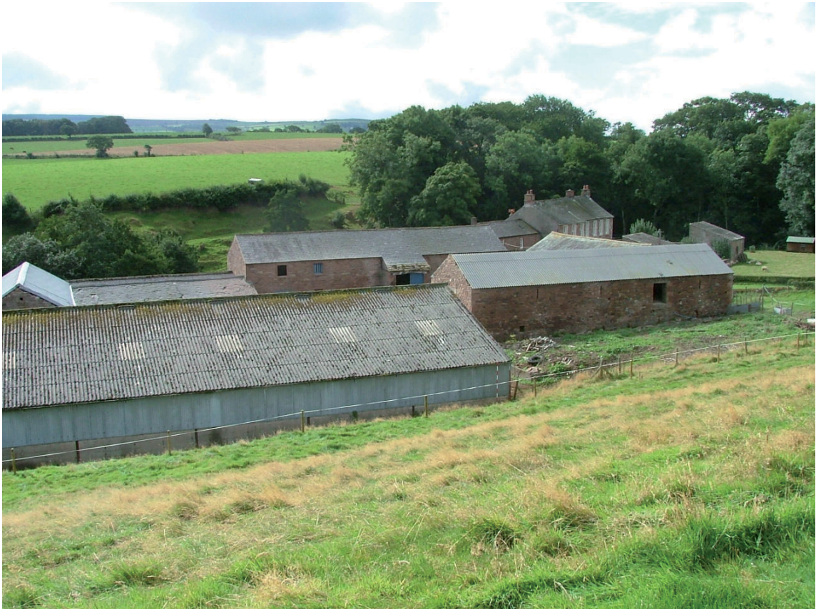
Plate 1 – The farm buildings and house beyond, Islekirk Hall, as seen from the north-east
