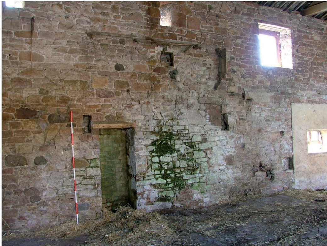
Plate 8 – Southern interior wall of 'A' showing features related to threshing cereals
