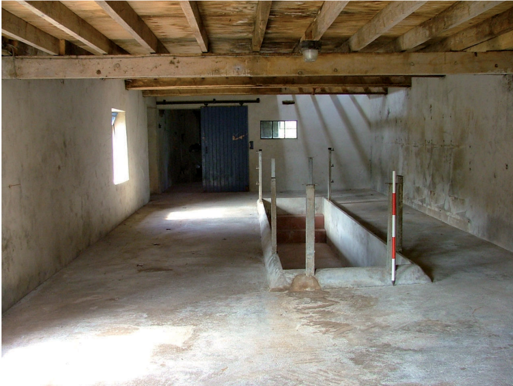
Plate 26 – Interior of ‘E’, showing pit for milking parlour and modern ceiling
