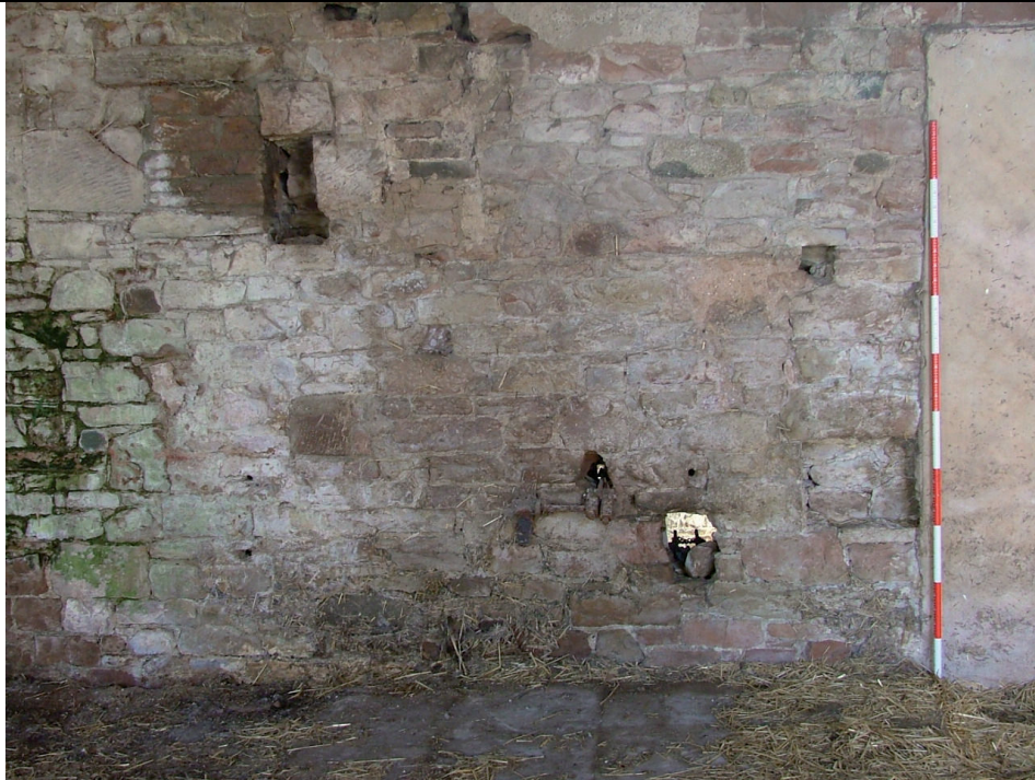
Plate 9 – Blocked aperture (left hand side) and lower hole for drive shaft?
