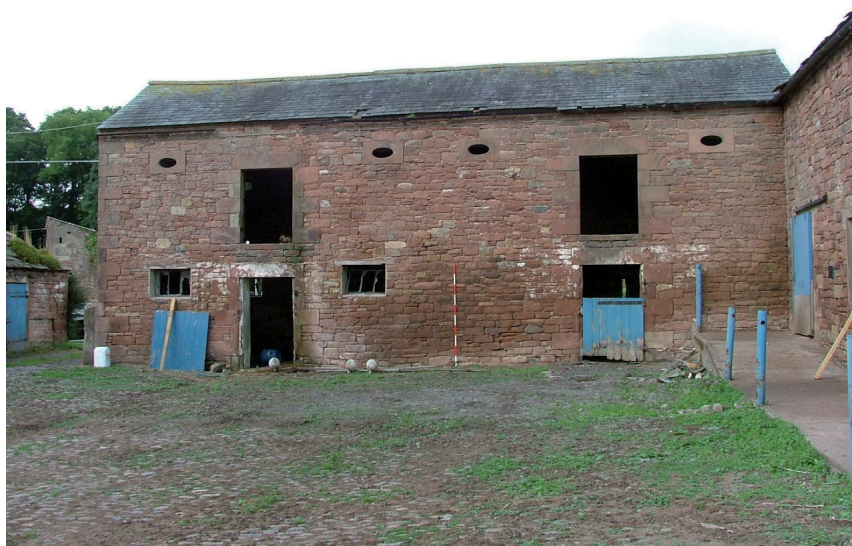
Plate 18 – Eastern elevation of ‘D’
