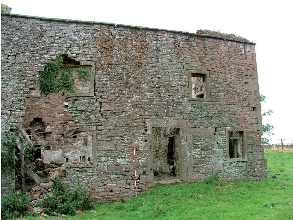
Plate 39 – Western elevation of the mill
