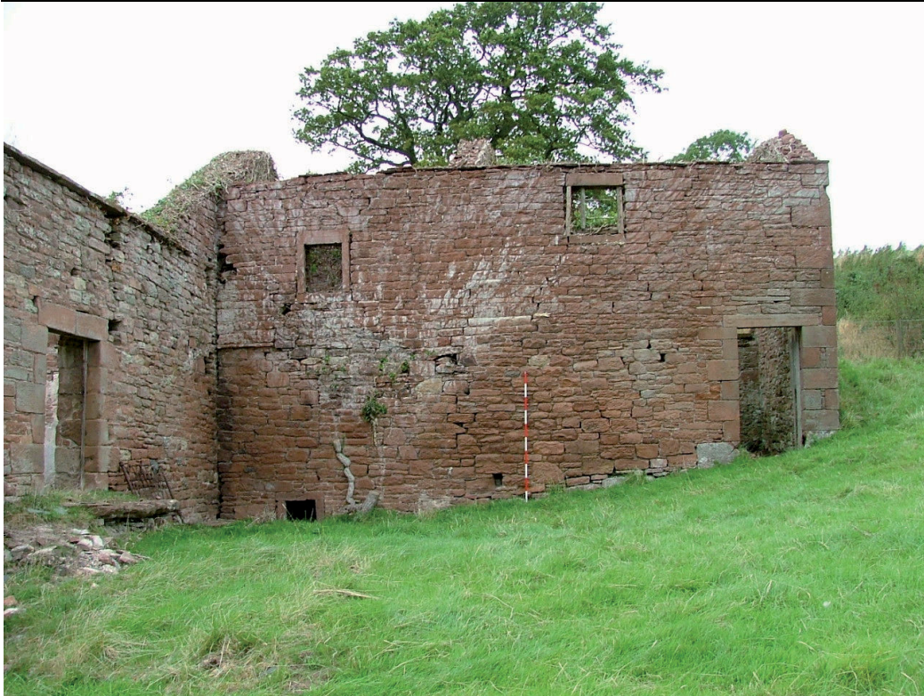
Plate 50 – South facing elevation of rear wing (eastern side) of mill
