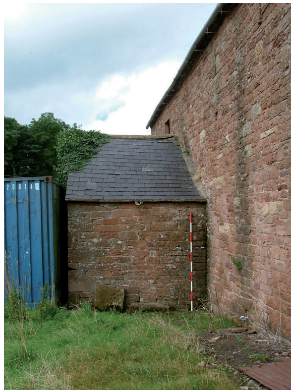
Plate 10 – Eastern elevation of building on S elevation of 'A', a culvert was observed running beneath this structure, parallel to the wall of the barn
