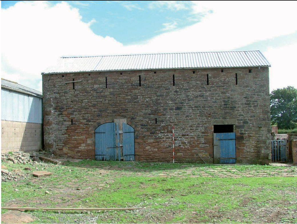
Plate 28 – Western elevation of ‘F’
