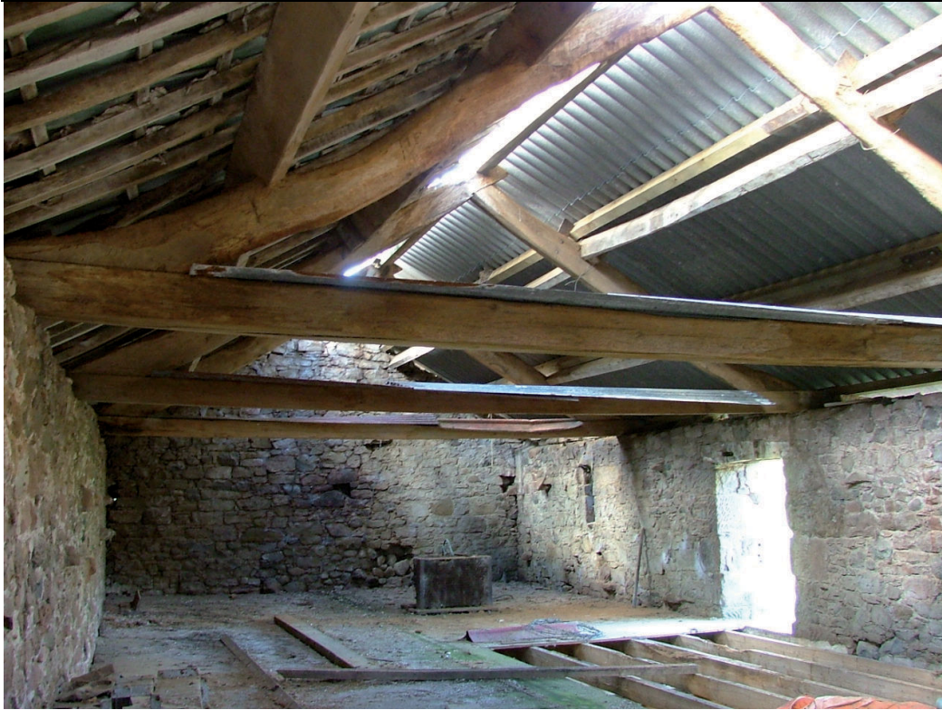
Plate 27 – Roof detail, Building ‘E’
