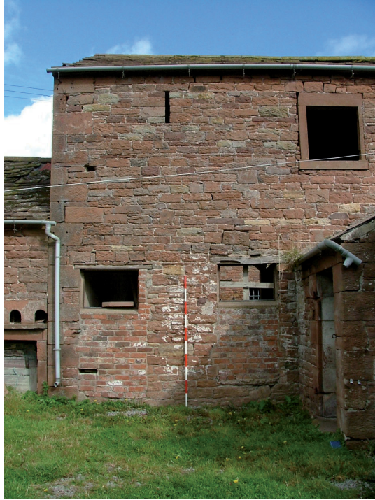
Plate 5 – Two doorways at western end of ‘A’ (south elevation), bricked-up to create windows
