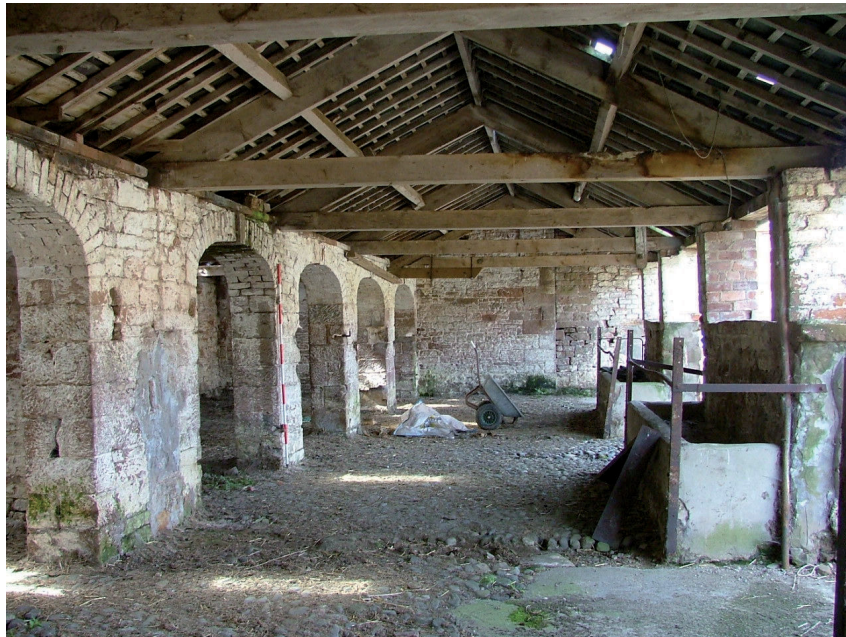
Plate 14 – View looking west showing arched doorways to cart sheds of ‘C’
