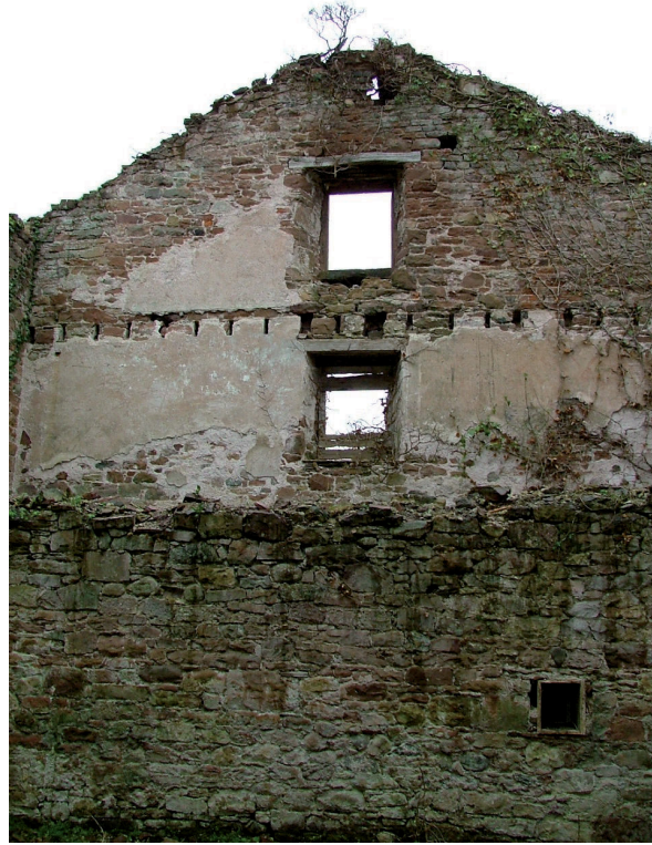
Plate 56 – Southern gable end of the main mill building showing locations of two former floors
