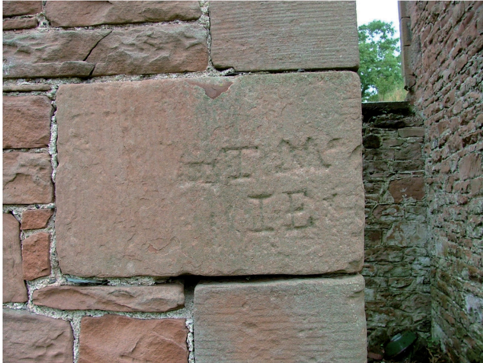
Plate 62 – South facing elevation of the rear wing – initials ‘TM’ and ‘IE’
