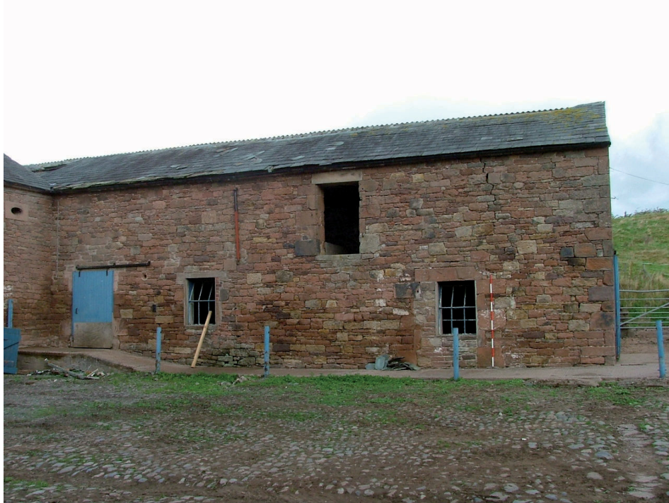
Plate 21 – Southern elevation of Building ‘E’
