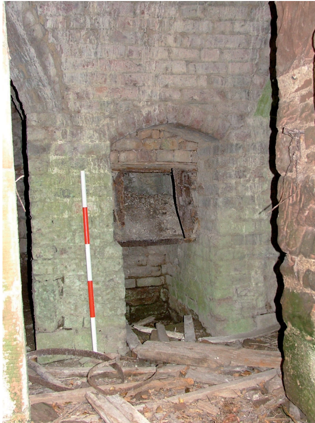
Plate 57 – Base of corn-drying kiln as seen from the main mill building
