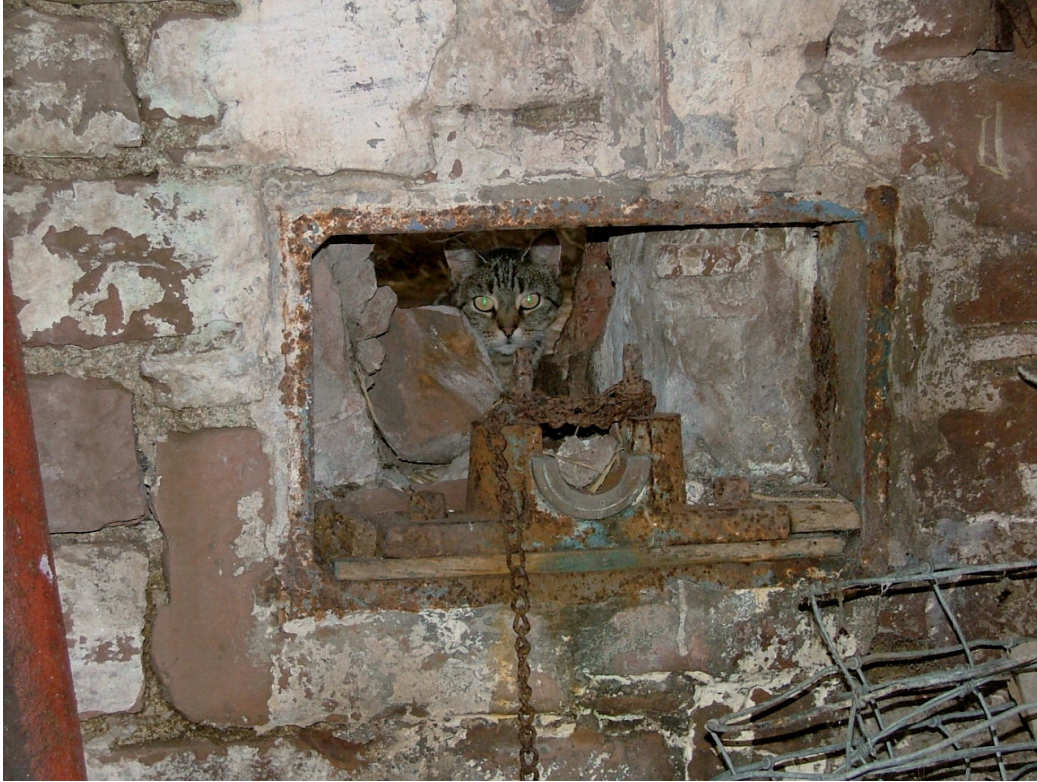
Plate 11 – Housing for a drive shaft for an oil or diesel engine used to power thresher? (Cat included for scale), as seen from the gable structure behind ‘A’
