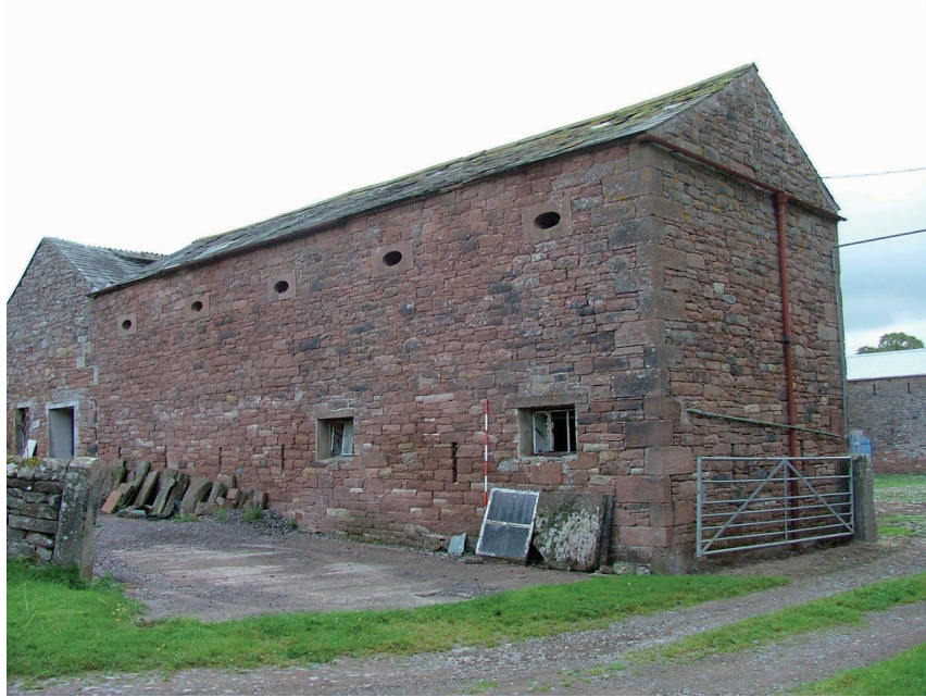
Plate 17 – Western elevation of ‘D’
