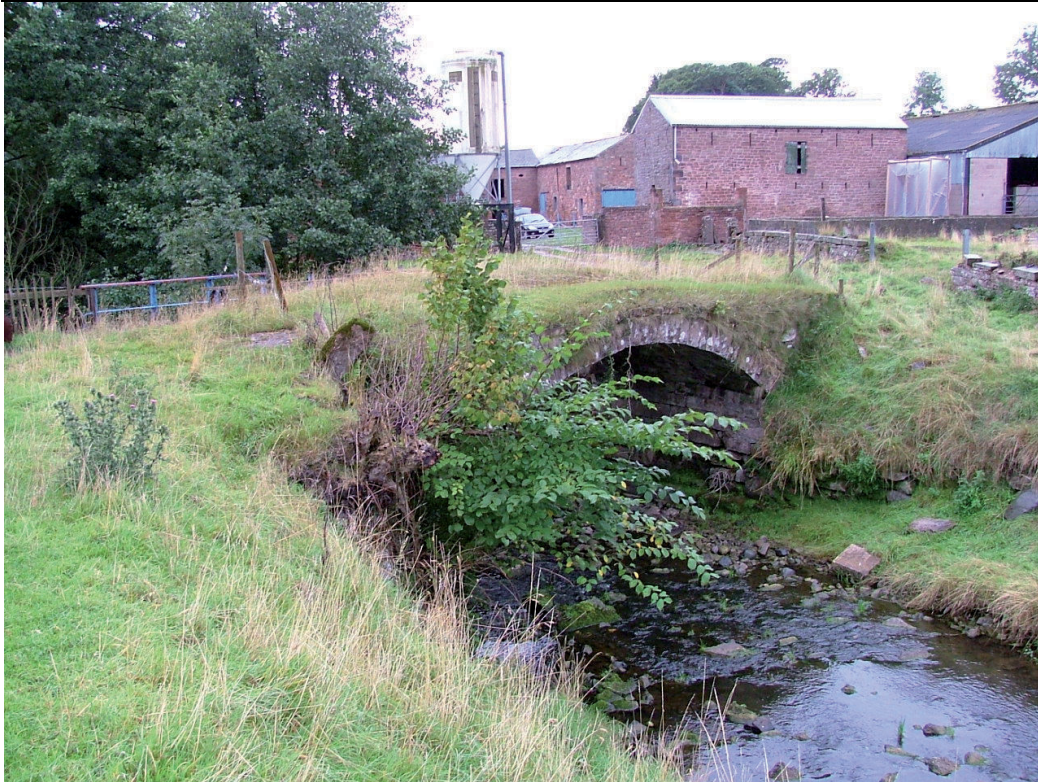
Plate 65 – View of the Packhorse Bridge looking west towards the farm buildings
