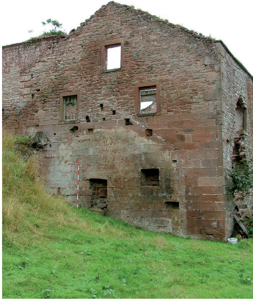
Plate 43 – Northern elevation showing the location of the former wheel-house
