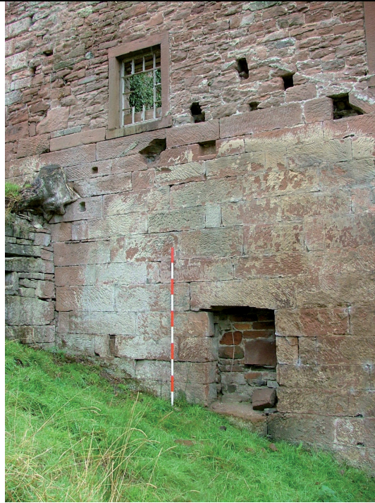
Plate 44 – Former axle hole (now partly blocked) for water-wheel
