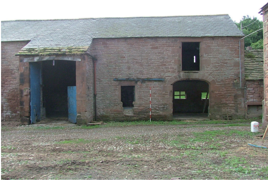
Plate 2 – North facing elevation of the large barn ‘A’
