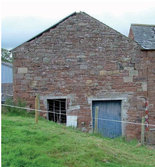
Plate 24 – Western gable end of ‘E’
