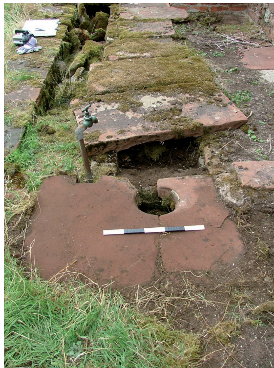
Plate 34 – Tap and circular hole, eastern end of sheep dip (Scale measures 500mm)
