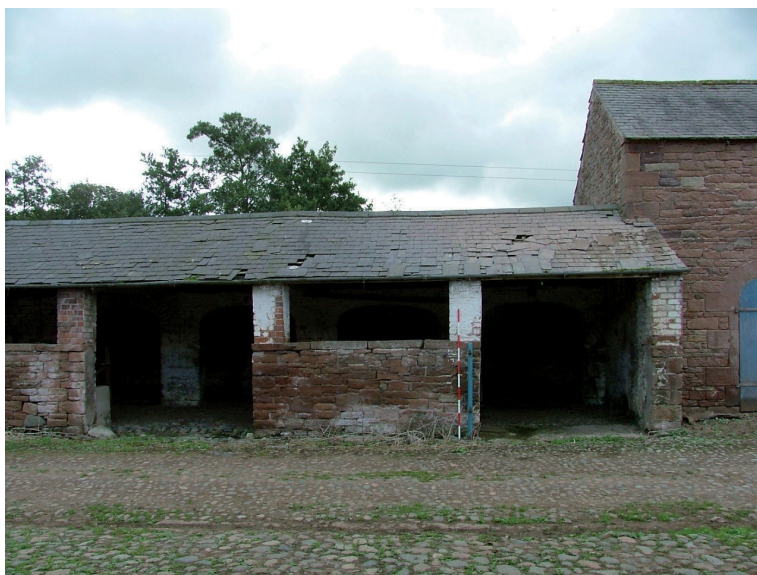
Plate 16 – Shelter shed added to northern elevation, ‘C’
