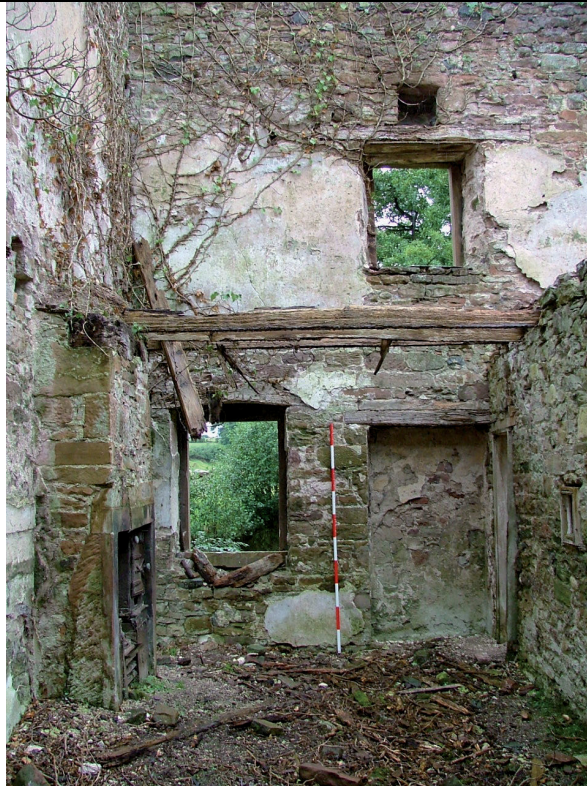
Plate 53 – Blocked doorway and window, western wall of main mill building
