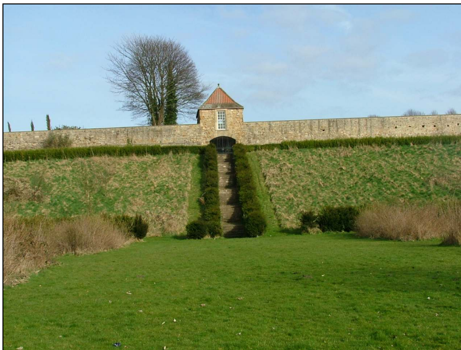
Plate 45 – View looking east of the restored Gardens and Gazebo at Old Durham
