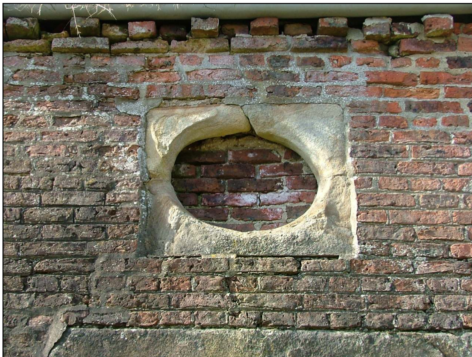
Plate 14 – Detail of ceil-de-boeuf window over doorway in east elevation
