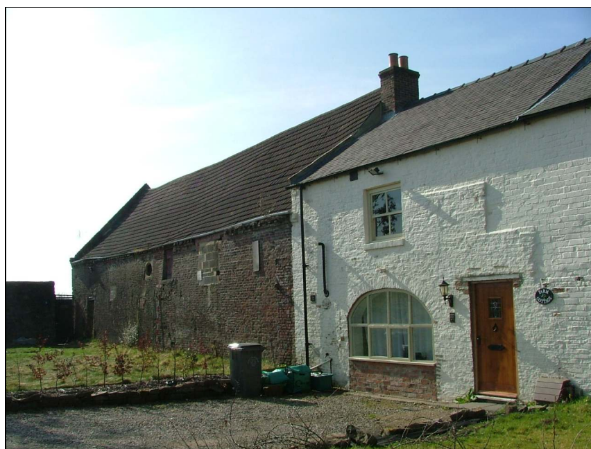
Plate 8 – View looking south-west showing the east elevation of the barn as well as part of Farm Cottage with shows evidence for being partly rebuilt and the arched doorway of a former cart shed
