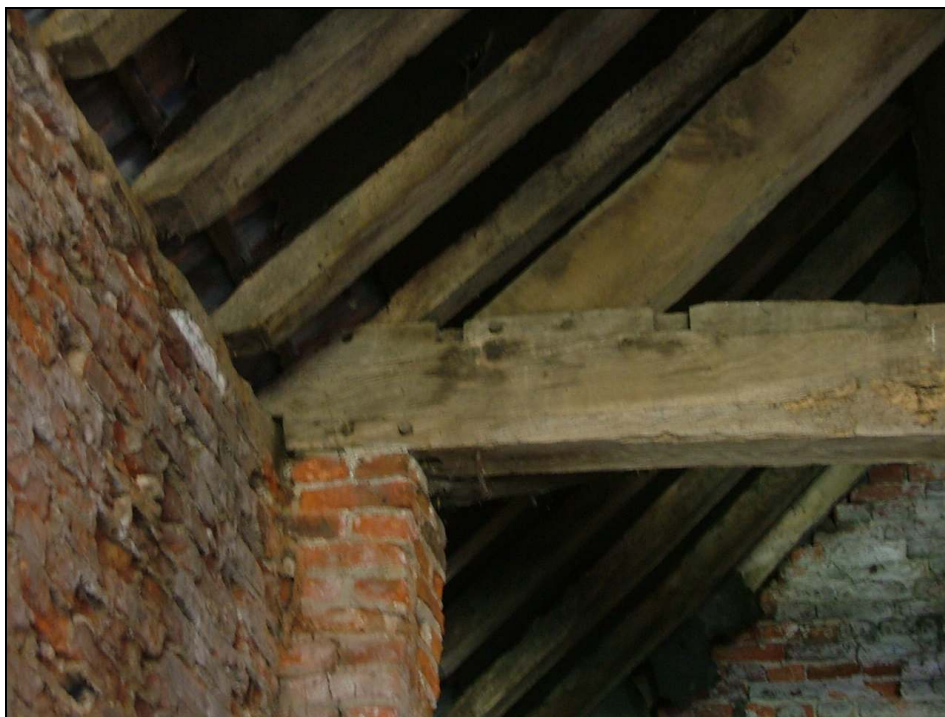
Plate 32 – West end of northernmost tie-beam showing wooden pegs and redundant notches
