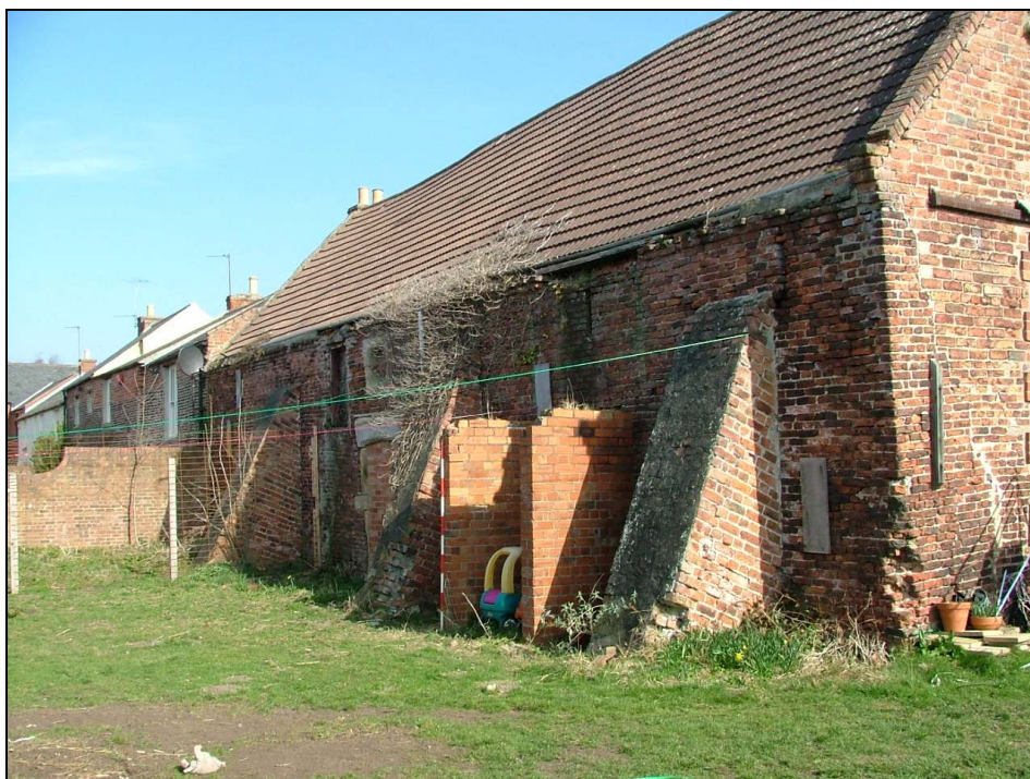
Plate 20 – West elevation as seen from the south-west (Scale= 2m)
