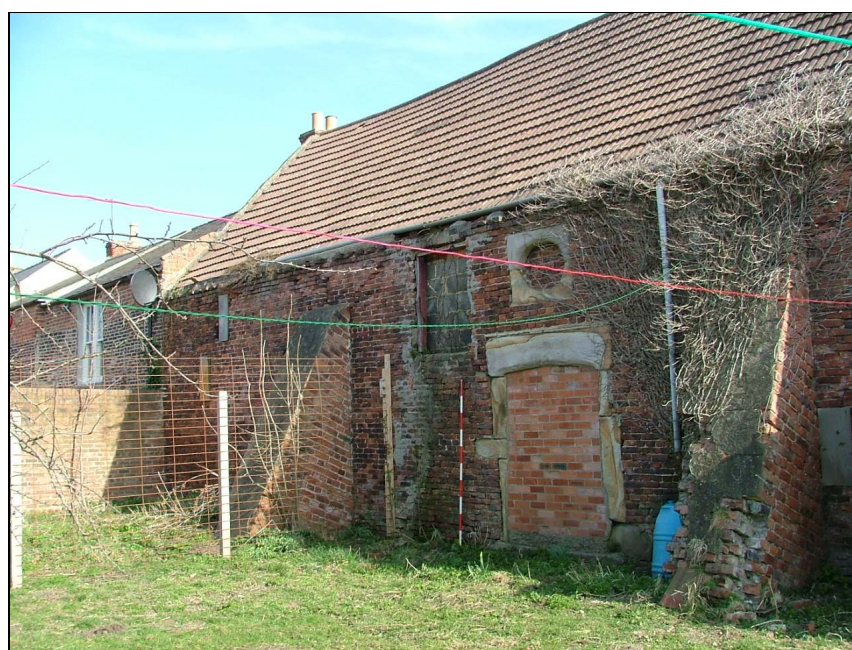
Plate 22 – North end of the west elevation showing two of the diagonal buttresses (Scale = 2m)
