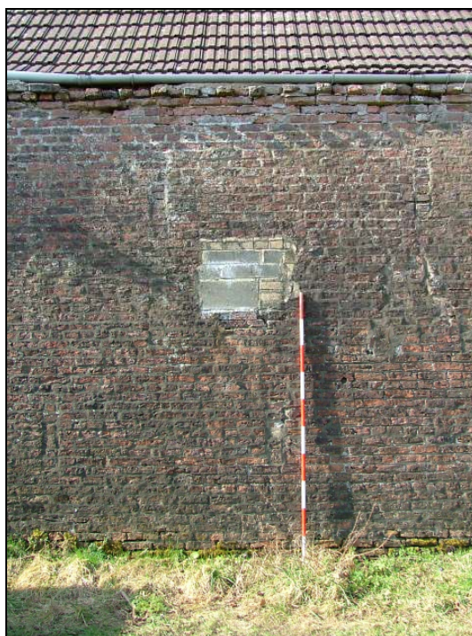
Plate 11 – Blocked aperture, east elevation (Scale = 2m)
