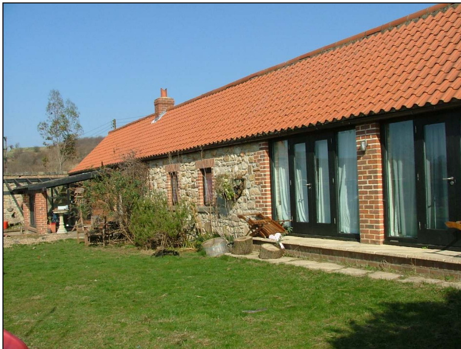
Plate 40 – View looking north-east of the west elevation of The Stables
