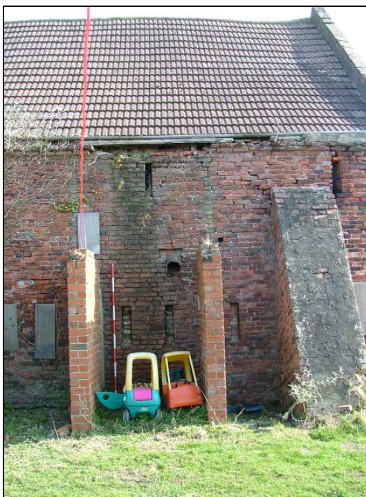
Plate 24 – Two modern brick-built 'piers', west elevation (Scale = 2m)
