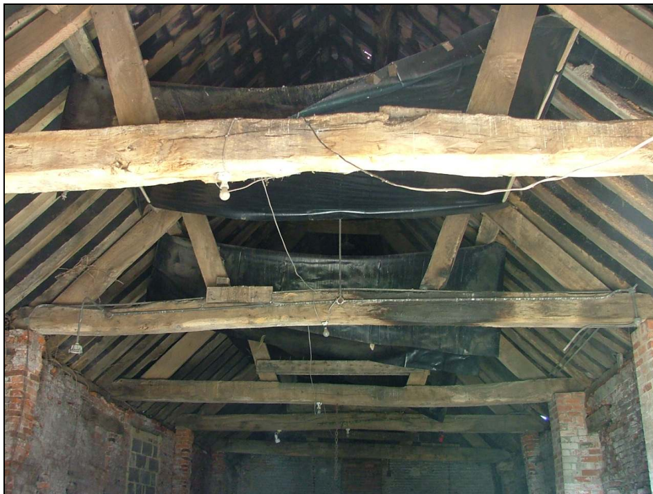
Plate 28 – View looking north of roof trusses
