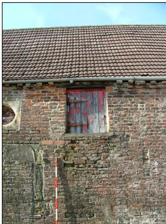
Plate 15 – Opening complete with door, east elevation
