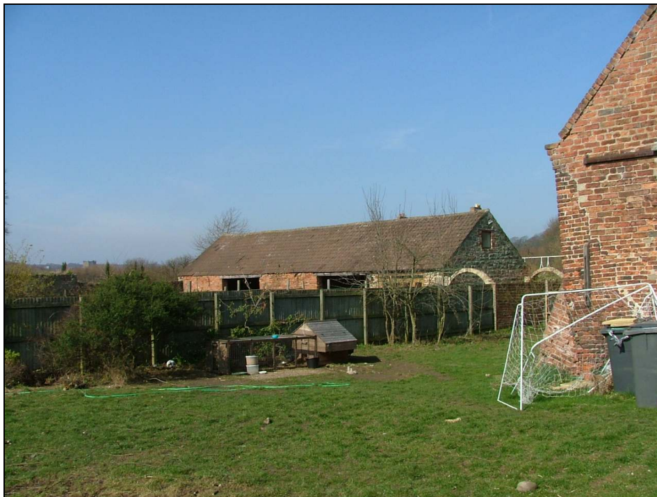
Plate 46 – View looking north-west showing the former cart shed to the west of the barn
