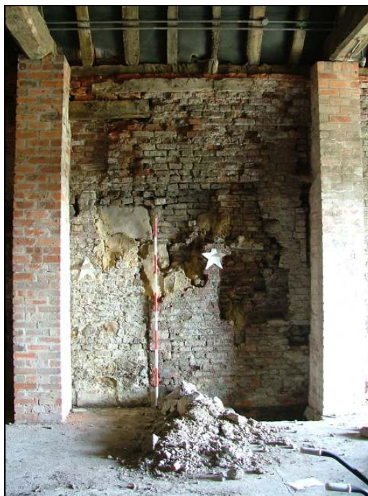
Plate 34 – Area of brickwork removed, east internal elevation (Scale = 2m)
