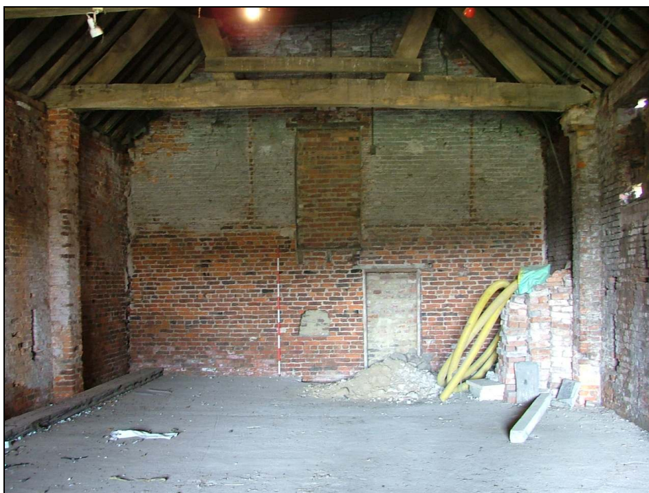
Plate 35 – North internal gable wall of barn (Scale = 2m)
