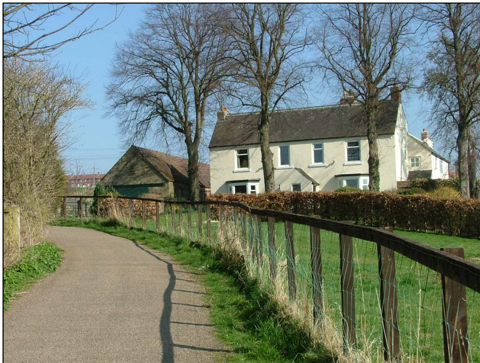
Plate 42 – West elevation of Old Durham Farmhouse
