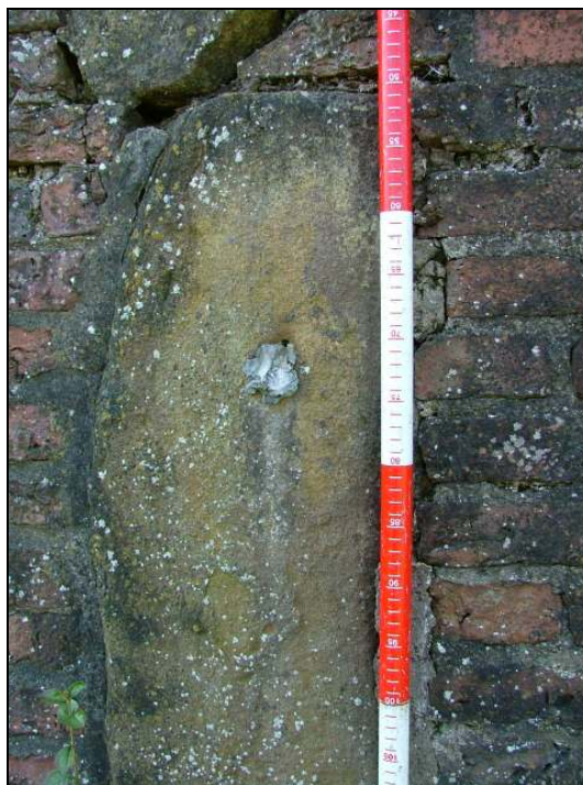
Plate 13 – Detail of lead remaining in-situ, left-hand jamb of door, east elevation
