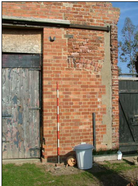
Plate 19 – East side of south elevation showing former doorway (Scale = 2m)
