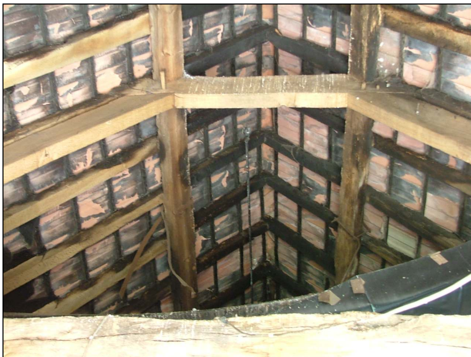
Plate 29 – Detail of one of the roof collars with wooden pegs
