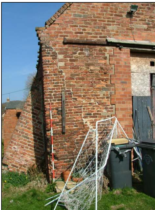
Plate 18 – West side of south elevation showing three phases of brickwork (Scale = 2m)
