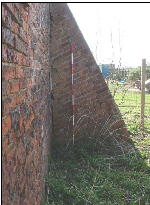
Plate 23 – Detail of one of the buttresses, west elevation (Scale = 2m)
