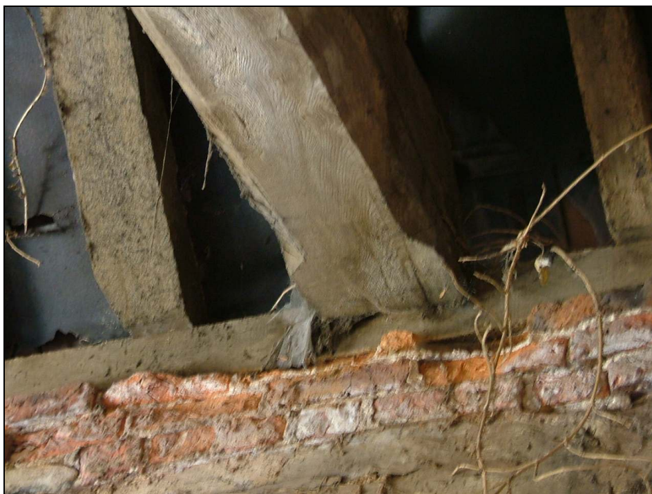
Plate 31 – Detail of end of one of the tie-beams showing chamfered edges
