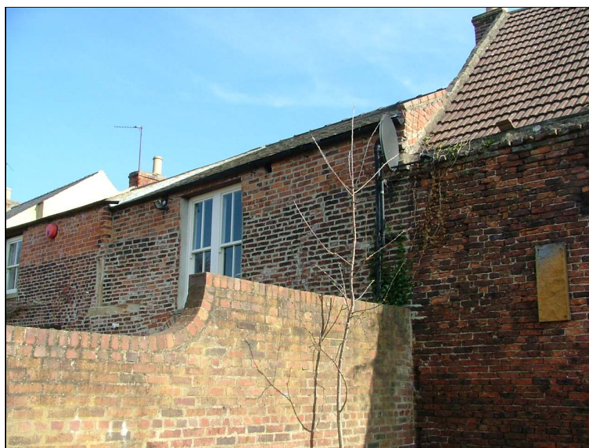
Plate 26 – Part of the west elevation of Farm Cottage showing heightened wall and reused masonry
