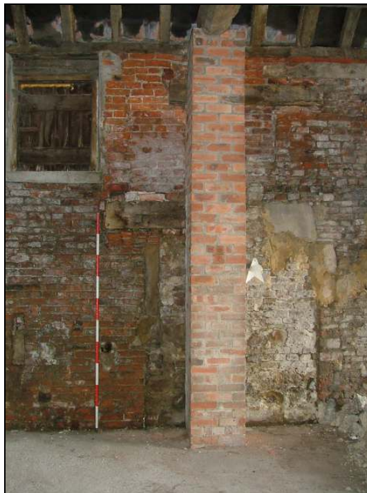
Plate 30 – Modern brick pier, east internal elevation (Scale = 2m)
