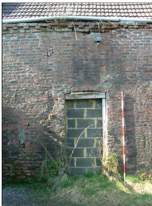
Plate 10 – Blocked doorway, south end of east elevation (Scale = 2m)
