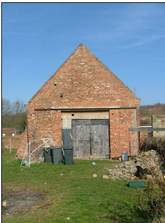
Plate 17 – South elevation of barn (Scale = 2m)
