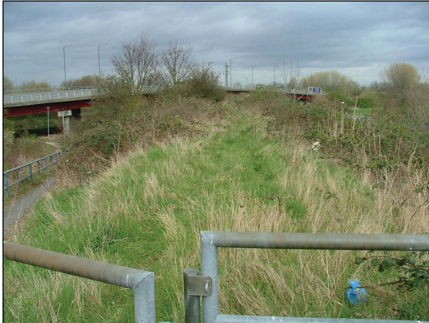
Plate 2 – View looking east of The Ridgeway with the bridge of Eastern Way visible in the background
