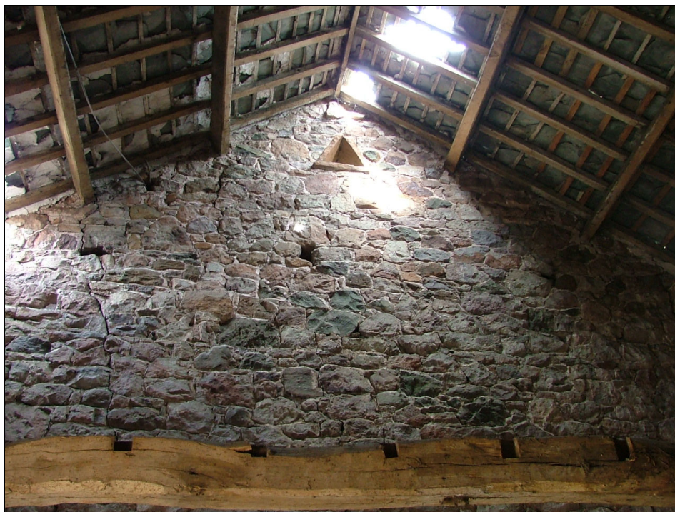
Plate 27 – North internal gable of East Byre showing triangular owl hole and uncovered walls for former hay loft
