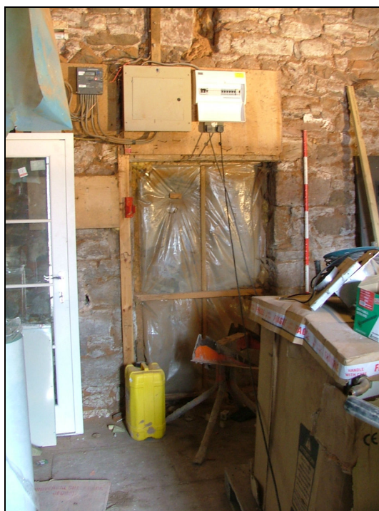
Plate 16 – Blocked doorway in west elevation, West Barn (Scale = 2m)
