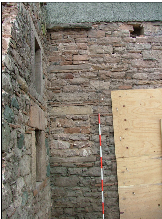
Plate 54 – Detail of two blocked windows to possible former stable with granary above (Scale = 2m)
