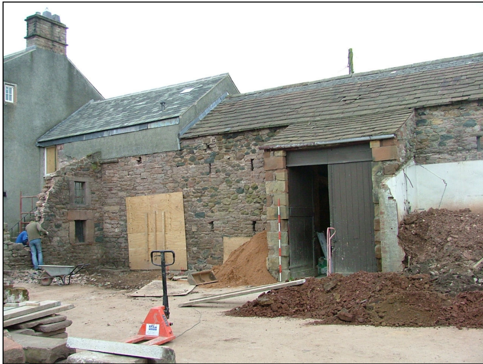
Plate 9 – East elevation of West Barn and part of the house which appears to be contemporary with the barn (Scale = 2m)
