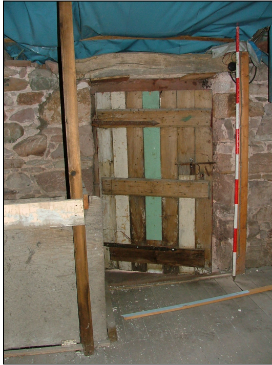
Plate 33 – First floor of East Byre showing pitching door (Scale = 2m)
