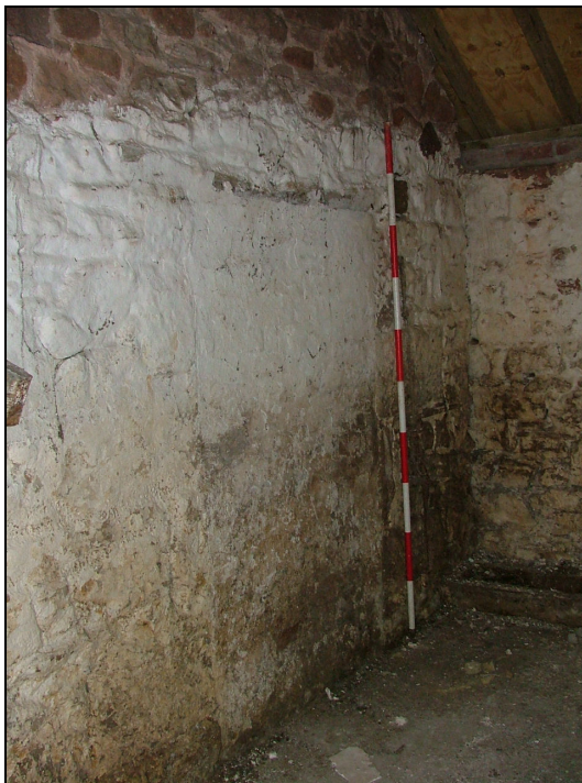
Plate 40 – Blocked doorway between loose box/stable and shelter shed/cart shed (Scale = 2m)
