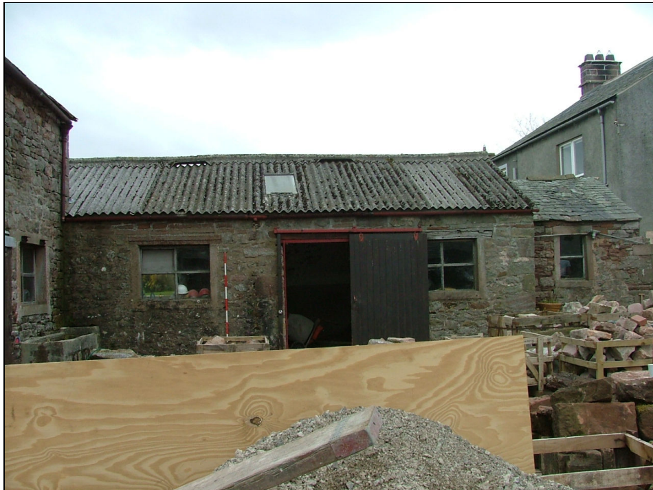
Plate 42 – North elevation of South Range (Scale = 2m)
