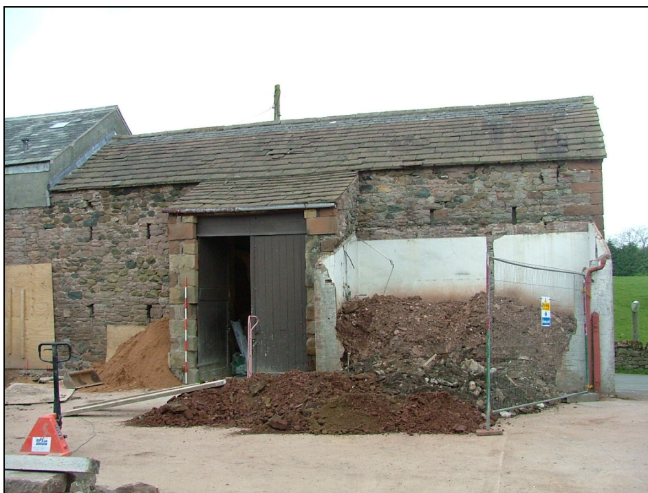
Plate 7 – East elevation of West Barn (Scale = 2m)
