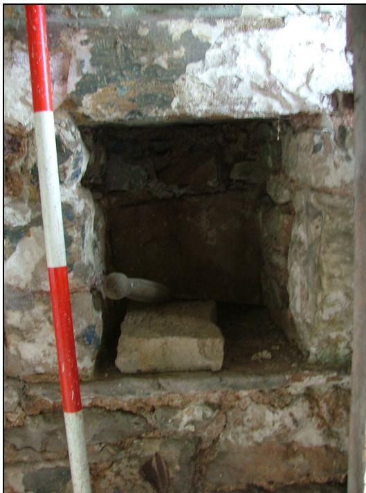
Plate 45 – Niche in the east wall of the privy (Scale is in 20cm graduations)
