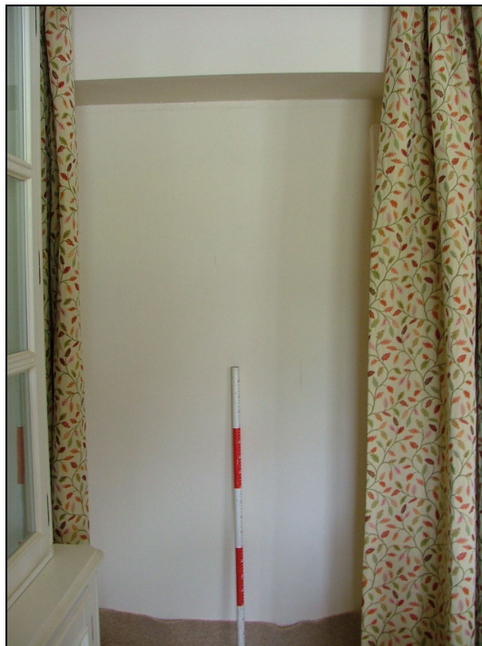
Plate 61 – Blocked doorway in east wall of possible former stable (Scale = 1m)
