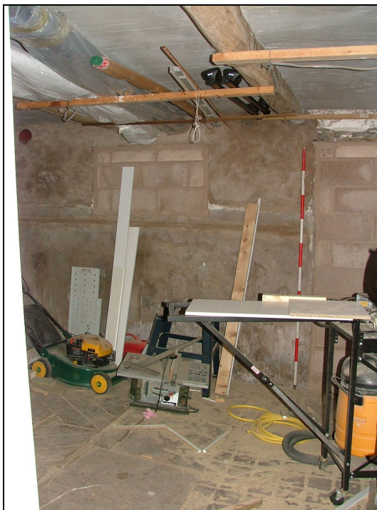
Plate 32 – Blocked window and doorway, east wall of East Byre (Scale = 2m)
