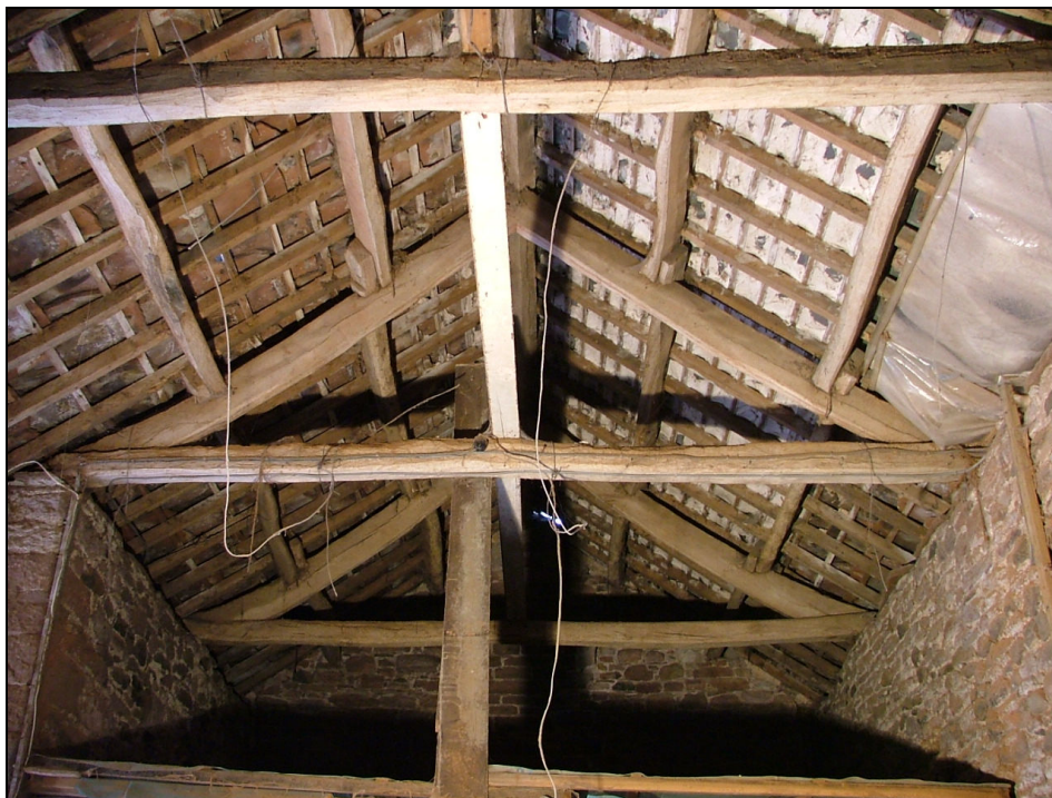
Plate 10 – Detail of roof trusses, interior of West Barn
