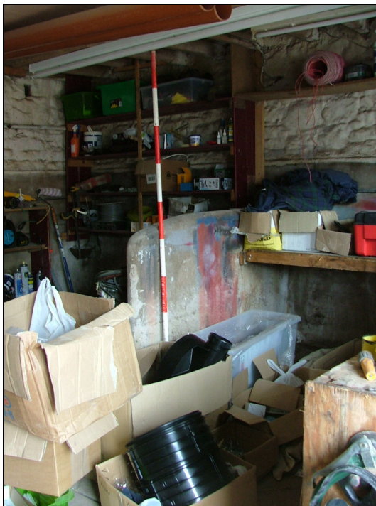
Plate 31 – Concrete stall divider, south end of East Byre (Scale = 2m)
