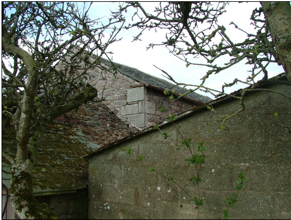
Plate 25 – The faint line of a former roof just visible on the quoin of the south gable, East Byre (the block work shed in the foreground is in separate ownership)
