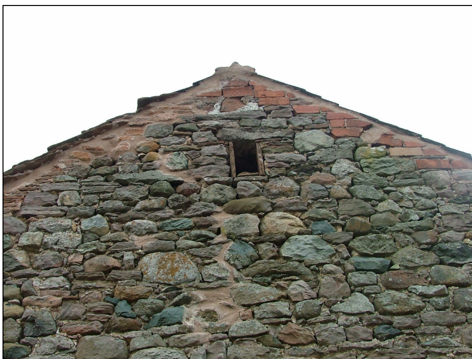
Plate 6 – Detail of owl hole, north elevation of West Barn
