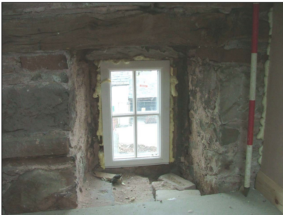
Plate 66 – Window in north gable of house as seen from the attic
