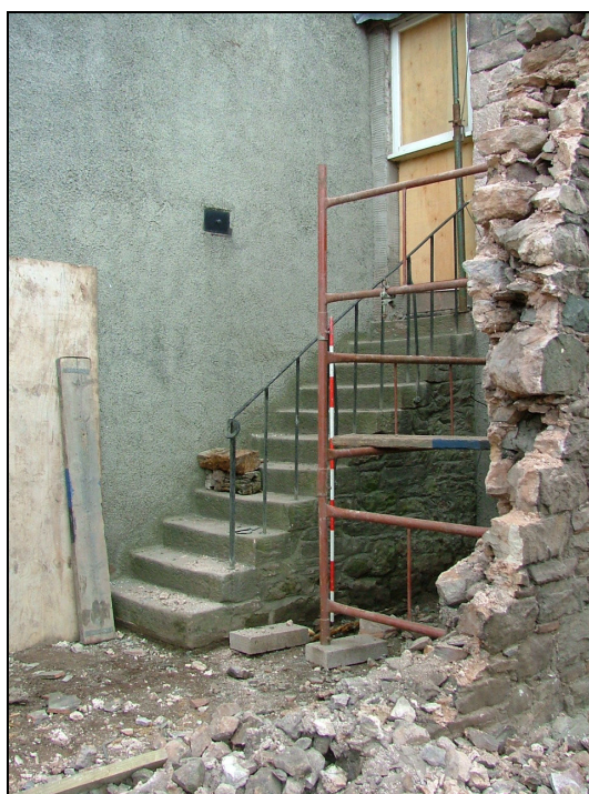
Plate 56 – Detail of stone staircase to possible former granary (Scale = 2m)
