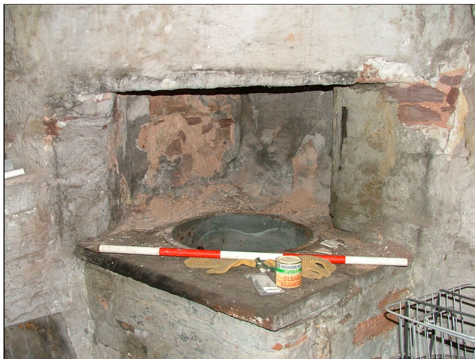
Plate 52 – Detail of metal set-pot set in a stone surround (Scale =1m)
