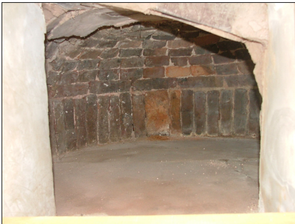
Plate 64 – Interior of the brick-lined bread oven still surviving in the present kitchen of Greystone House
