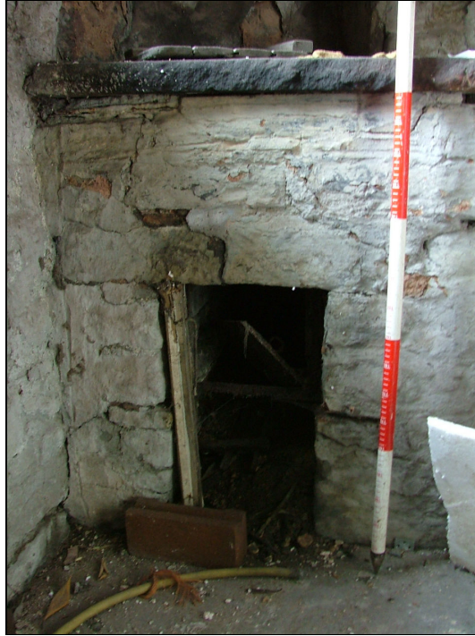
Plate 53 – Hole at base of set-pot for lighting the fire
