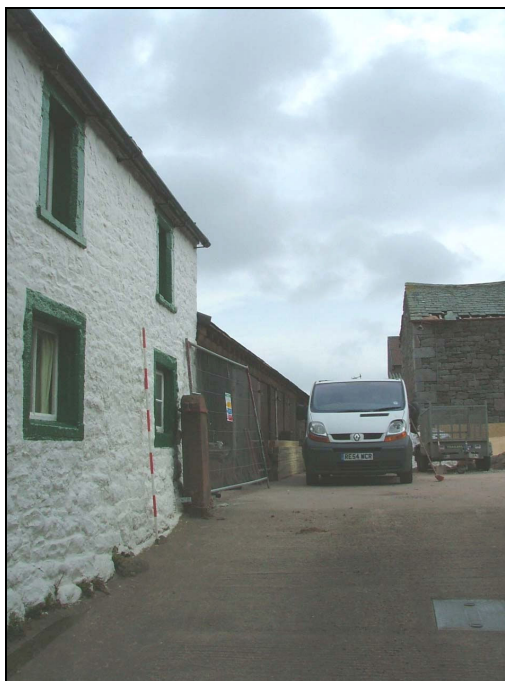
Plate 34 – View looking east from entrance to farmyard showing Chapel Cottage (whitewashed) with the North range beyond
