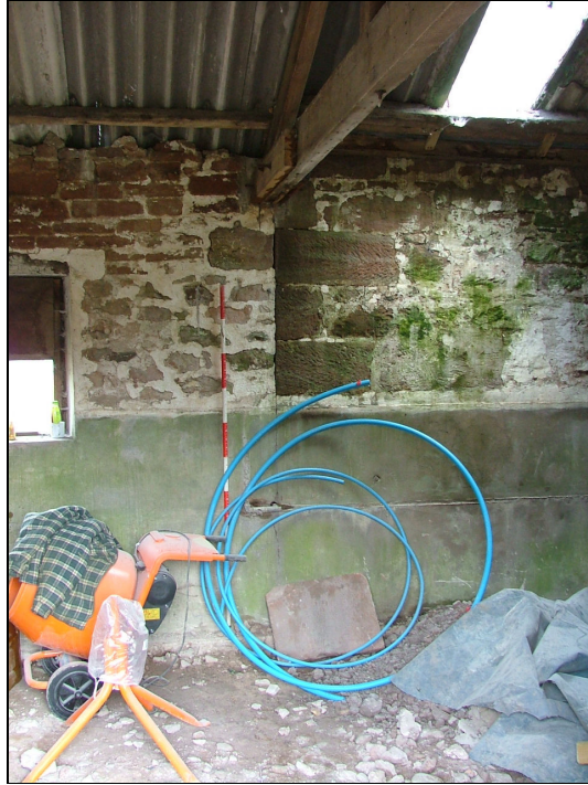
Plate 47 – North wall of South Range showing the quoins of the south gable of the East Byre (Scale = 2m)
