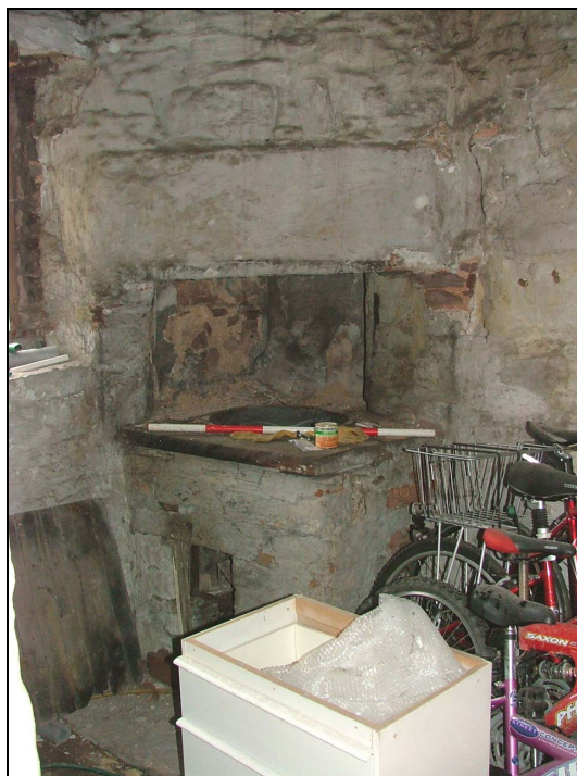
Plate 51 – Stone-built surround for a set-pot, interior of the wash-house (Scale = 1m)
