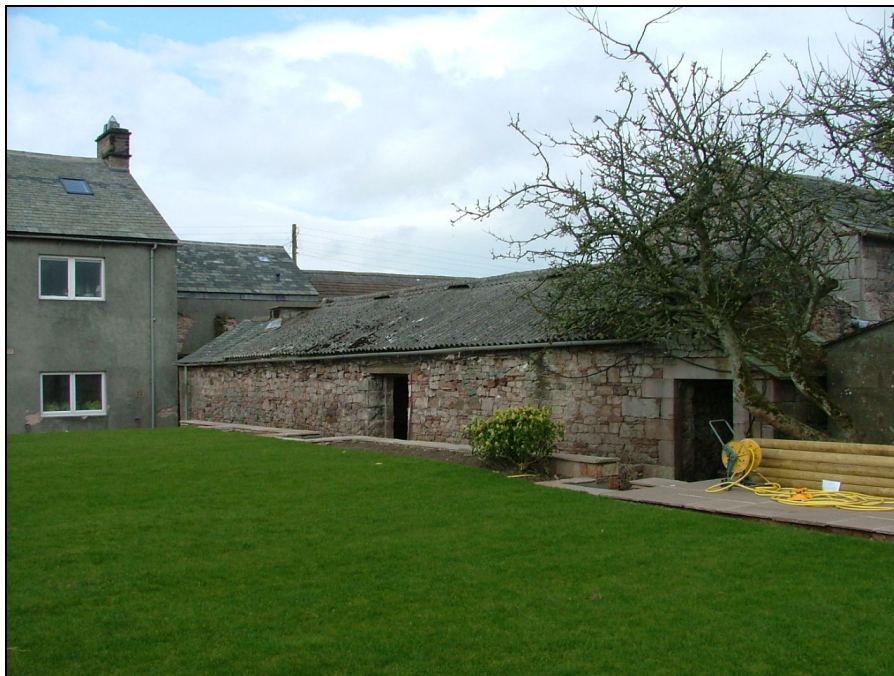
Plate 43 – View looking north-west of the south elevation of the South Range
