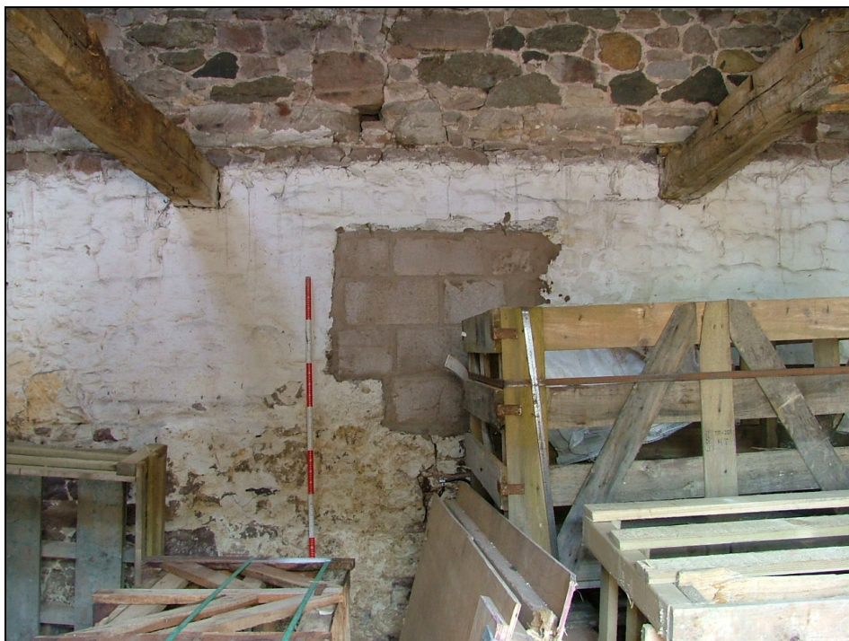
Plate 29 – Blocked window, east wall of East Byre (Scale = 2m)
