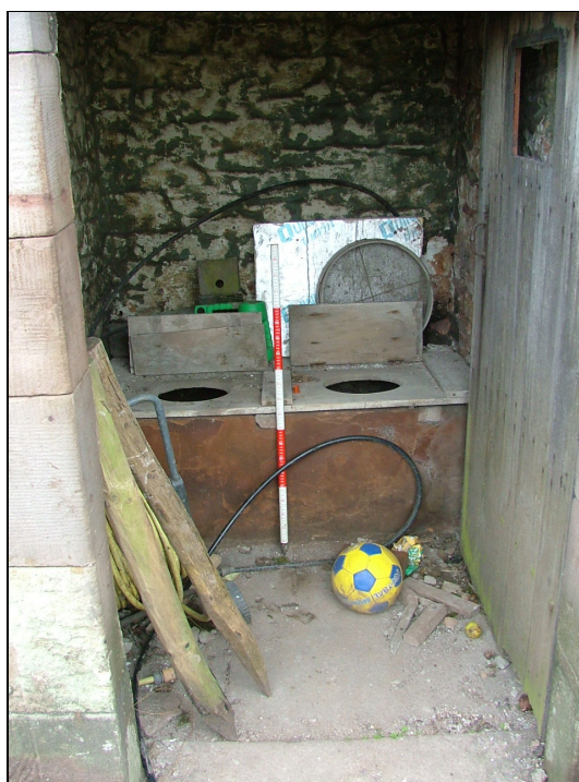
Plate 44 – Privy at east end of the South Range showing two holes with lids (Scale = 1m)
