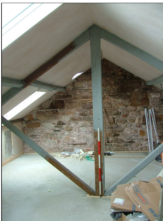
Plate 65 – One of the roof trusses of the house (Scale = 1m)
