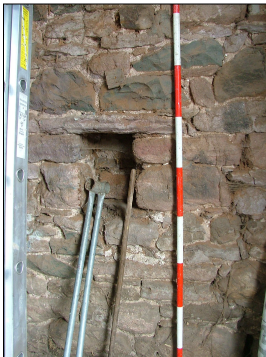
Plate 18 - Niche in projecting porch way, West Barn (Scale is in 20cm graduations)
