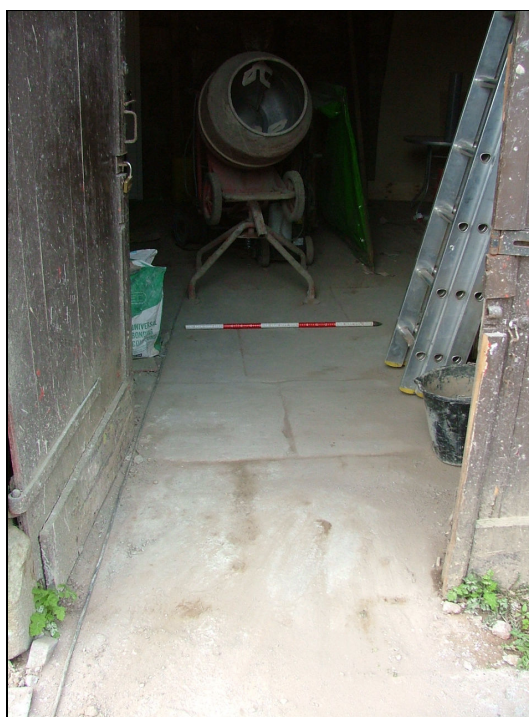
Plate 14 – Detail of sandstone flagged floor, central section of West Barn (Scale = 1m)
