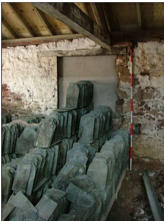
Plate 41 – Possible blocked doorway in north wall of North Range (Scale = 2m)
