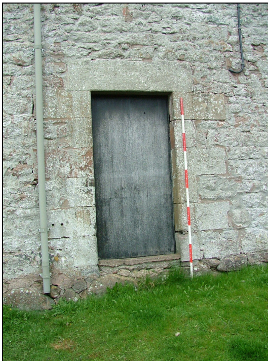
Plate 3 – Doorway, west elevation of West Barn (Scale = 2m)
