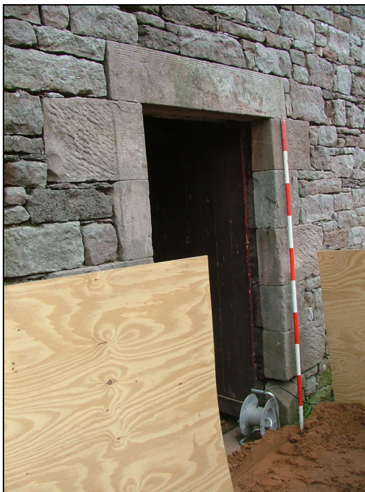
Plate 21 – Detail of north doorway, west elevation of East Byre (Scale = 2m)
