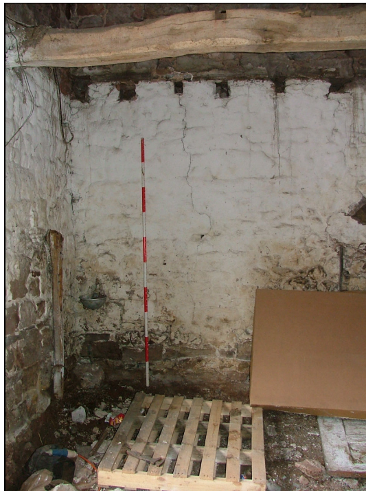
Plate 26 – North internal wall of East Byre showing limewashed walls and redundant joist holes for a former first floor (Scale = 2m)
