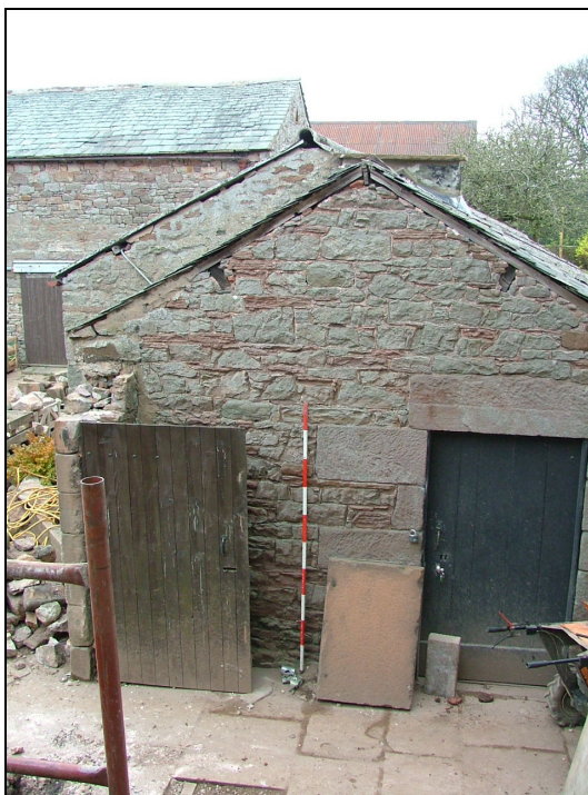
Plate 49 – West gable of wash-house (Scale = 2m)
