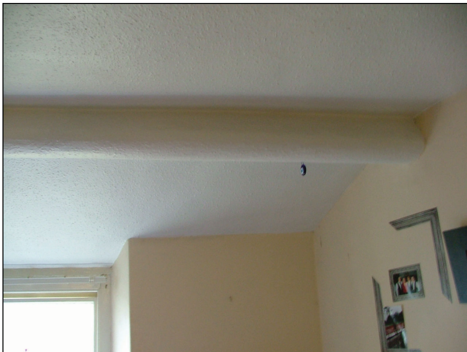
Plate 29 – Covered purlin, second floor of Mill Cottage
