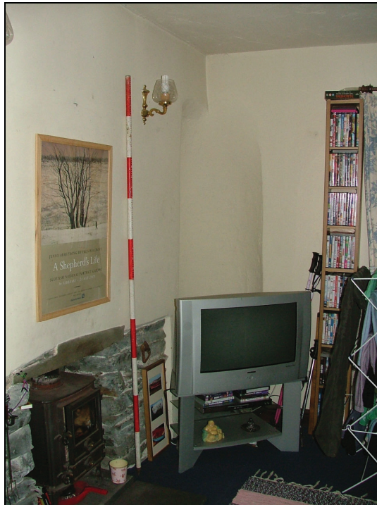
Plate 39 – Circular recess in north-east wall of small cottage, possible former set-pot? (Scale =2m)
