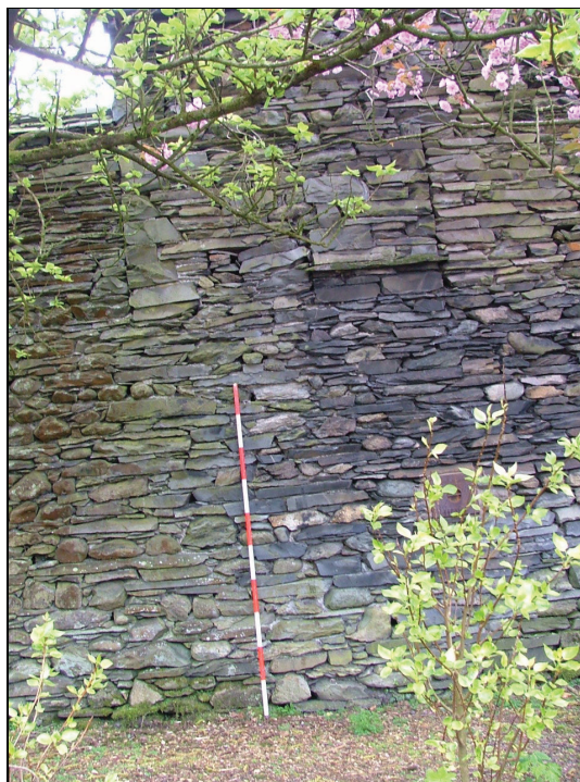
Plate 36 – Blocked window, north elevation of small cottage (Scale = 2m)
