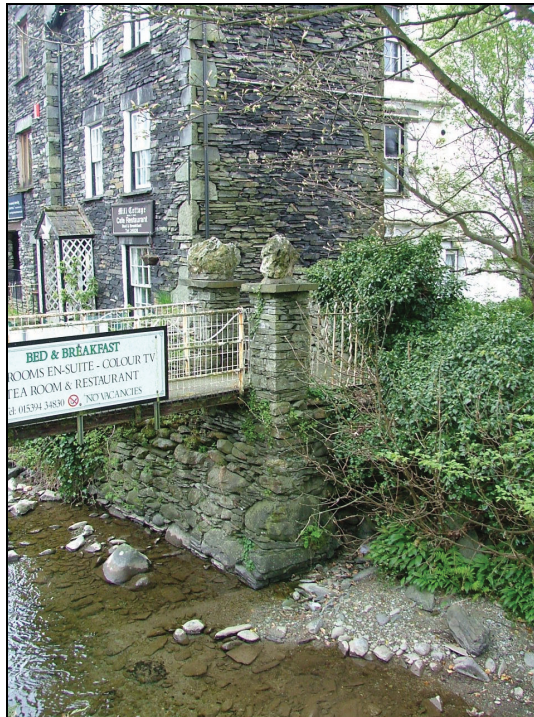
Plate 9 – Metal footbridge to Mill Cottage, with a square aperture at its base possibly relating to the former mill race
