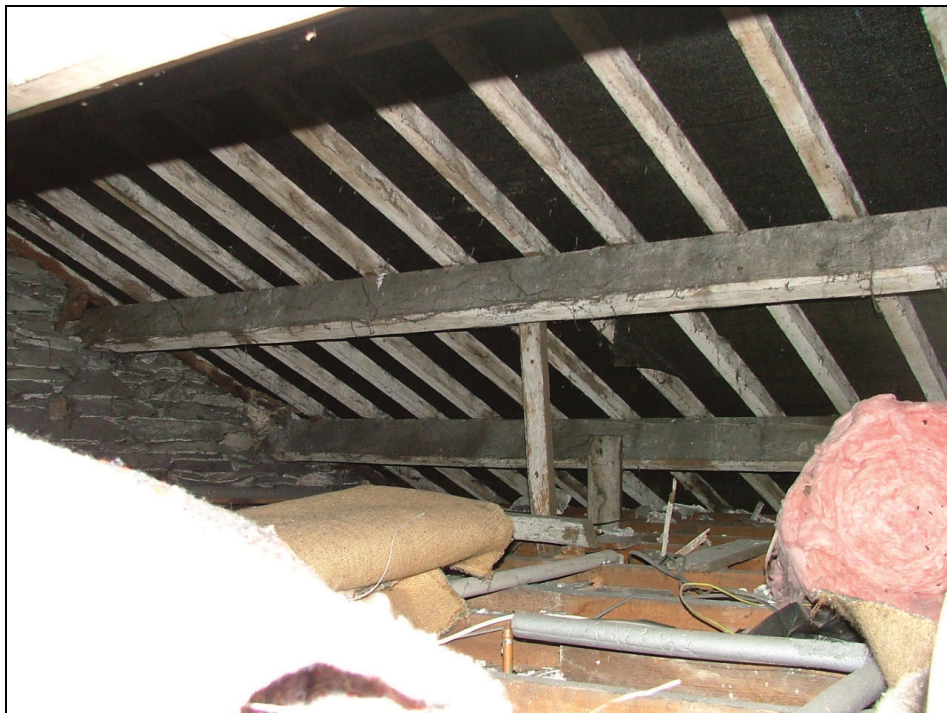
Plate 31 – Detail of part of the roof structure
