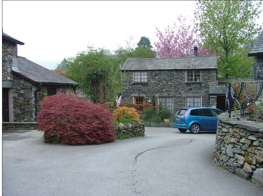
Plate 13 – View looking north showing the small cottage, landscaping and hard standing to the west of Mill Cottage
