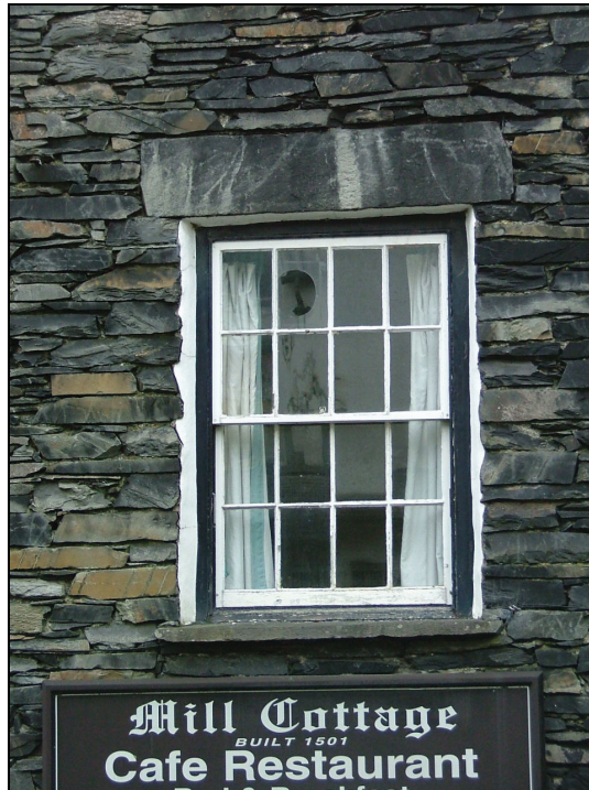
Plate 16 – Detail of first floor sash window, east elevation of Mill Cottage
