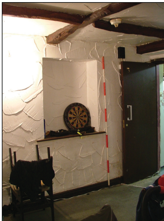
Plate 27 – Possible former doorway in east wall (Scale = 2m)
