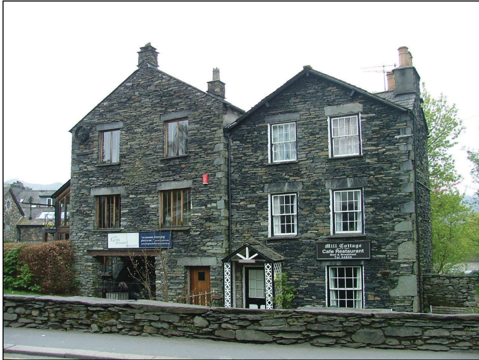
Plate 1 – East elevations of Mill Cottage and the Glass House Restaurant (former woollen mill)
