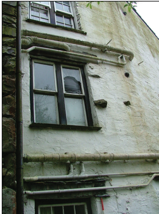
Plate 22 – Detail of first floor window, north elevation
