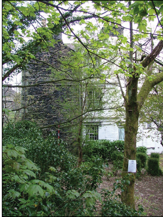
Plate 18 – North elevation of Mill Cottage
