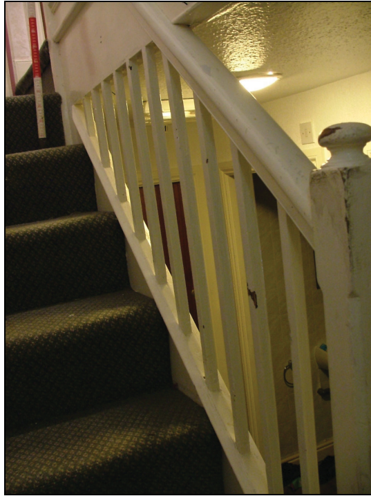
Plate 28 – Detail of staircase, interior of Mill Cottage
