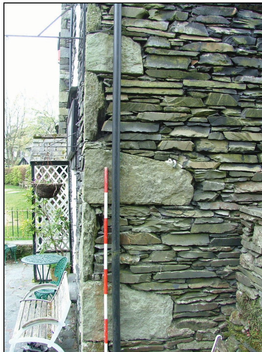
Plate 17 – Detail of quoins at the corner of the north and east elevations (Scale is in 20cm graduations)
