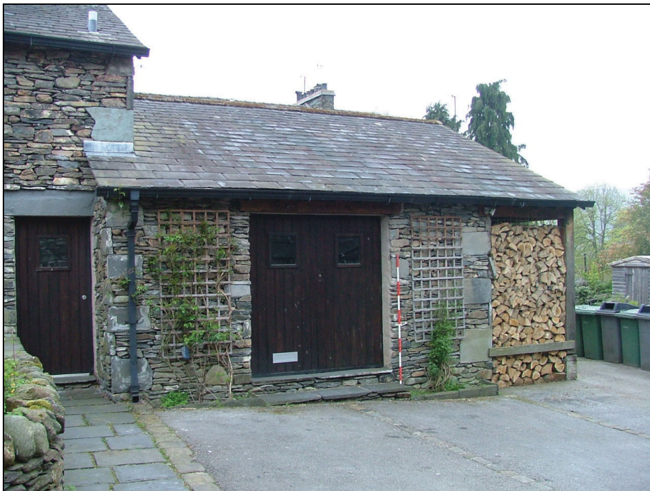
Plate 43 - East elevation of store to west of Mill Cottage and the Glass House Restaurant (Scale = 2m)
