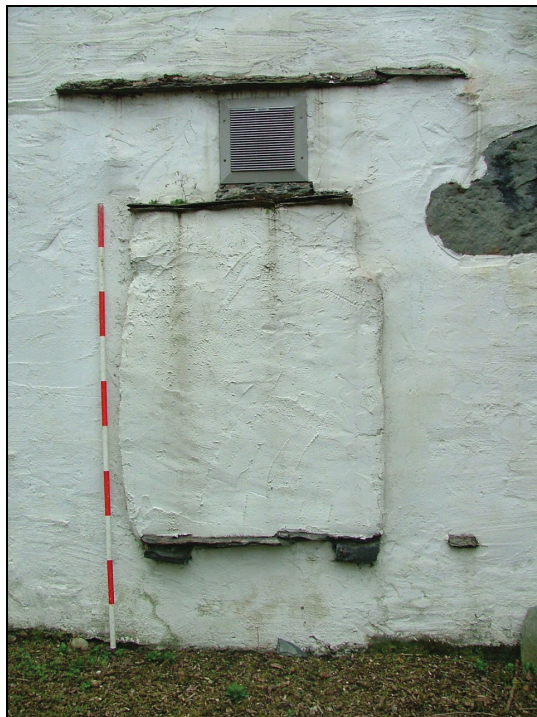
Plate 21 – Possible blocked window or chimney, north elevation (Scale = 2m)
