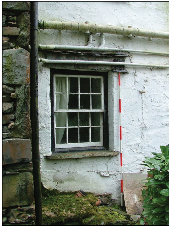
Plate 20 – Detail of ground floor sash window, north elevation (Scale = 2m)
