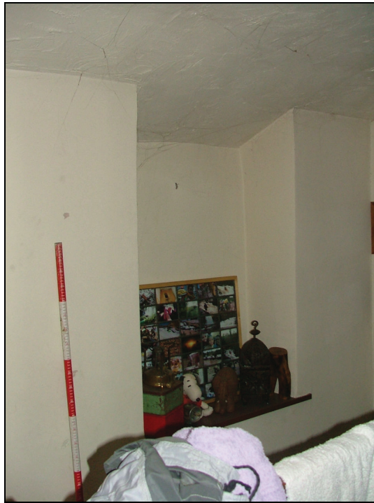
Plate 41 – Former window at first floor level, small cottage
