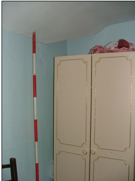
Plate 30 – Sloping ceiling, second floor of Mill Cottage (Scale = 2m)
