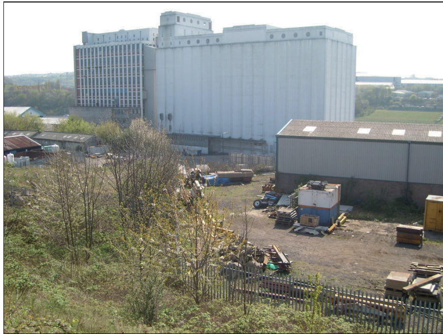
Plate 10 - View looking south-east from the former railway line showing the east side of the site with Spillers Mill in the background (Courtesy of Lewis Ray)
