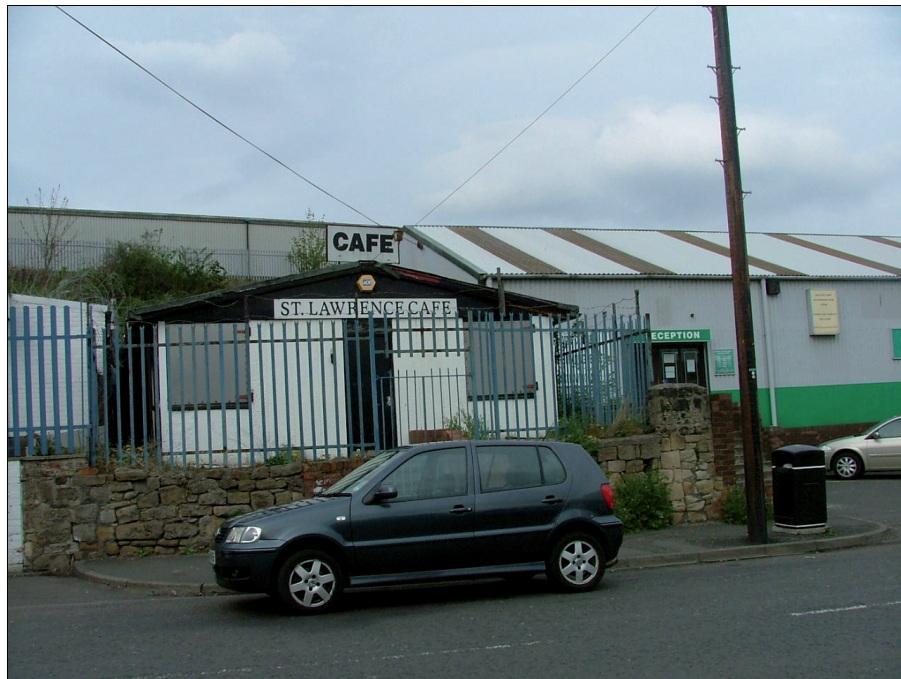
Plate 11 - View looking north from St Lawrence Road showing buildings below the former Kesson Lifting site
