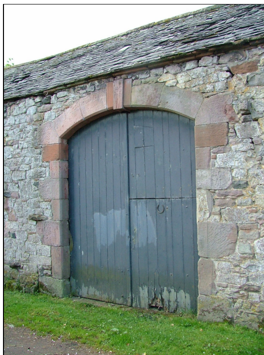
Plate 48 – Doorway with keystone containing the inscription 'P G 1751', redundant farm building opposite The Mains
