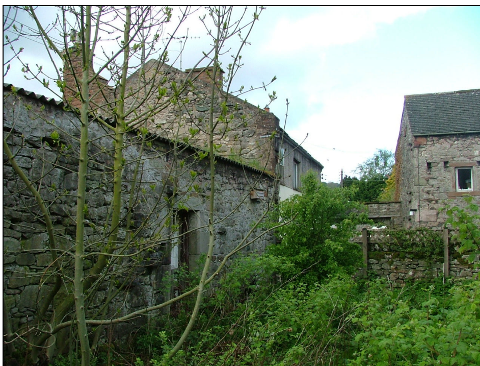
Plate 31 – View looking west along the north elevation of Building 3
