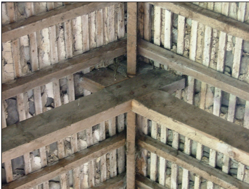
Plate 10 – Detail of apex of principal rafter, Building 1
