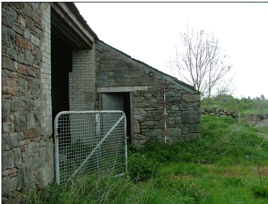
Plate 3 – South-west elevation of outshut against Building 1 showing possible inserted door (Scale = 2m)
