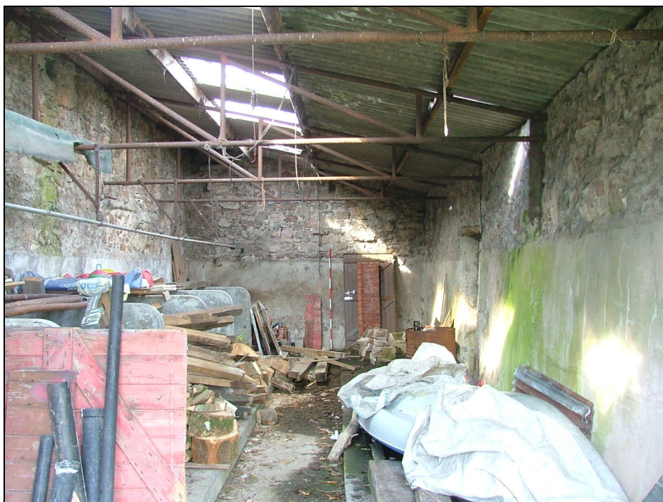
Plate 35 – View looking west of the interior of Building 3 (Scale = 2m)
