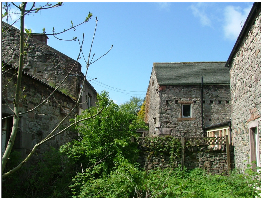
Plate 45 – View looking west to the north of Building 3 showing the former barn adjoining Midtown, with the upper floor containing a row of possible nesting boxes for birds
