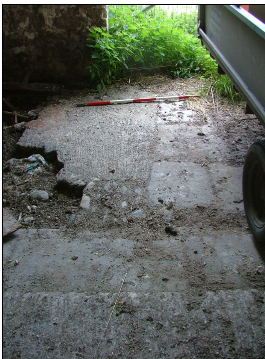
Plate 13 – Remains of the stone flagged floor, central section of Building 1 (Scale = 1m)
