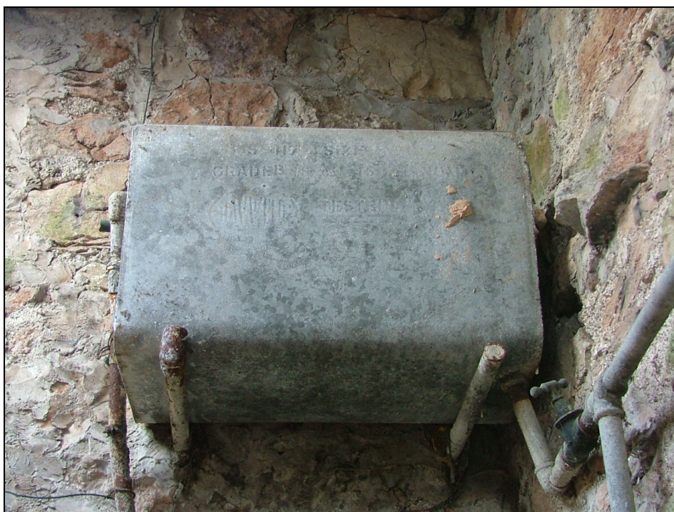
Plate 37 – Water tank on the east wall of the byre, Building 3
