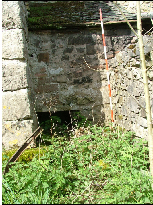
Plate 23 – Hole at the base of the privy wall (Scale = 2m)
