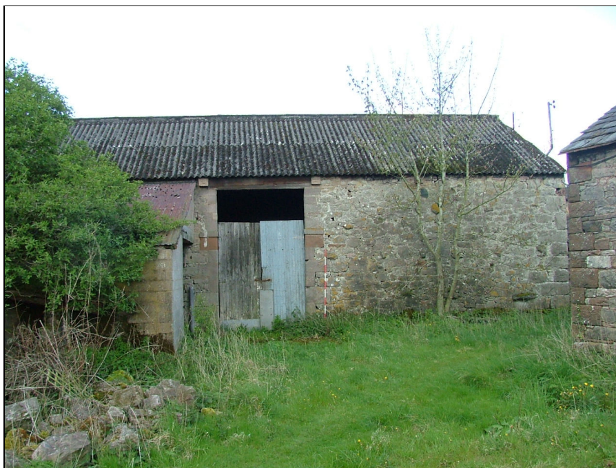
Plate 16 – East elevation of Building 2 (Scale = 2m)
