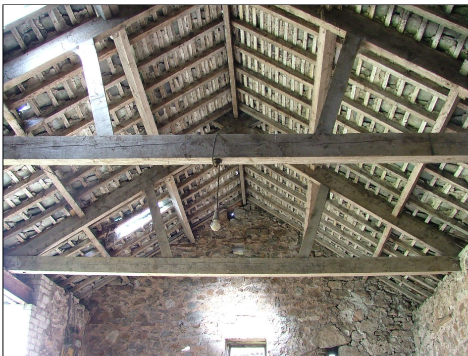
Plate 9 – Detail of roof structure, Building 1
