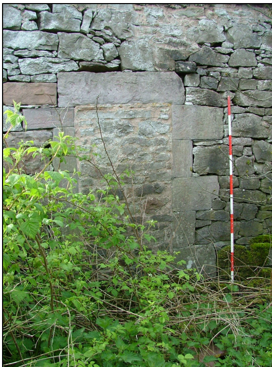
Plate 33 – Blocked doorway in north elevation of Building 3 (Scale = 2m)
