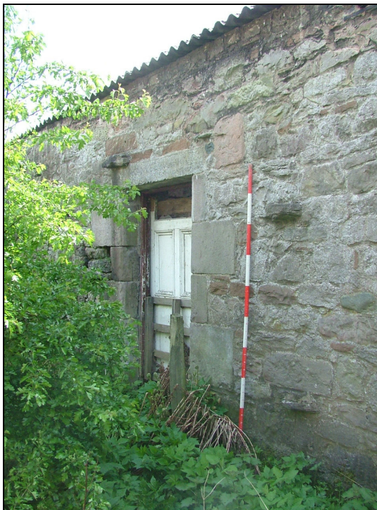
Plate 32 – Doorway in north elevation of Building 3 (Scale = 2m)
