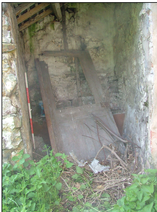
Plate 22 – View into the privy showing the sandstone support for the seat partly hidden by the door, and the limewashed walls (Scale = 1m)
