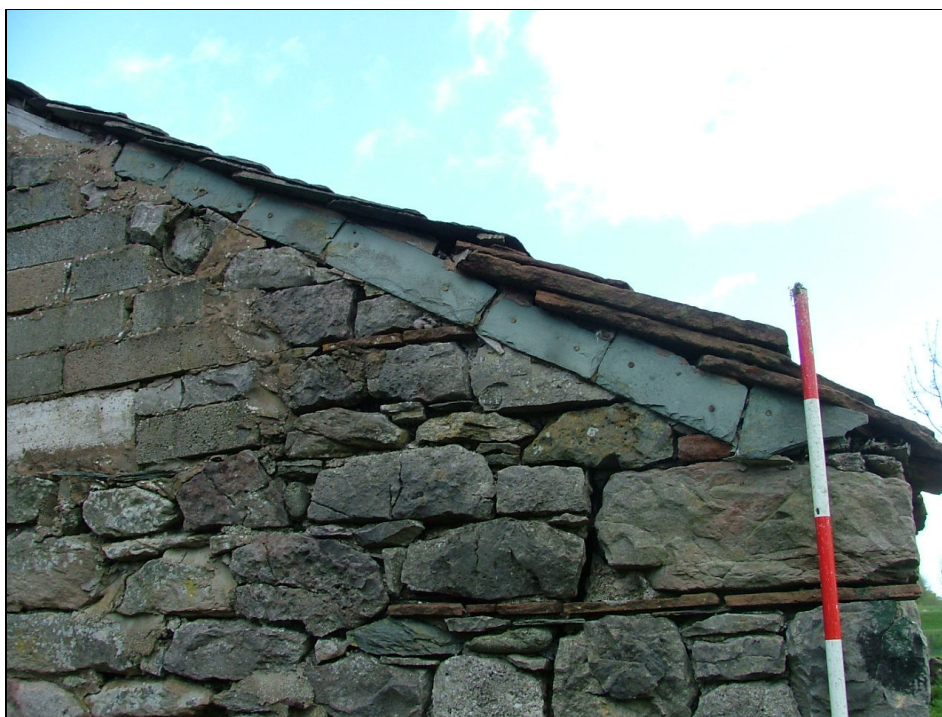
Plate 4 – Detail of slate nailed to timber below roof, outshut against Building 1
