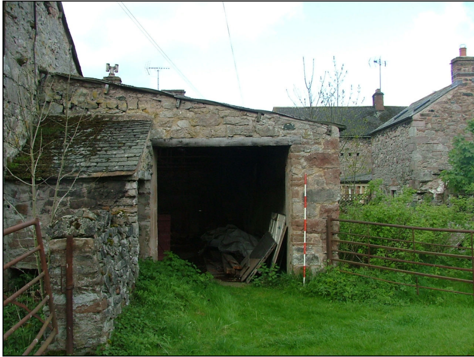
Plate 34 – East elevation of Building 3 (Scale = 2m)
