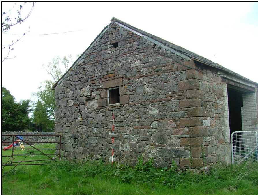
Plate 5 – South-west elevation of Building 1 (Scale = 2m)
