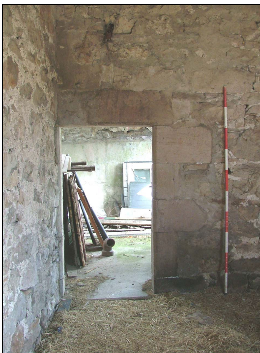
Plate 26 – Doorway in north gable of Building 2 which has chamfered edges to the jambs and lintel suggesting Building 3 was in existence prior to Building 2 (Scale = 2m)
