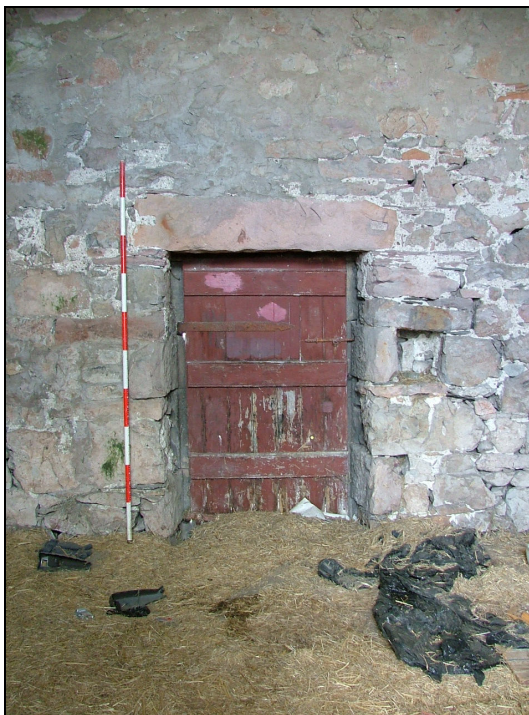
Plate 27 – Doorway in west elevation of Building 2, with a niche for a candle or oil lamp to the right-hand side (Scale = 2m)
