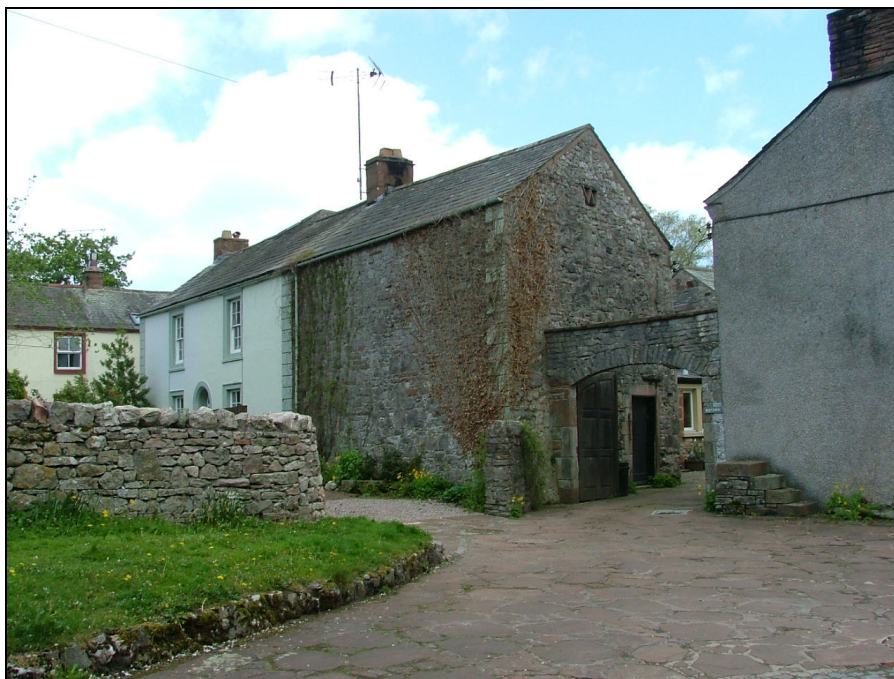
Plate 41 – West elevation of Midtown and adjoining barn
