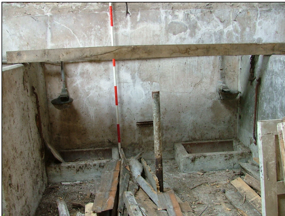
Plate 36 – Detail of one of the double stalls showing metal stanchion, water troughs and feeding troughs (Scale is in 20cm graduations)
