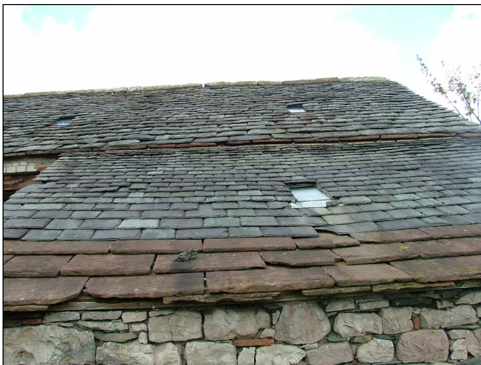
Plate 2 – Detail of the south facing roofs of Building 1 and the outshut
