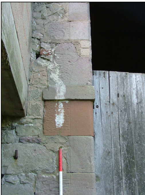
Plate 17 – Detail of the masonry blocks which make up part of the left-hand jamb with one block showing evidence for a former arched head, Building 2
