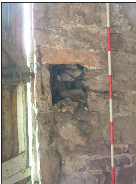
Plate 28 – Niche in east wall, Building 2 (Scale is in 20cm graduations)
