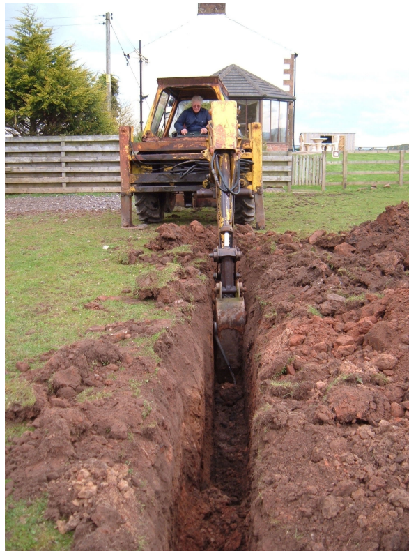
Plate 1: Excavation of north eastern end of service trench
