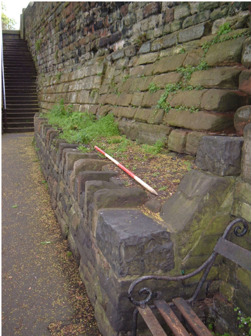
Plate 1: View northwest of Trench 1 location (pre-ex) and Victorian retaining wall (105)
