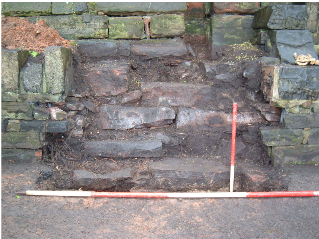
Plate 3: Southwest facing elevation of wall foundations (106) Trench 1
