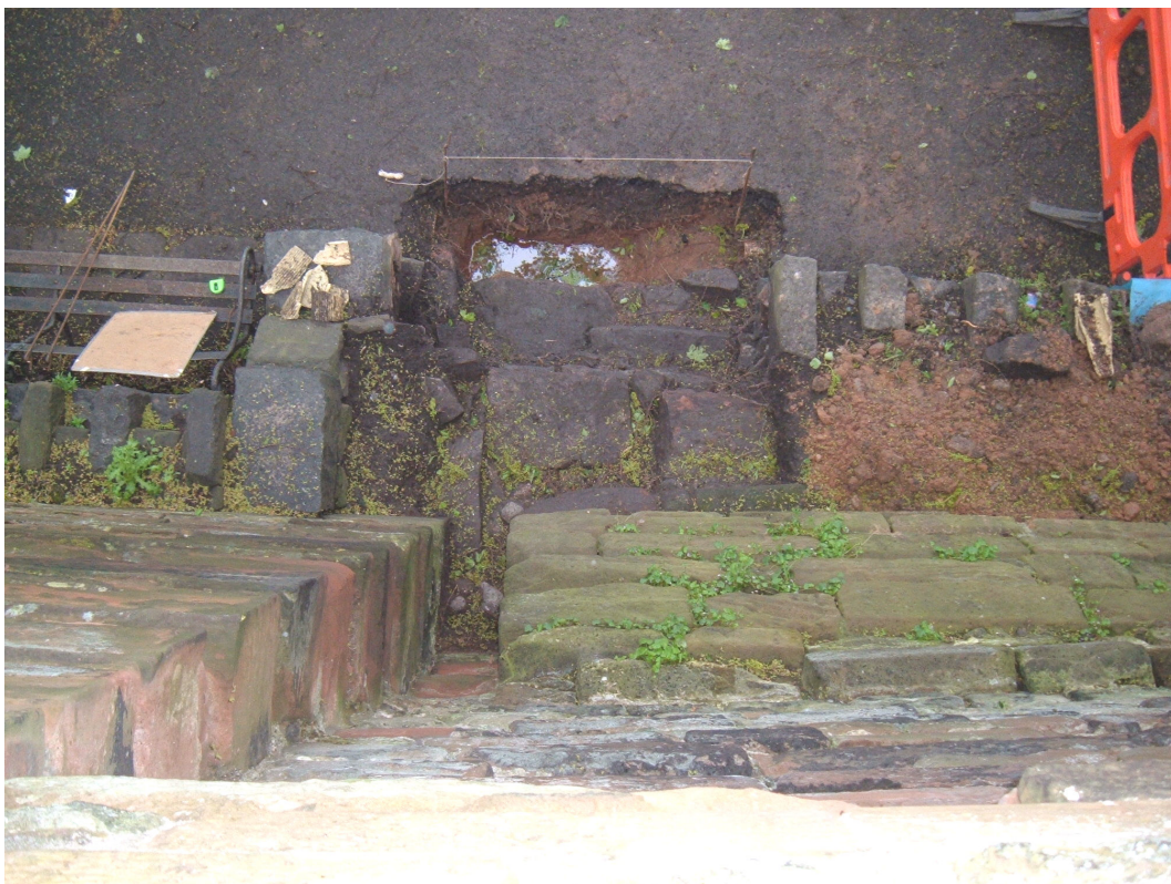
Plate 4: Plan view of Trench 1 (note the varied wall structure in foreground)
