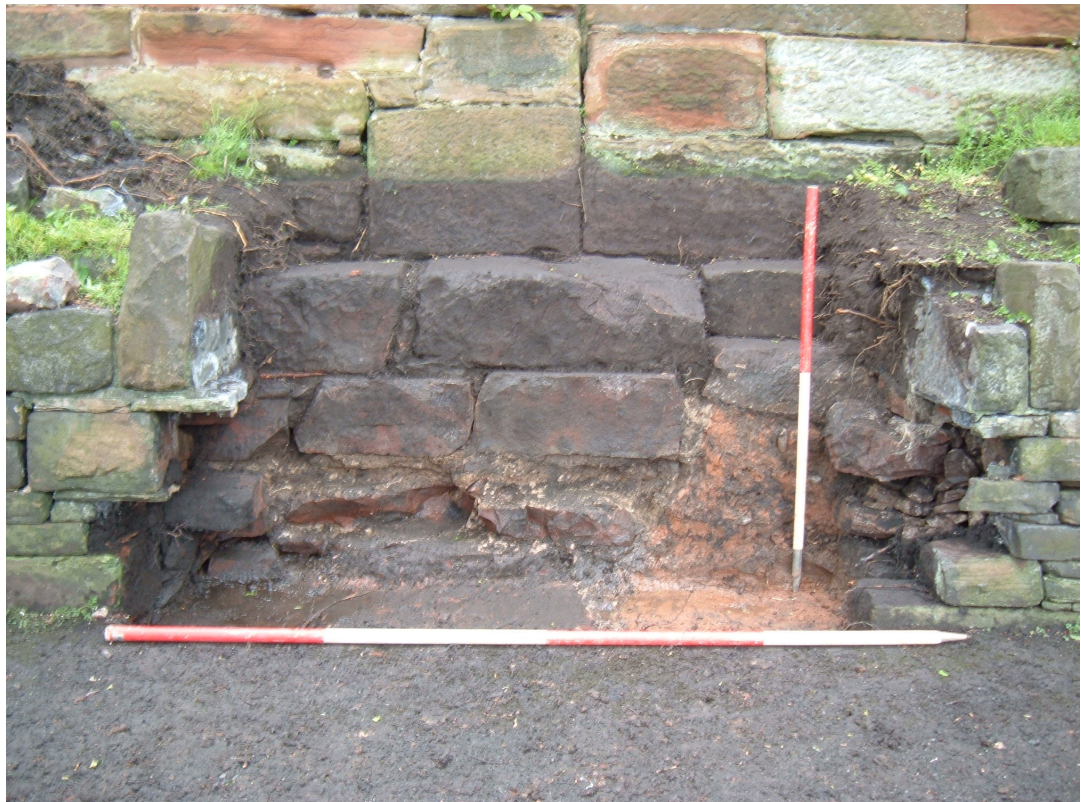
Plate 7: Southwest-facing section of Trench 2 showing foundations (106) cut into the natural ground (101)
