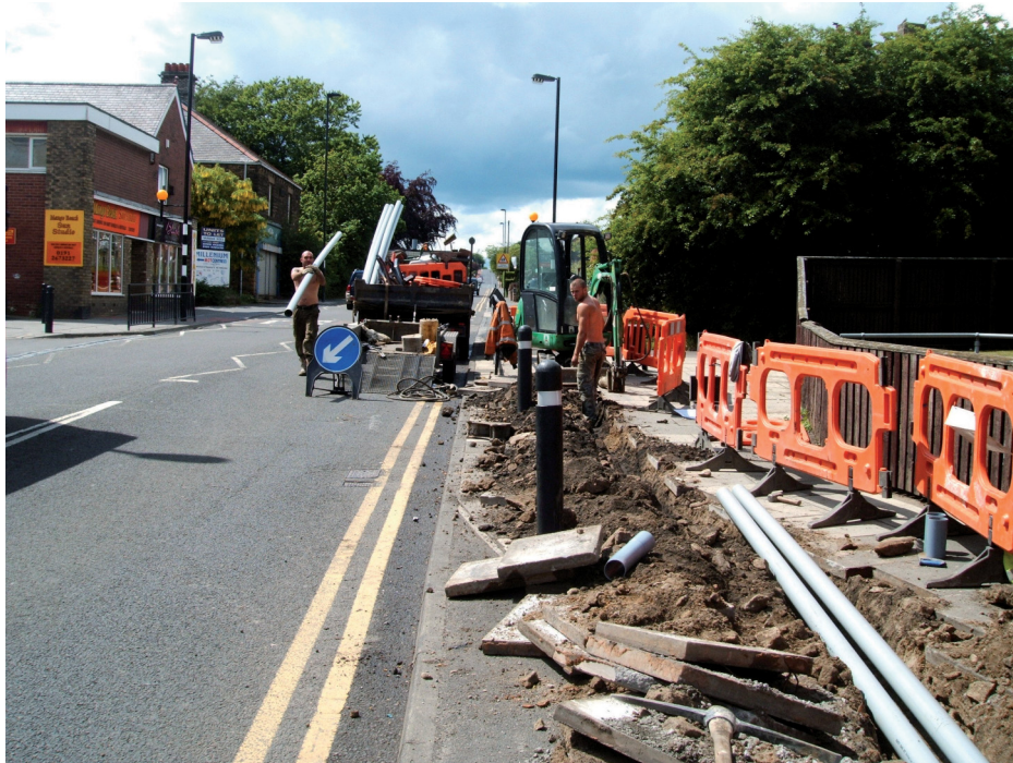
Plate 1: View of trench nearing completion looking east.
