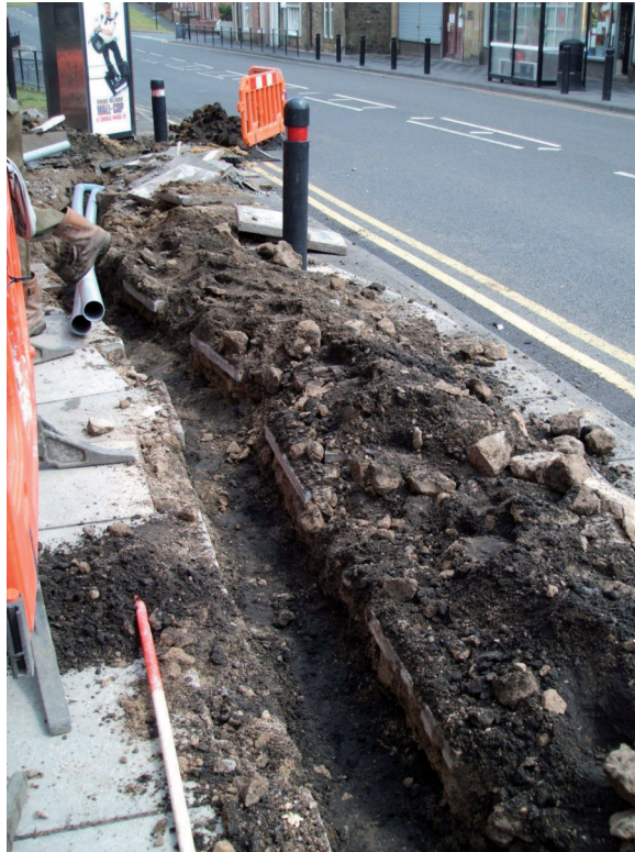
Plate 4: View of deeper west end of trench, looking to the west.
