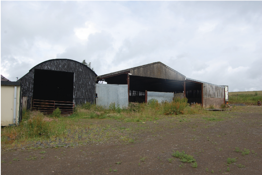
Plate 15: Modern open fronted, steel-framed barn
