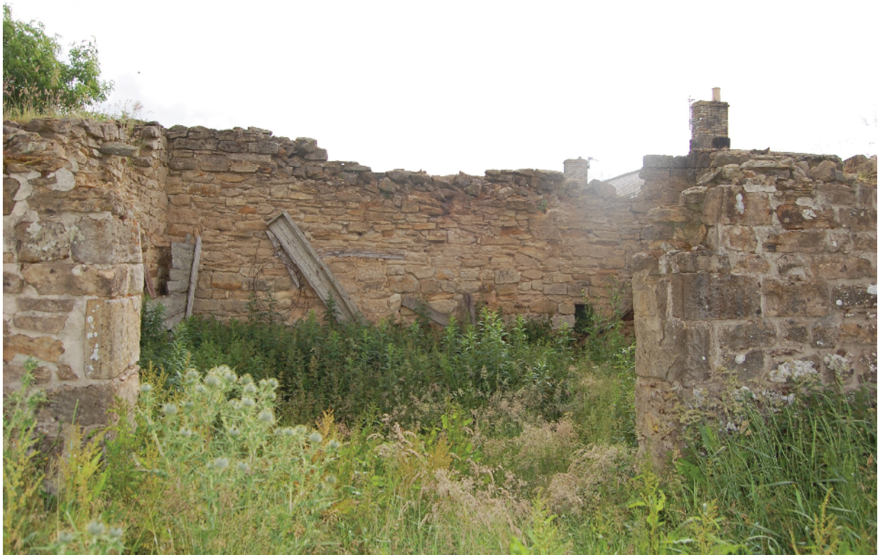
Plate 10: The interior of the outbuilding, looking east
