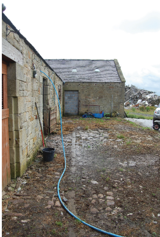
Plate 14: Cobbled area to the front of the stables, looking east
