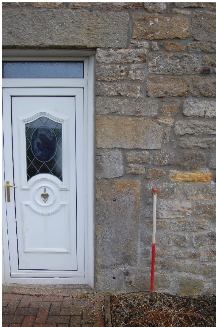
Plate 6: 'T.H' etched into the sandstone blocks to the right of the front door of the dwelling house
