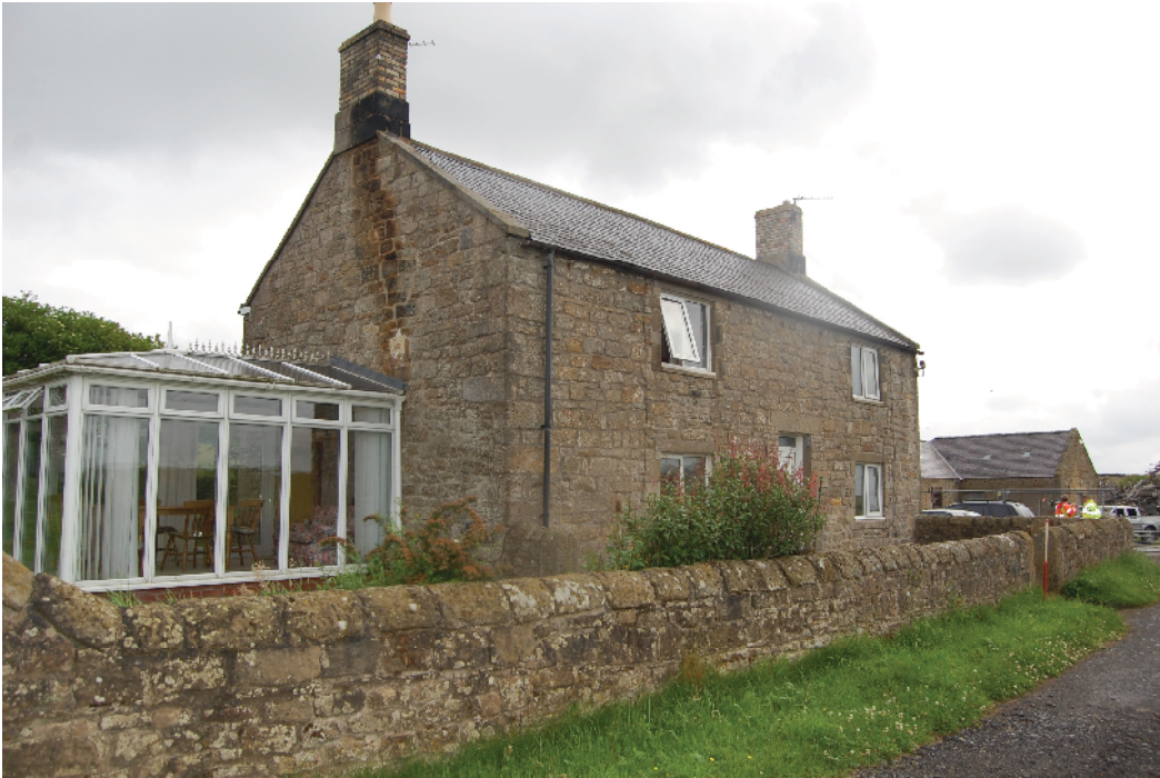
Plate 4: Main dwelling house at Waterfalls Farm, looking northeast
