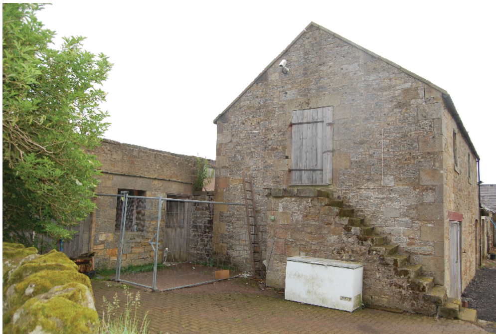
Plate 11: Sandstone granary with cartshed to the rear, located to the east of the main dwelling house, looking east
