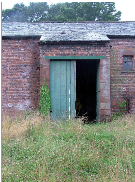
Plate 4: Large doorway in east elevation of Building 1 (Scale = 2m)
