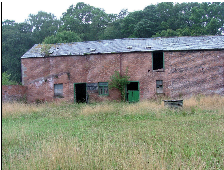
Plate 9: East elevation of Building 2, Range A
