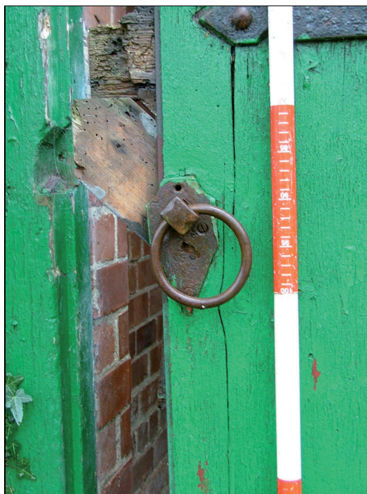
Plate 12: Detail of door handle, Building 2
