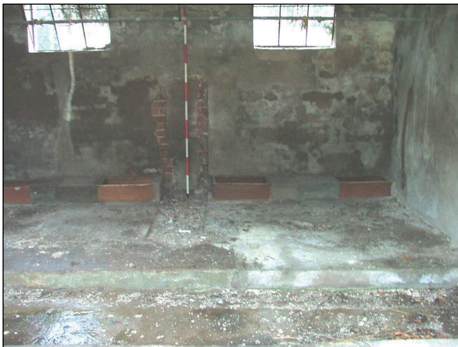
Plate 48: Interior of small byre, Building 3 (Scale = 2m)
