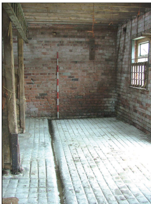
Plate 33: Concrete floor and drainage channel, stable in Building 2 (Scale = 2m)
