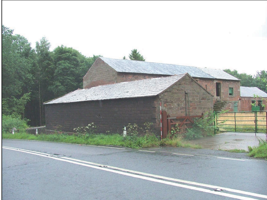
Plate 64: North and west elevations of Building 5 (Scale = 2m)
