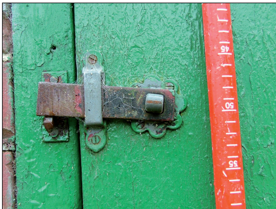
Plate 13: Detail of door latch, Building 2
