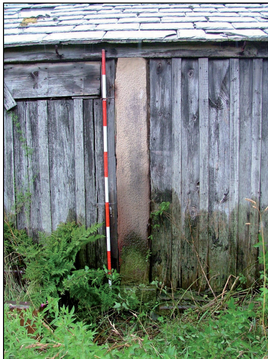
Plate 62: Detail of sandstone pillar, south elevation of Building 5 (Scale = 2m)
