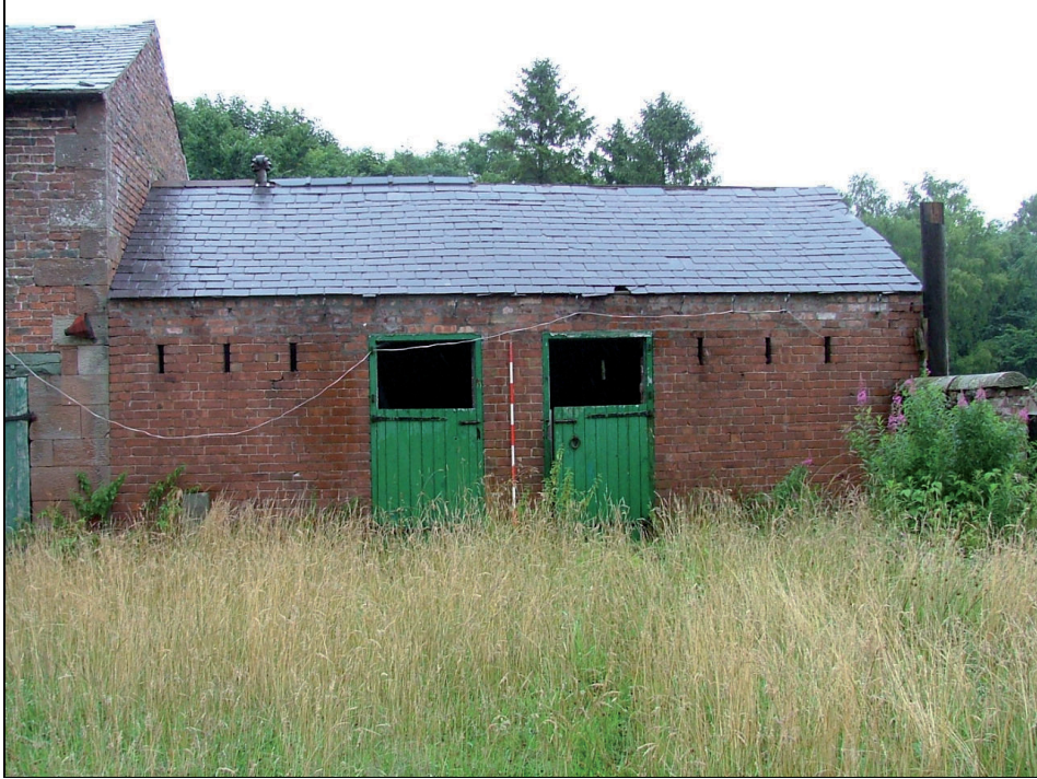
Plate 46: West elevation of Building 4 (Scale = 2m)
