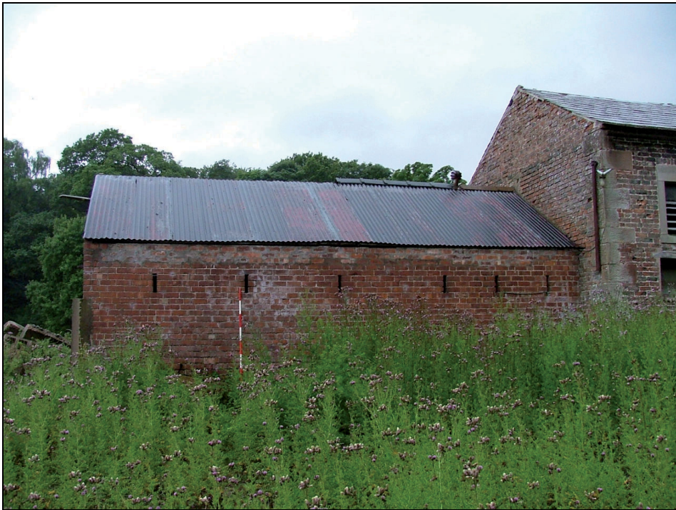
Plate 47: East elevation of Building 4 (Scale = 2m)
