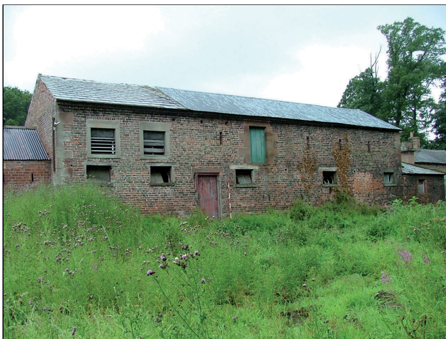
Plate 43: East elevation of Building 3
