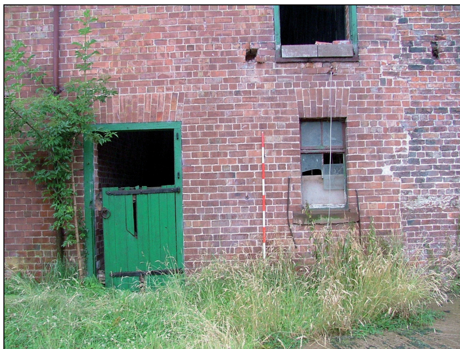
Plate 11: Detail of doorway and window with vertical brickwork for the heads, east elevation of Building 2 (Scale = 2m)
