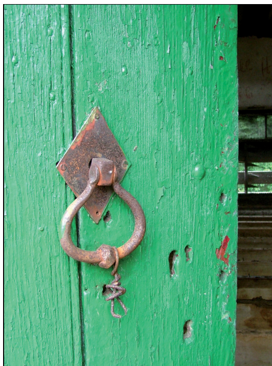
Plate 54: Detail of door handle to granary, Building 3
