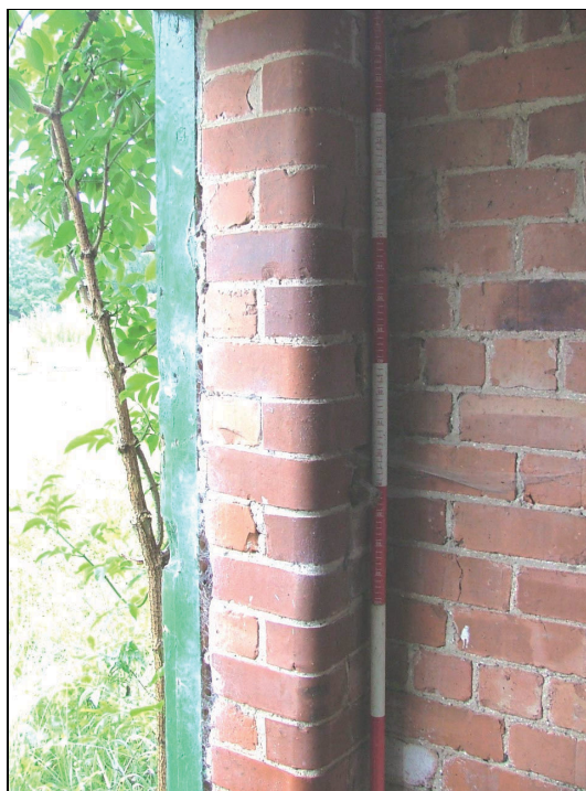
Plate 30: Detail of curved edges to the brickwork, loose box, Building 2
