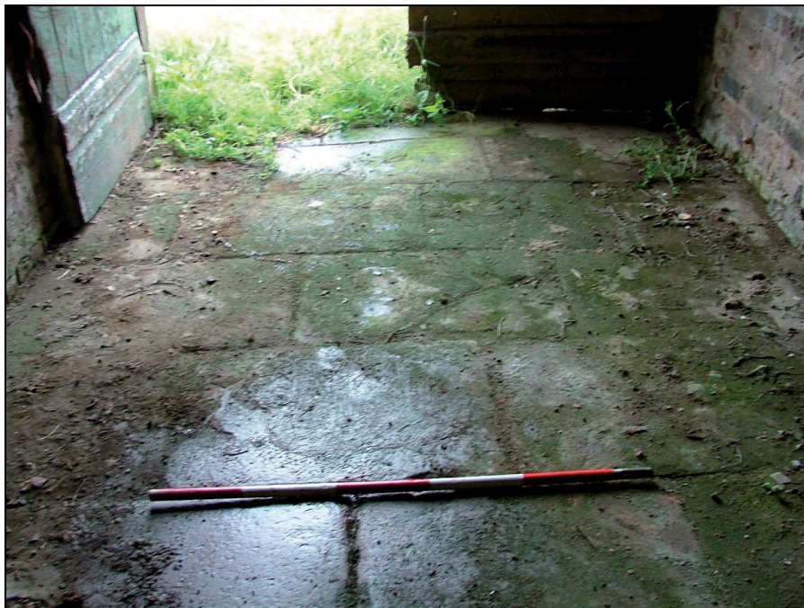
Plate 24: Detail of sandstone flagged floor, Building 1 (Scale = 1m)
