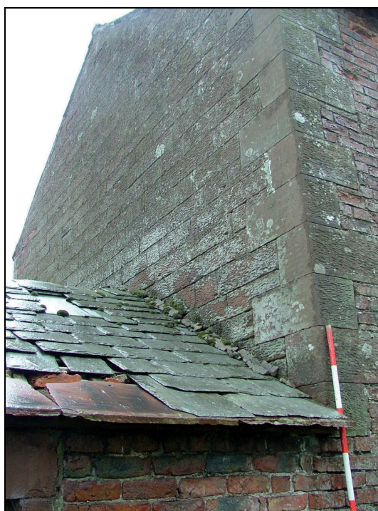
Plate 3: North gable of Range A (Building 1) showing coursed masonry compared to the brickwork of the rest of the building
