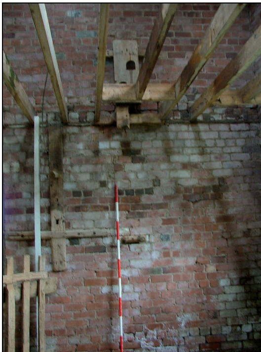
Plate 34: Remains of a Jacobs ladder, east wall of stable, Building 2
