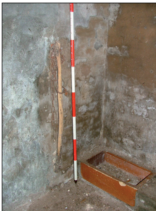
Plate 49: Detail of wooden tethering bar and ceramic feeding trough, small byre in Building 3 (Scale is in 20cm graduations)
