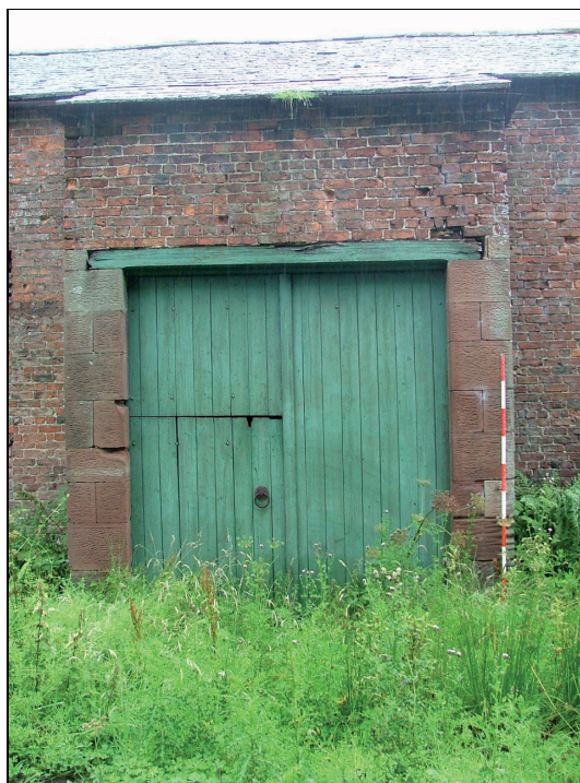
Plate 8: Large doorway in west elevation of Building 1 (Scale = 2m)
