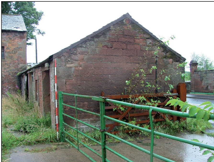
Plate 68: East gable of Building 6 (Scale = 2m)
