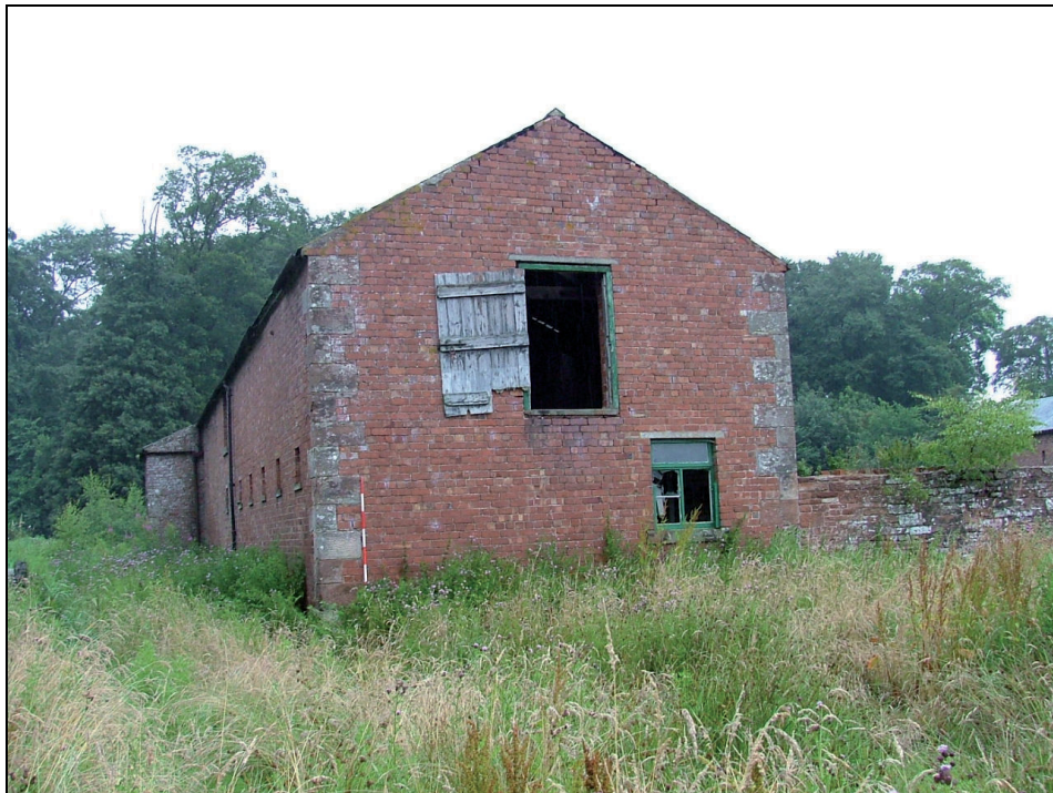
Plate 17: South gable of Building 2 (Scale = 2m)
