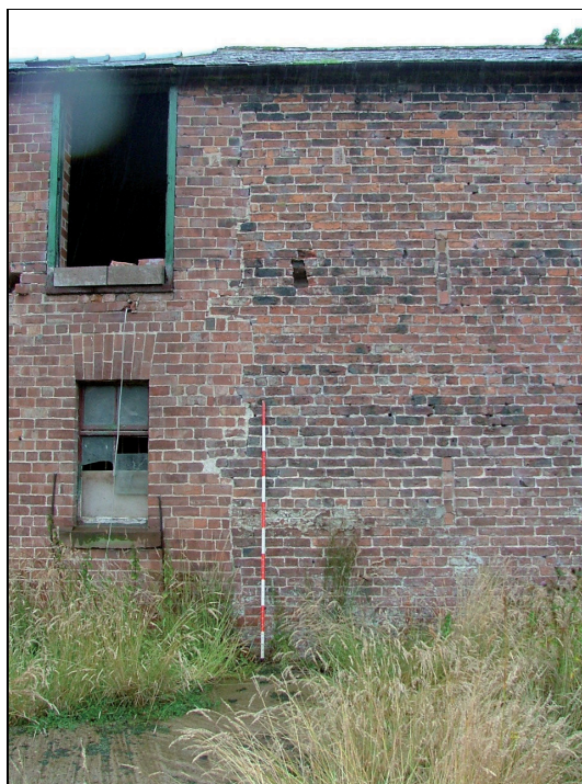
Plate 10: East elevation of Range A showing vertical construction break (Scale = 2m)
