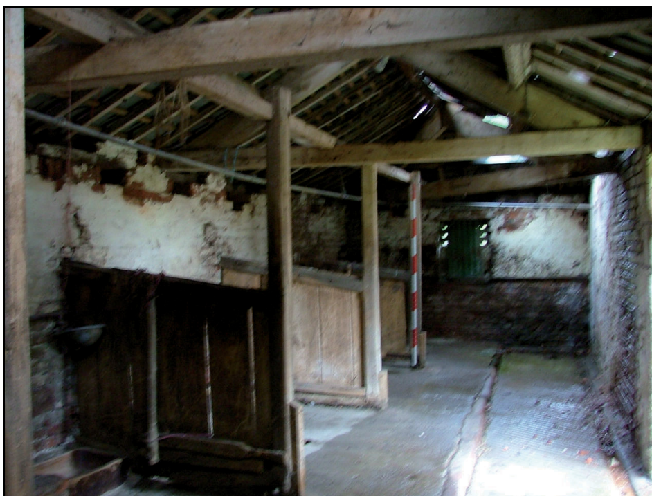
Plate 71: View looking east of the interior of Building 5 (Scale = 2m)
