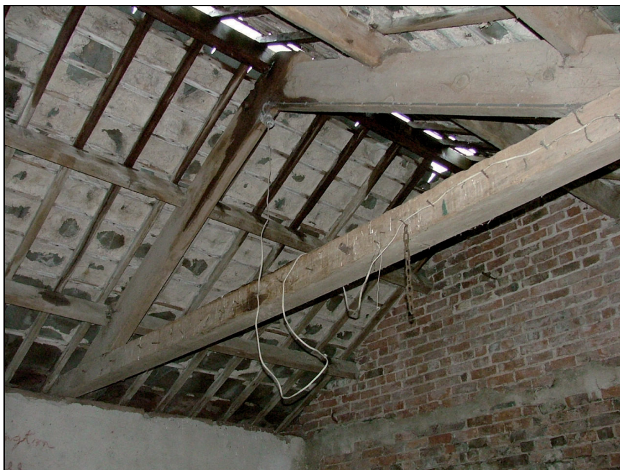
Plate 58: Roof truss and 'torching' to underside of roof, granary, Building 3
