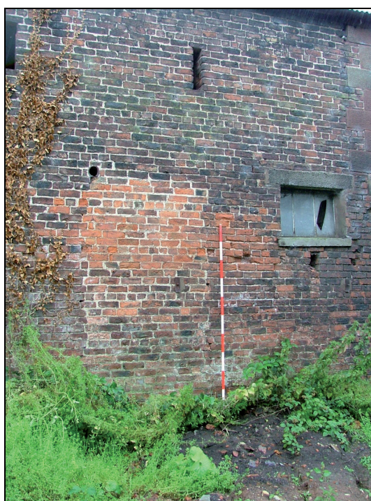
Plate 45: Blocked doorway, north end of east elevation, Building 3 (Scale = 2m)
