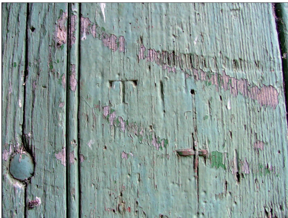
Plate 22: Initials 'T' and possible 'Y', door to barn, Building 1
