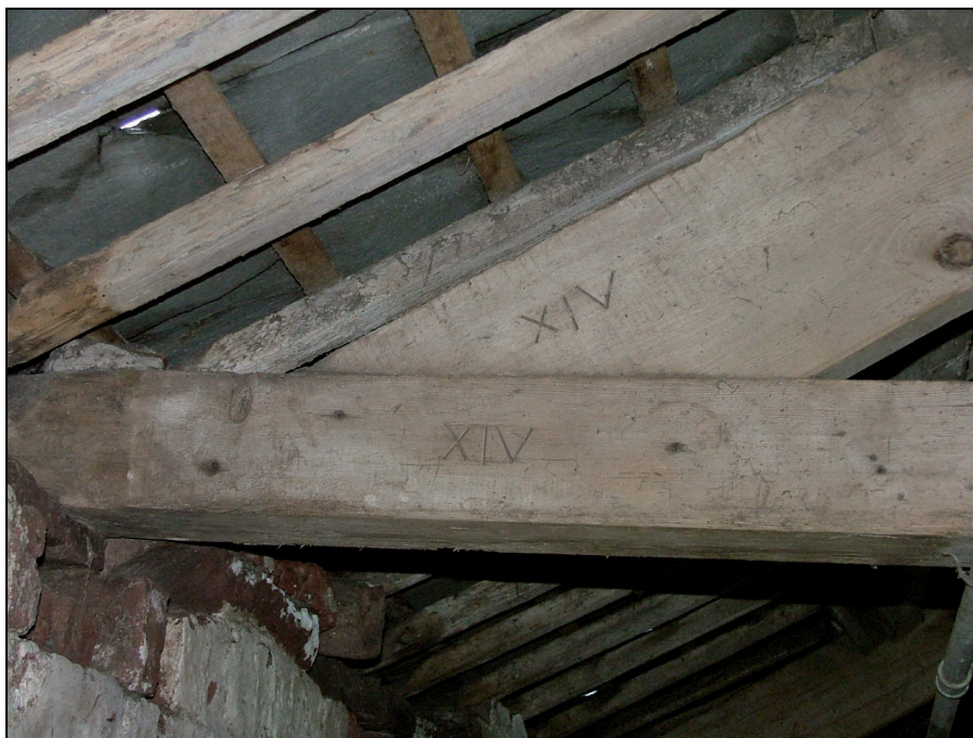
Plate 74: Assembly mark 'XIV' on the same truss as Plate 73, Building 5
