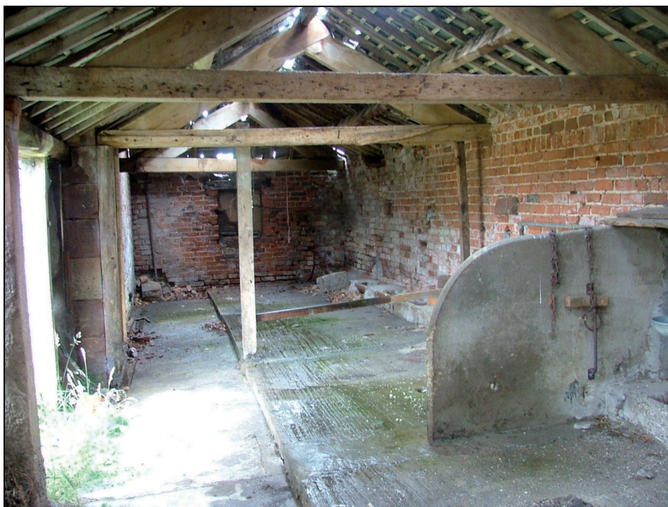
Plate 78: View looking west showing the interior of Building 6
