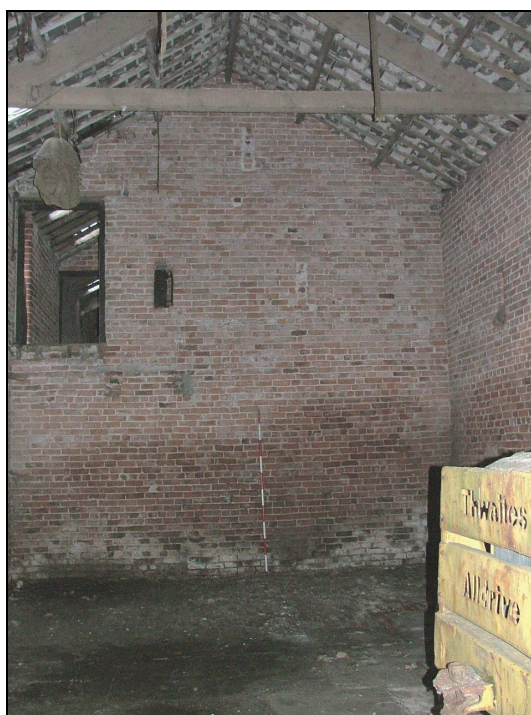
Plate 27: South internal gable of Building 1 (Scale = 2m)
