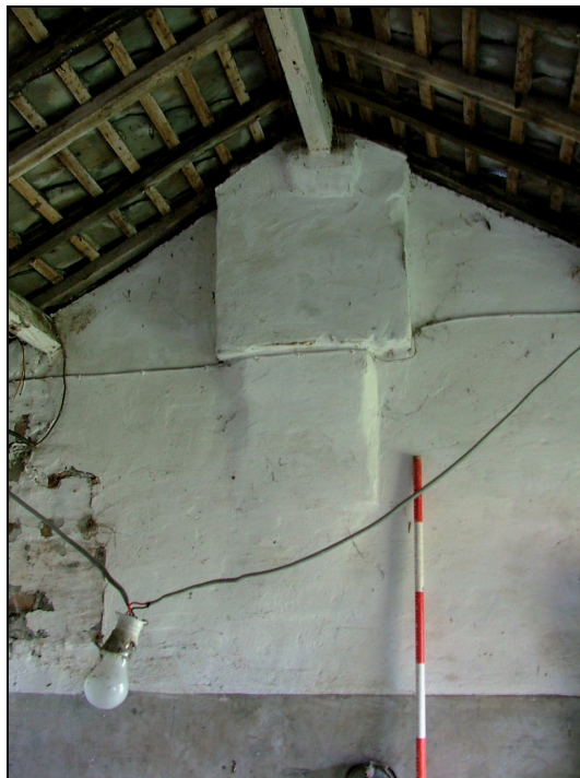
Plate 76: Possible remains of chimney stack, east room in Building 6
