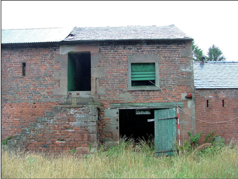
Plate 38: South end of the west elevation of Building 3 (Scale = 2m)
