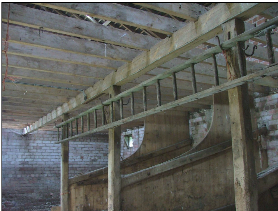
Plate 32: Iron hooks at the end of each stall, stable, Building 2
