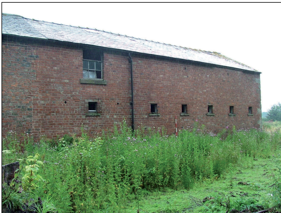
Plate 18: West elevation of Building 2
