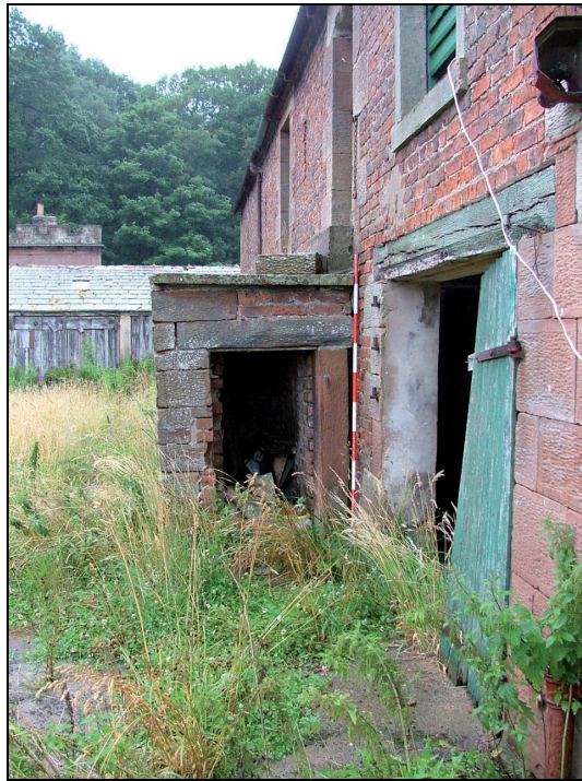
Plate 39: Void beneath the stone staircase, west elevation of Building 3 (Scale = 2m)
