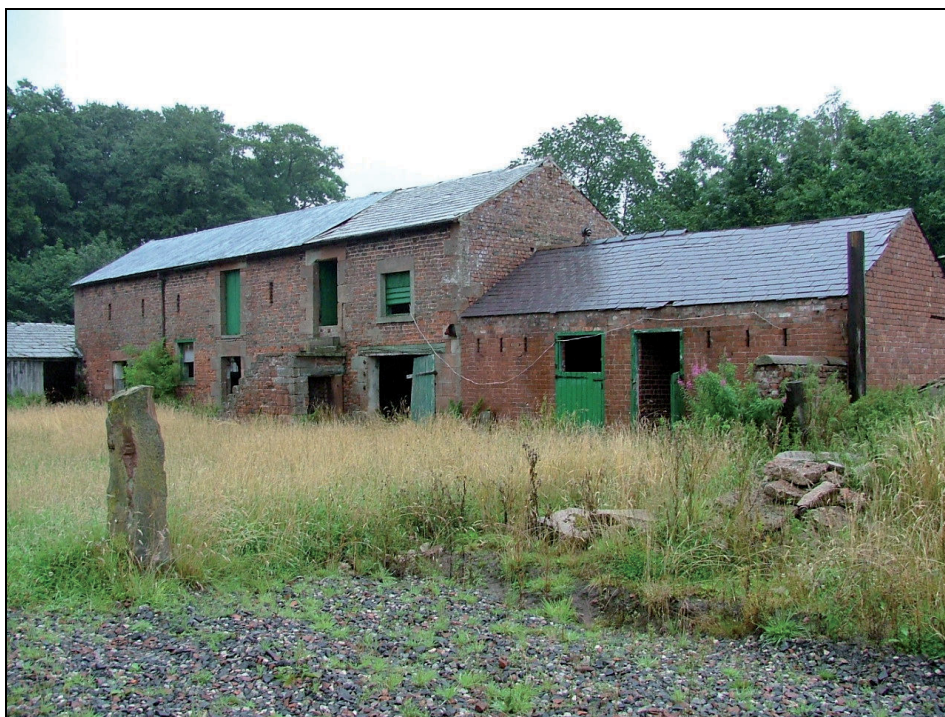
Plate 36: View looking north-east showing Range B, Buildings 3 and 4
