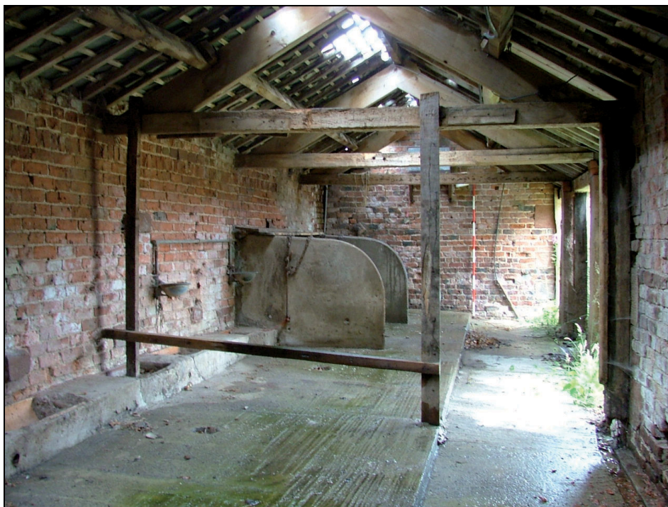
Plate 77: View looking east of the interior of Building 6 (Scale = 2m)
