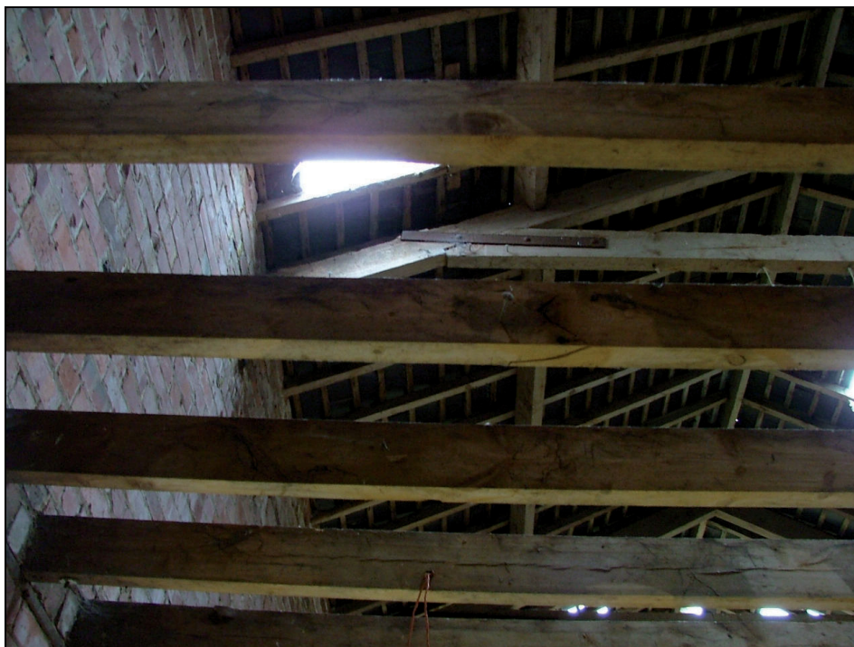
Plate 35: One of the two trusses over the hayloft, Building 2
