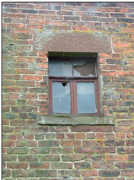
Plate 5: First floor window in east elevation of Building 1
