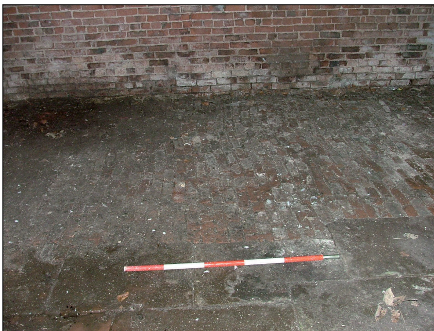
Plate 25: Detail of brick section of barn floor, Building 1
