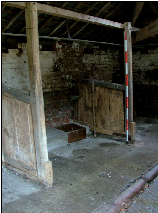
Plate 72: Detail of one of the stalls in Building 5 (Scale = 2m)
