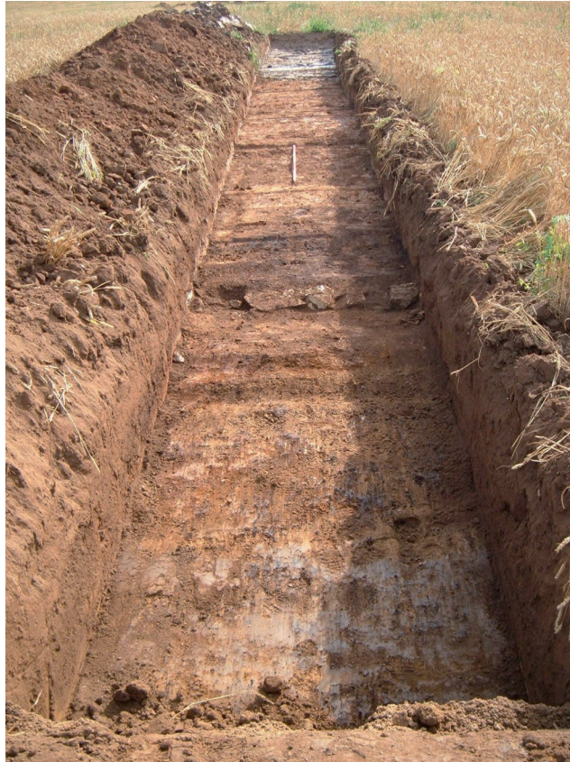
Plate 7: East facing overview of Trench 12 showing stone-lined drain in foreground.
