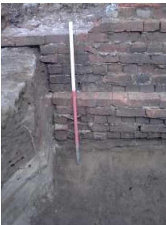
Plate 2: Detail of Foundation 1059, showing stepped brickwork. Facing North.
