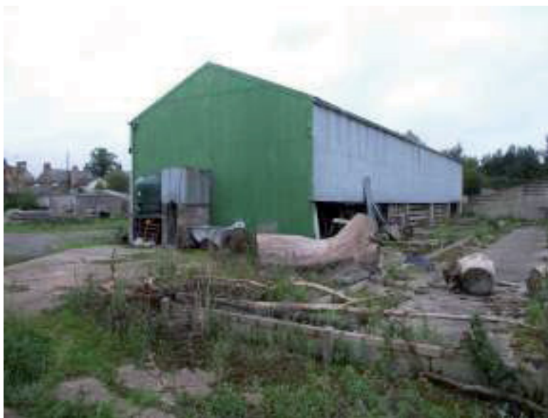
Plate 7: One of the standing buildings present on site, also shown on the left-hand side of Plate 6, looking south, southeast
