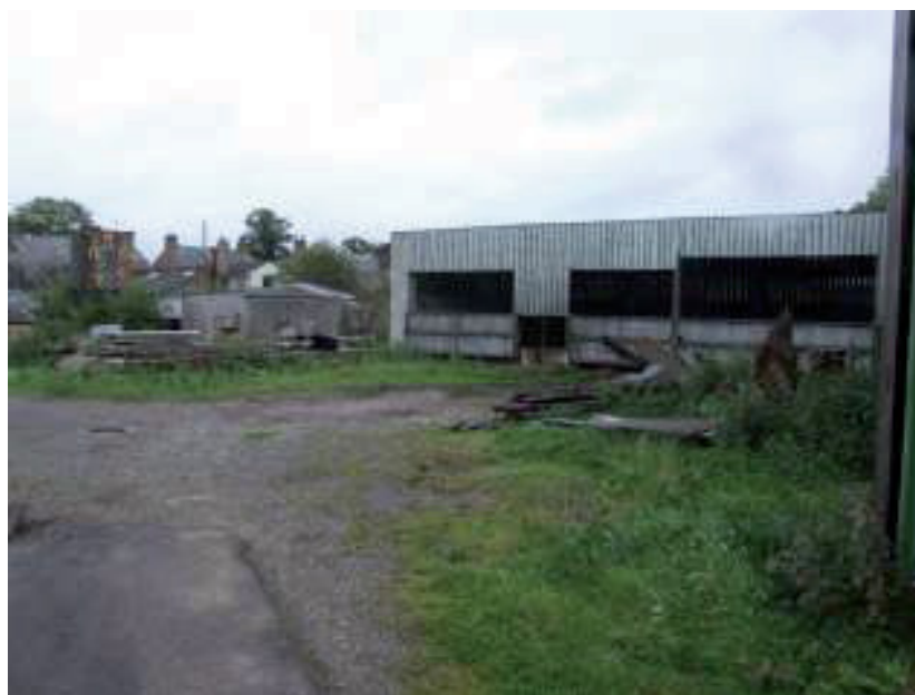
Plate 8: Two additional standing buildings present on site, looking east, northeast
