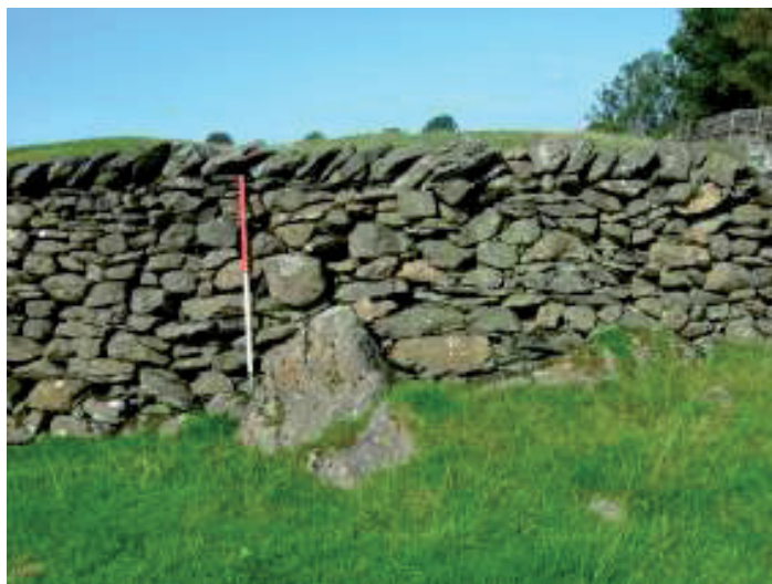
Plate 6: Limestone Drystone Wall using natural rocky terrain in Field 1, see (Plate 3)
