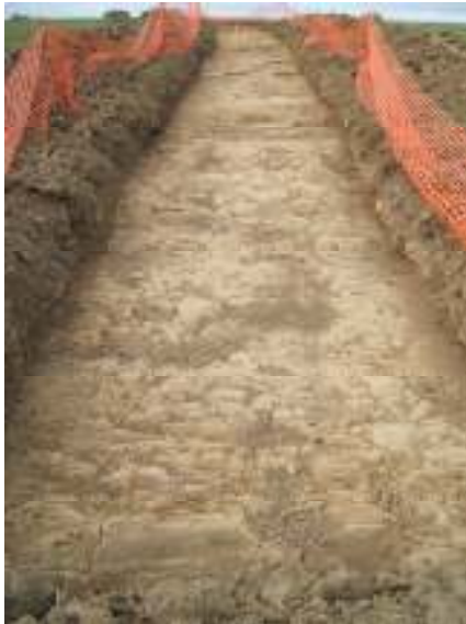
Plate 15: Trench 13 looking west-northwest
