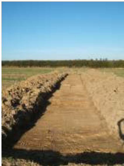
Plate 11: Trench 9 looking west
