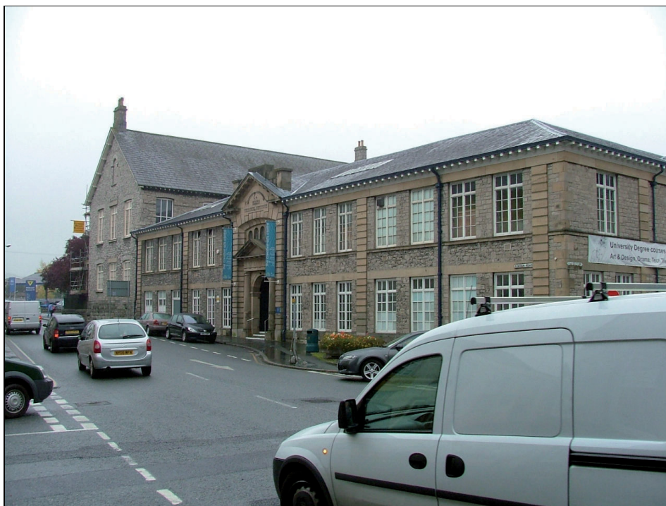
Plate 6: View looking north-east showing the Kendal College building with part of Kendal Museum in the background, Station Road
