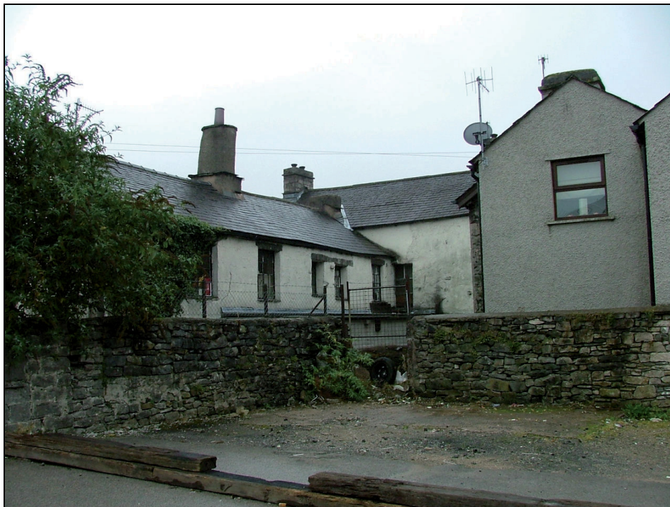
Plate 11: View looking east showing possible surviving cottages of a former long row of dwellings to the rear of Wildman Street
