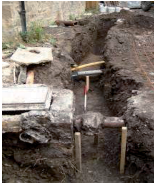
Plate 1: Trench 1 showing services, looking north.
