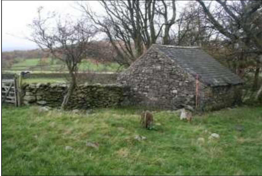
Plate 2: Foundations of a possible ruined building and existing shed on the west side of the site, looking northwest
