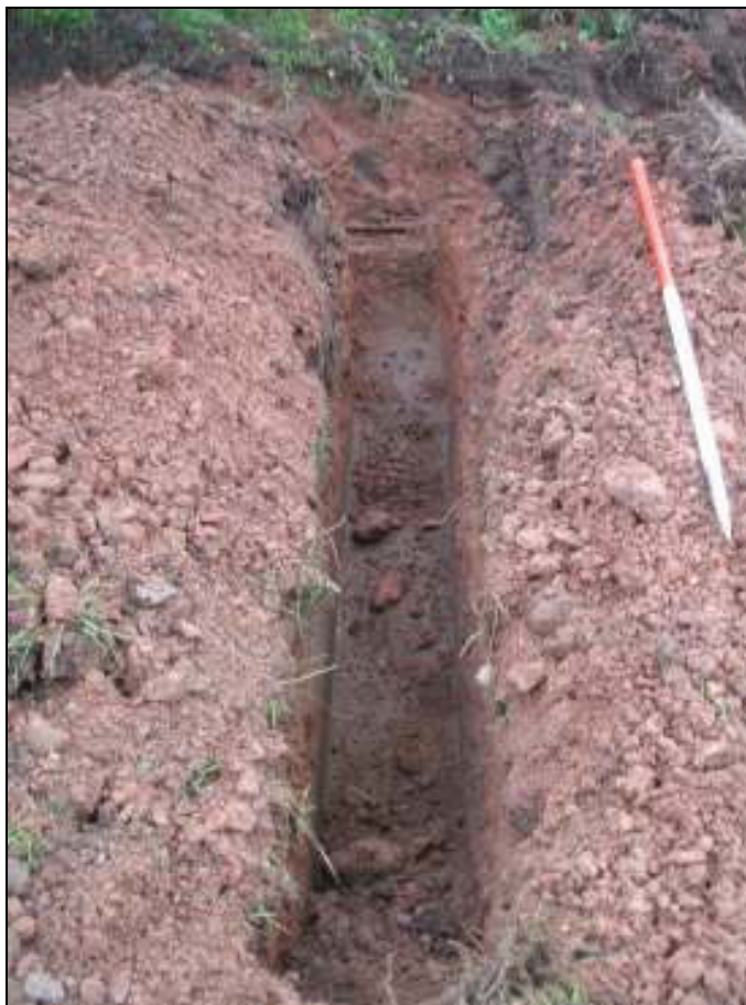
Plate 6: View north of additional section of service trench within field
