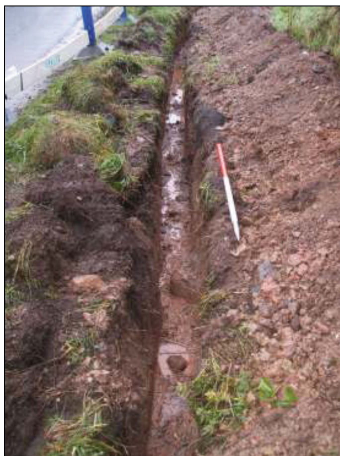
Plate 1: View north-northwest of service trench through grass verge
