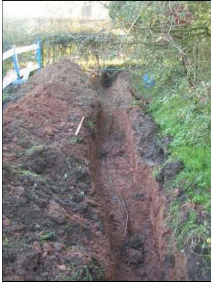
Plate 4: View east of service trench within field
