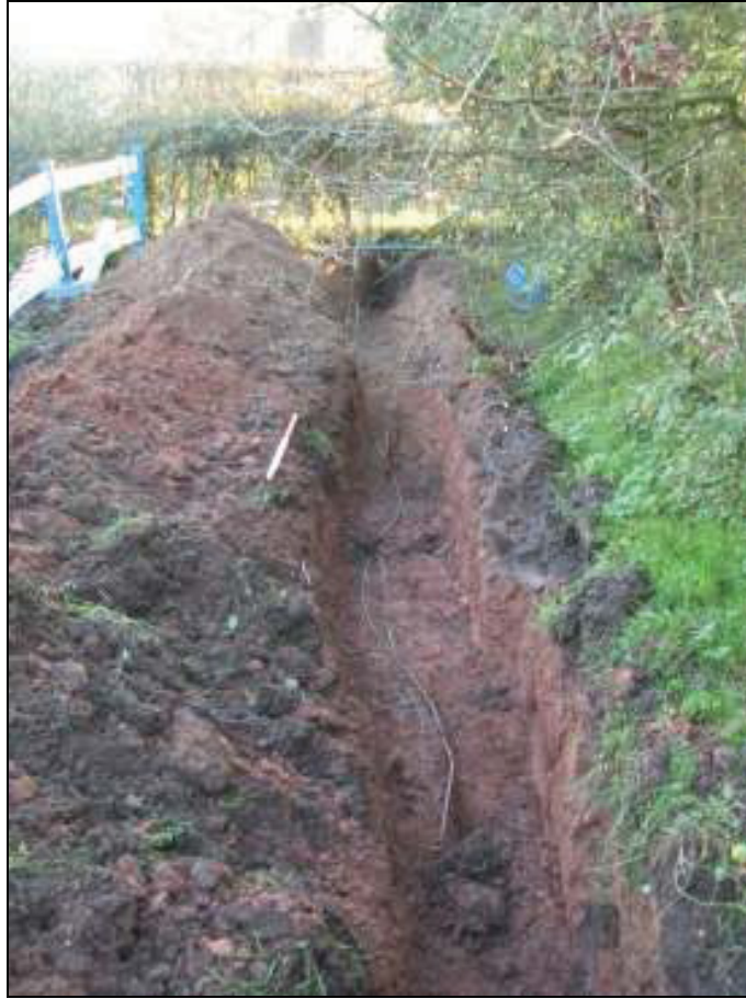
Plate 4: View east of service trench within field
