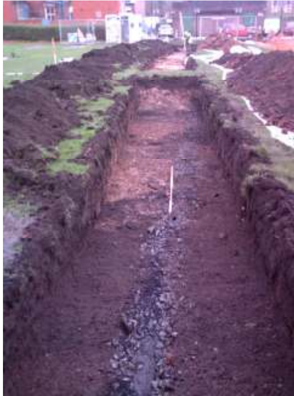
Plate 9: West facing overview of Trench 7
