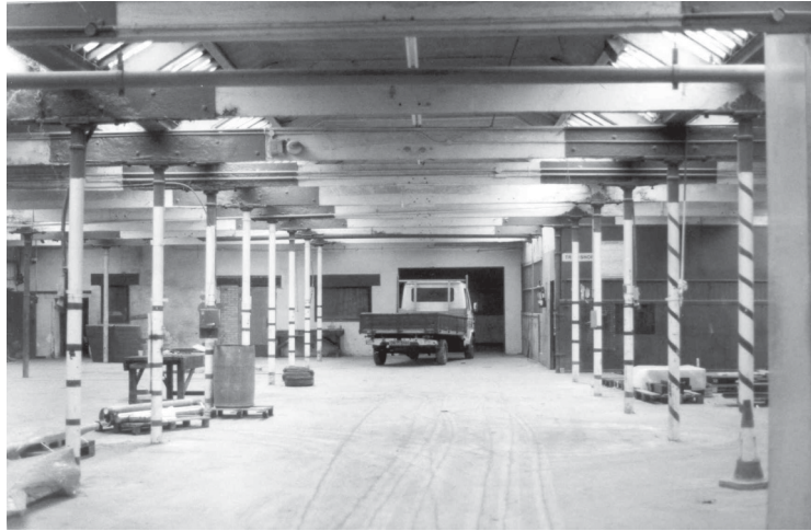
Plate 2: Interior of former weaving or power loom shed.
