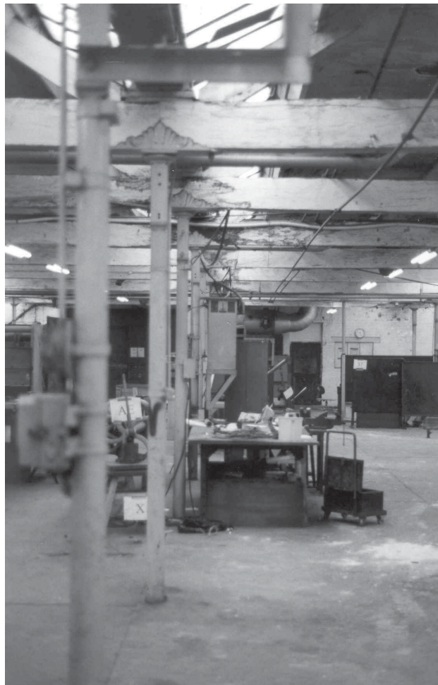
Plate 1: Interior of former power-loom shed.
