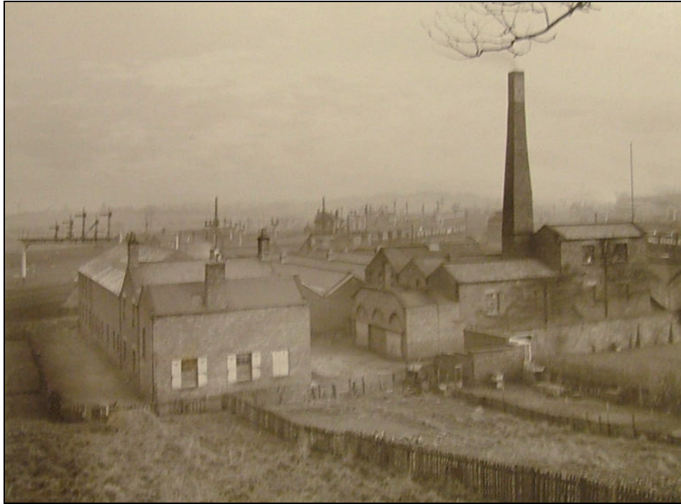
Figure 6 – Photograph of c.1907 showing the works as seen from the west
