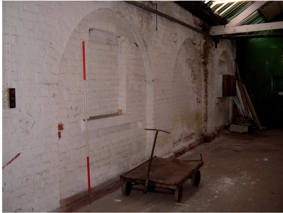
Plate 5: Evidence of at least two phases of use. East elevation of former two-storey building.
