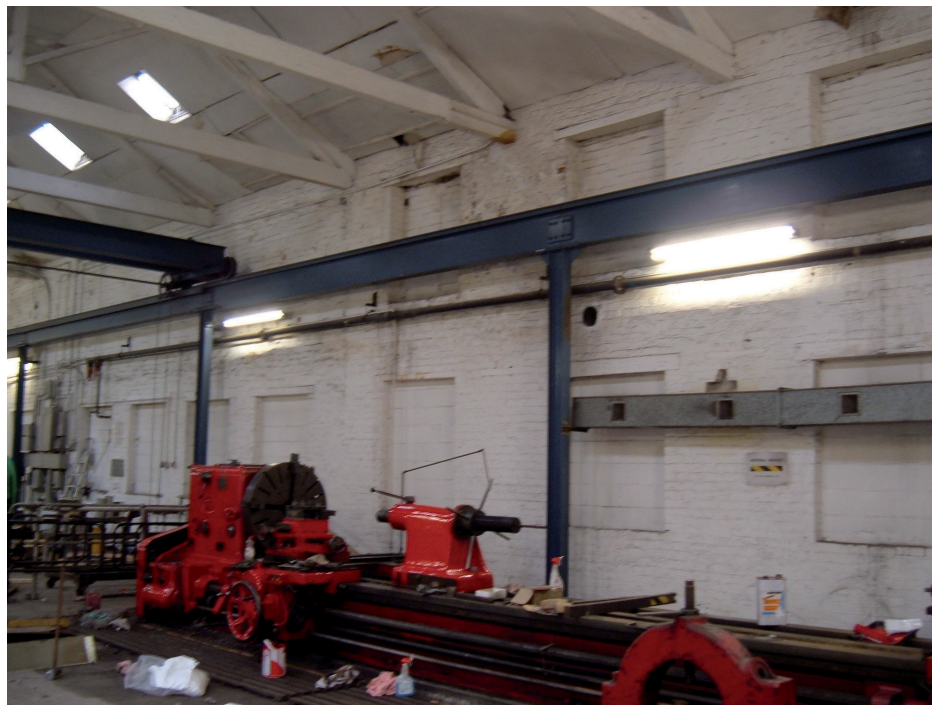
Plate 6: Former two-storey building shown on figures 5b and 6.
