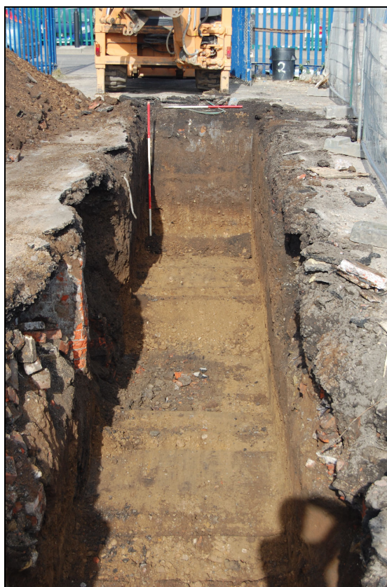
Plate 1: View north of Trench 1
