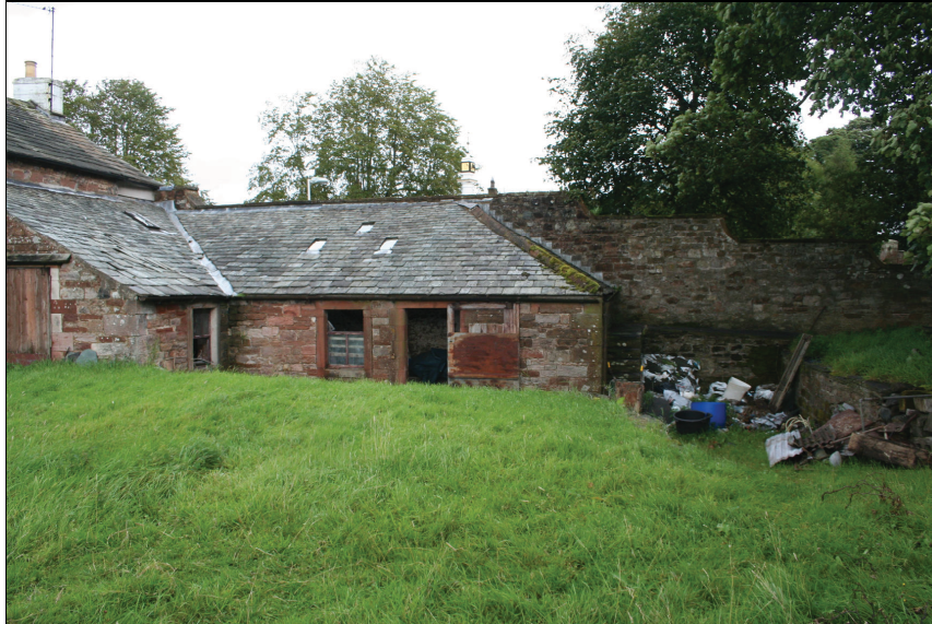
Plate 5: The site prior to excavation, showing the 19 th century lean-to building and sunken yard (looking east).
