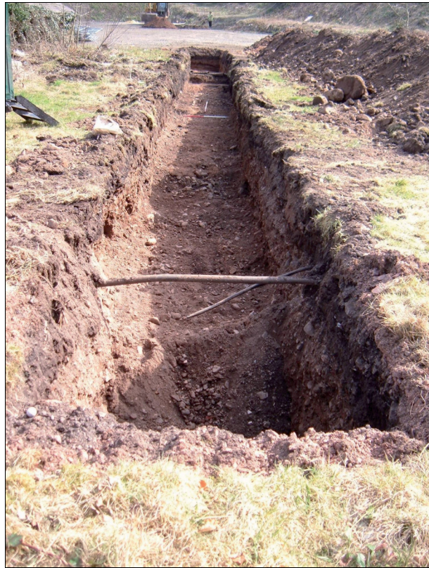
Plate 1: View southeast of Trench 1
